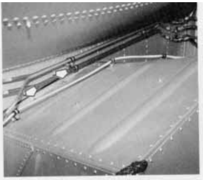
Two of the five rigid fasteners that can be replaced with NAS 1298 shoulders screws and spring washers are visible in this photograph.
