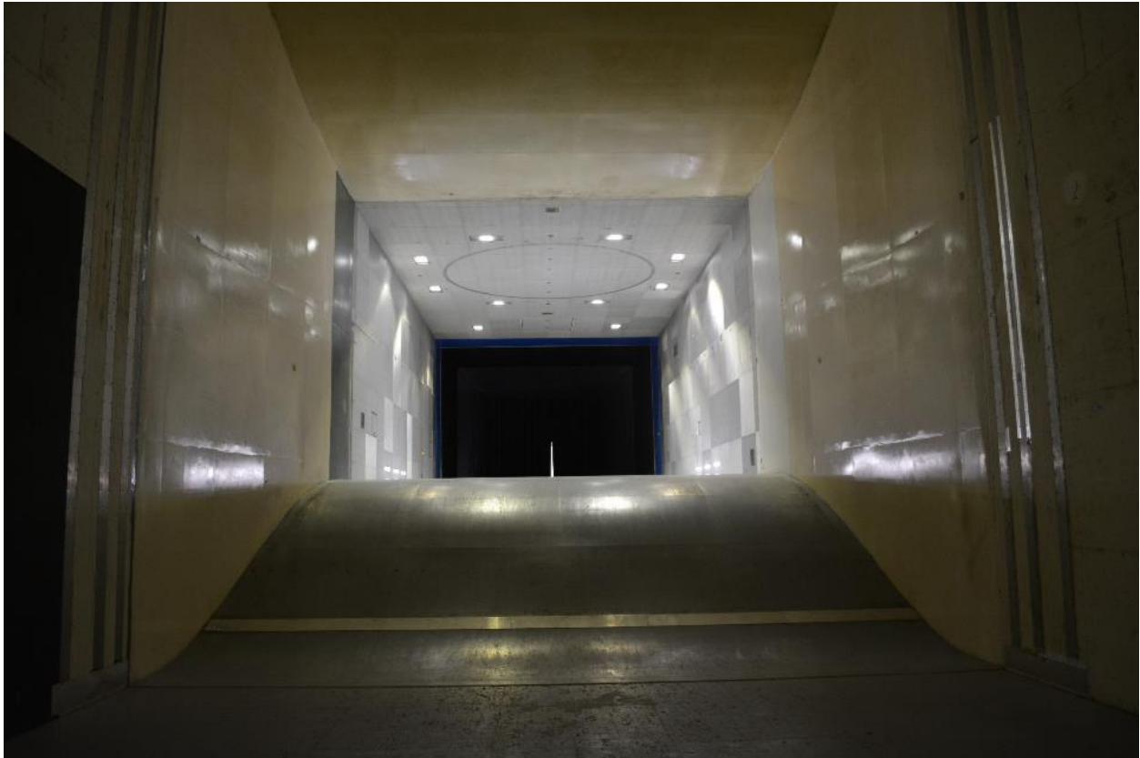
Figure 5. View Looking Downstream Through Both Test Sections.
