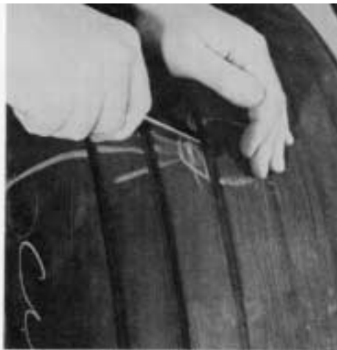
Probe foreign object damage with blunt awl: shield work. Photo courtesy of S. F. Goodrich Co.
