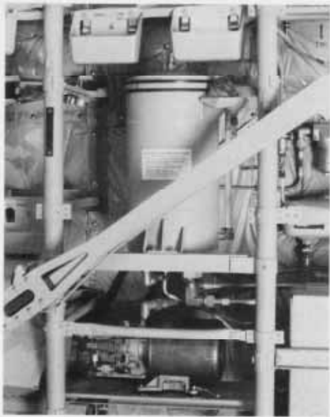
Auxiliary hydraulic system reservoir and pump.
