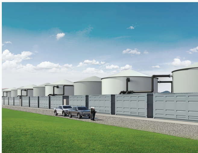
RENDERING: 10 MWAC, 100 MWh GridStar Flow installation consisting of five 2 MWAC ESUs coupled together
