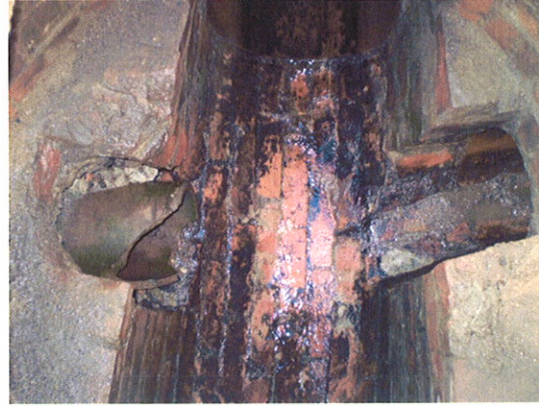
Manhole PAE-1 After Debris Removal
