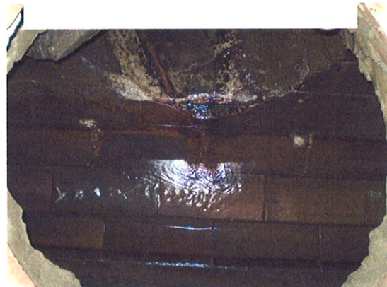
Manhole MH-1 After Debris Removal
