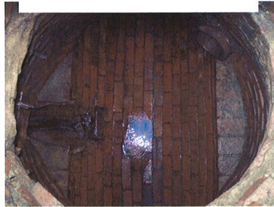
Manhole PAW-6 After Debris Removal
