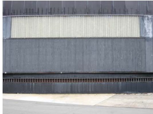
Typical Airdock door siding
