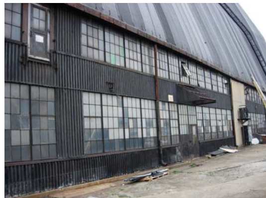
Typical Airdock vertical siding
