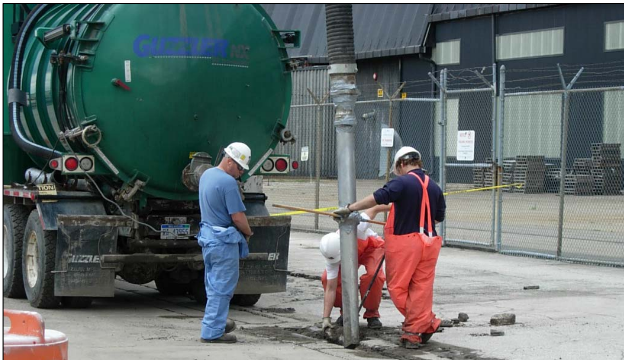
Photo 3 – Hand lance vacuum process removal
