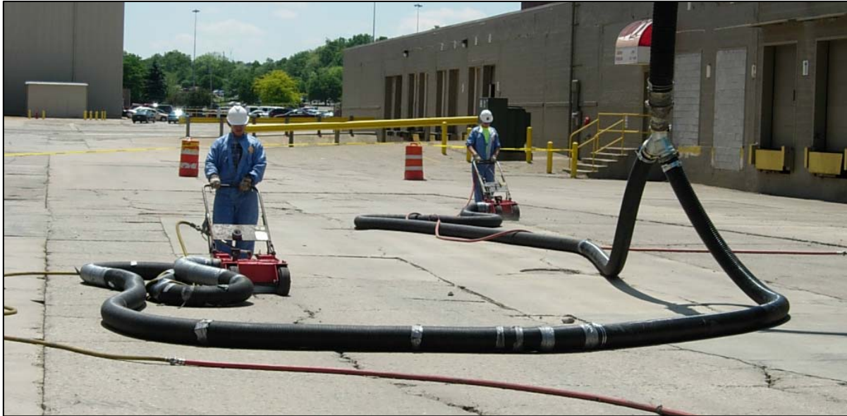
Photo 1 – Debris removal with shrouded mobile chambers
