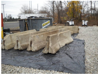
4. Concrete barriers lined up and ready for removal from site.
