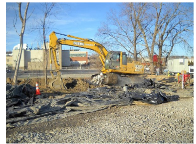
3. Cleaning of excavator tracks prior to removal of equipment from site.
