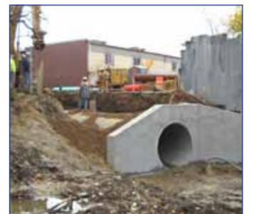
TAKEN from the southern end of the Haley's Ditch project and looking south, this photo shows the City of Akron's work to replace the 66-inch diameter storm drain pipe, which runs from Triplett Boulevard to the outfall of Haley's Ditch.
