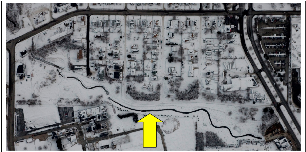
This is an aerial view of the Haley's Ditch project site taken in December 2009.
