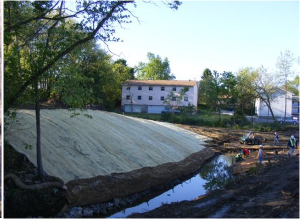
East bank of the trail has been restored
