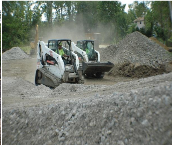
Materials for the restoration are stockpiled
