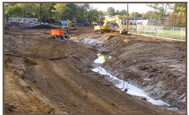
Forming new channel in the middle zone
