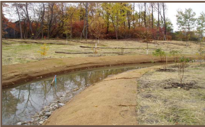
Stream bank protection and planting in the South Zone
