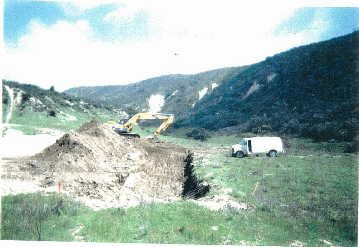
Figure 2-11. Excavated Disposal Trench
