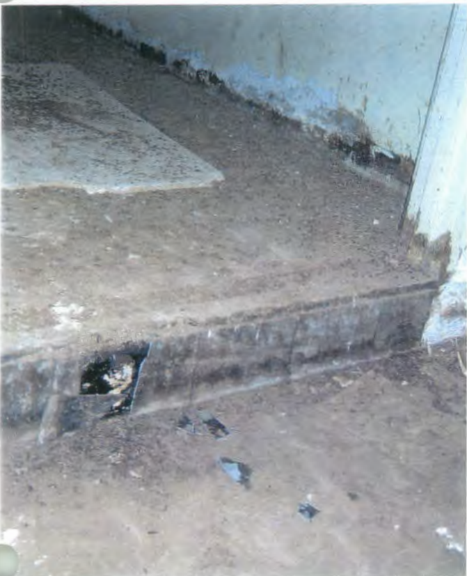
Site 1, Bldg. 305, Asbestos Containing Vinyl Floor Tile & Mastic & Base of Step
