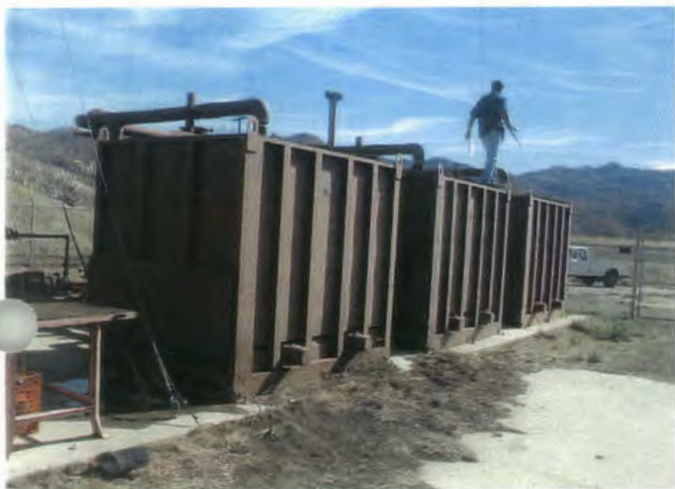
Site 1, Lead Paint on all Metal Components
