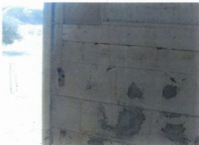
Site 1, Bldg. T4, Lead Paint on Exterior Walls
