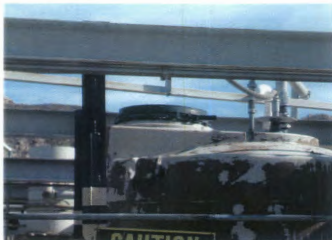
Site 1, Lead Paint on all Steel/Metal Components
