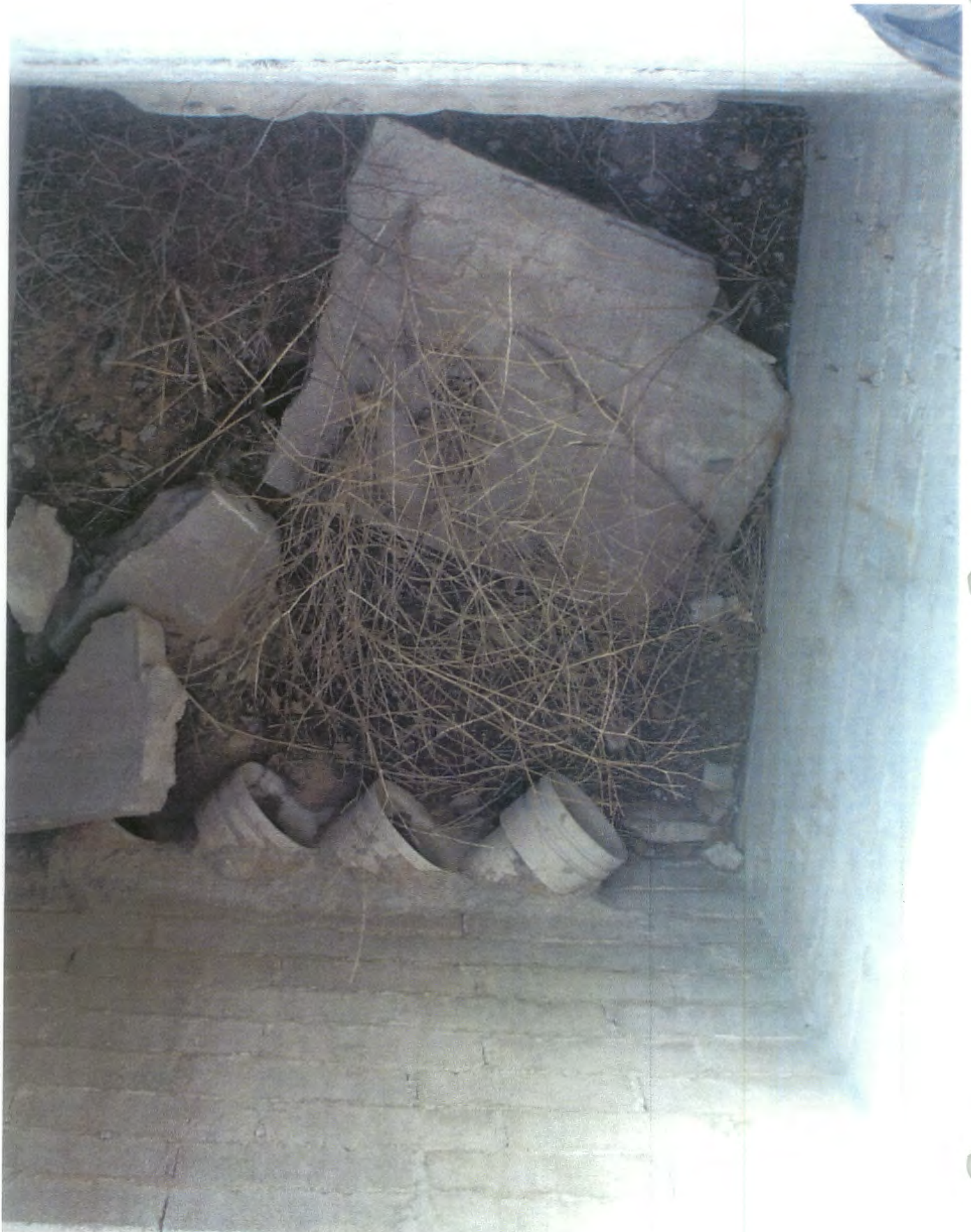
Site 1, Bldg 305, Asbestos Transit Pipes Extending Below Grade
