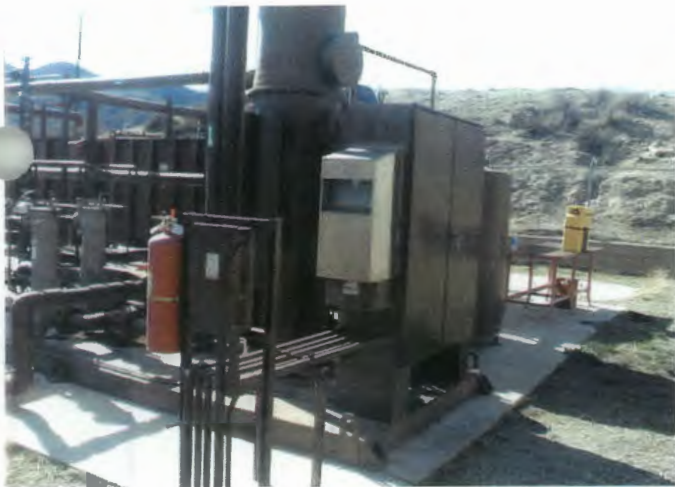
Site 1, Lead Paint on all Metal Components
