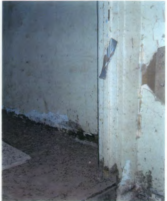
Site 1, Bldg. 305, Asbestos Containing Drywall Joint Compound
