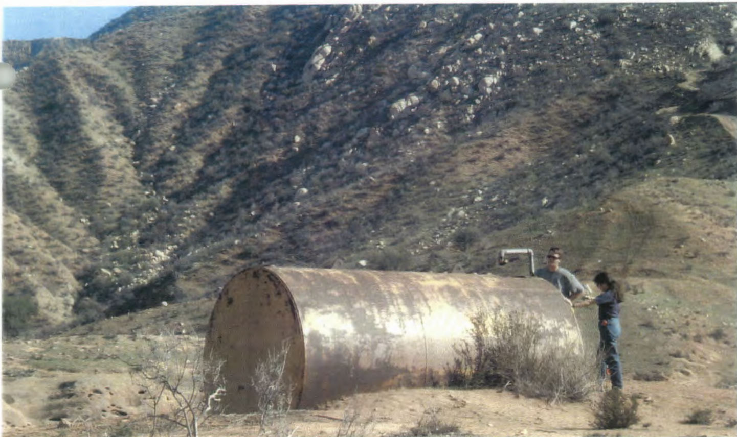
Site 1, Lead Paint on Steel/Metal Components
