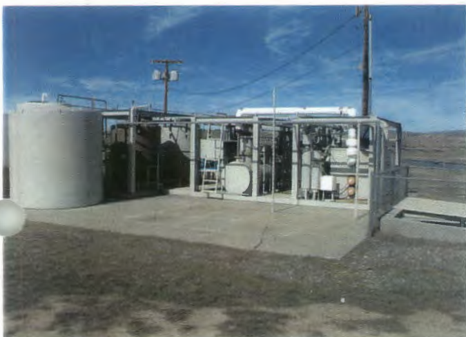
Site 1, Lead Paint on all Steel/Metal Components
