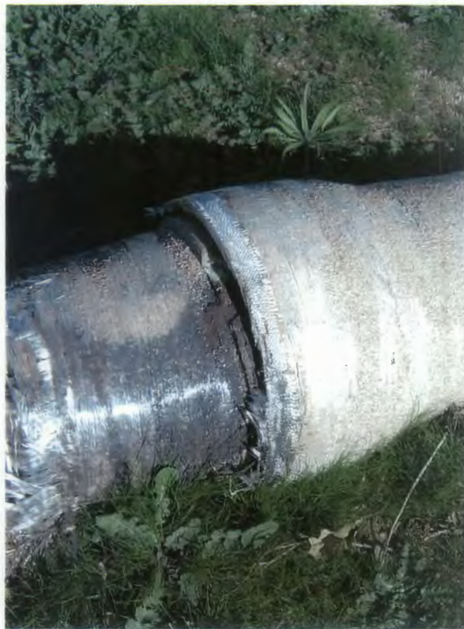
Site 1, Bldg. 305, Non-Asbestos Containing Pipe Insulation Layers
