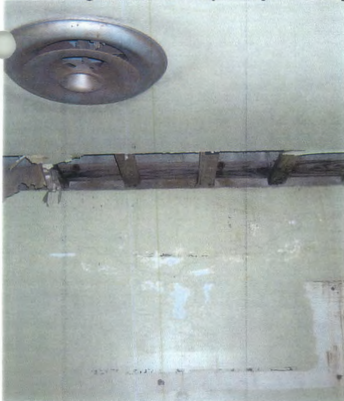
Site 1, Bldg. 303, damaged asbestos containing drywall joint compound
