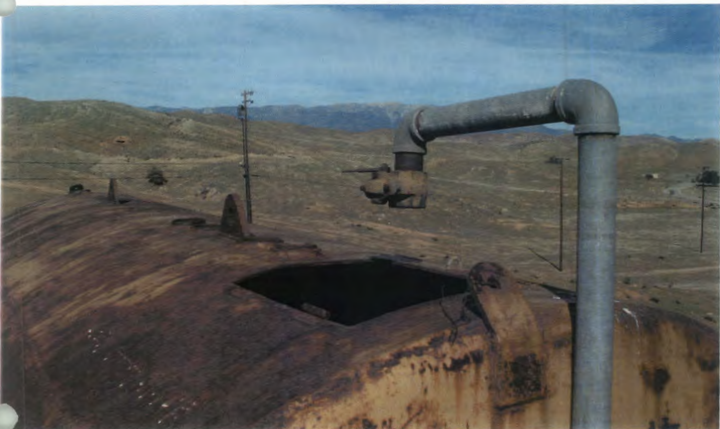
Site 1, Lead Paint on Steel/Metal Components
