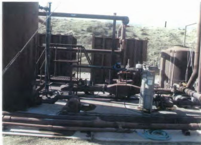
Site 1, Lead Paint on all Metal Components
