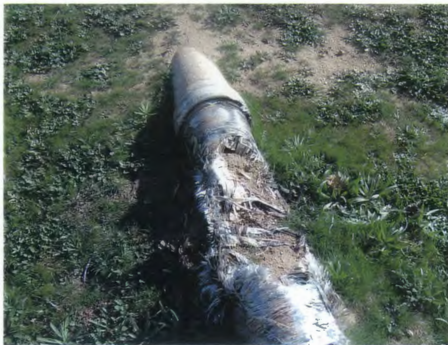
Site 1, Bldg. 305, Non-Asbestos Pipe Insulation Layers
