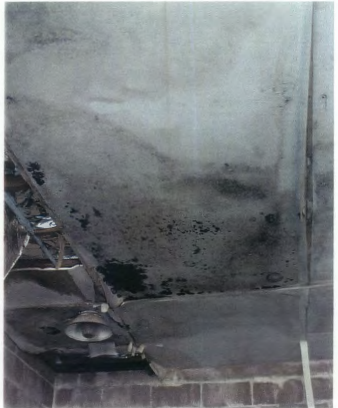
Site 1, Bldg. 312, Mold Growth on Ceiling Components
