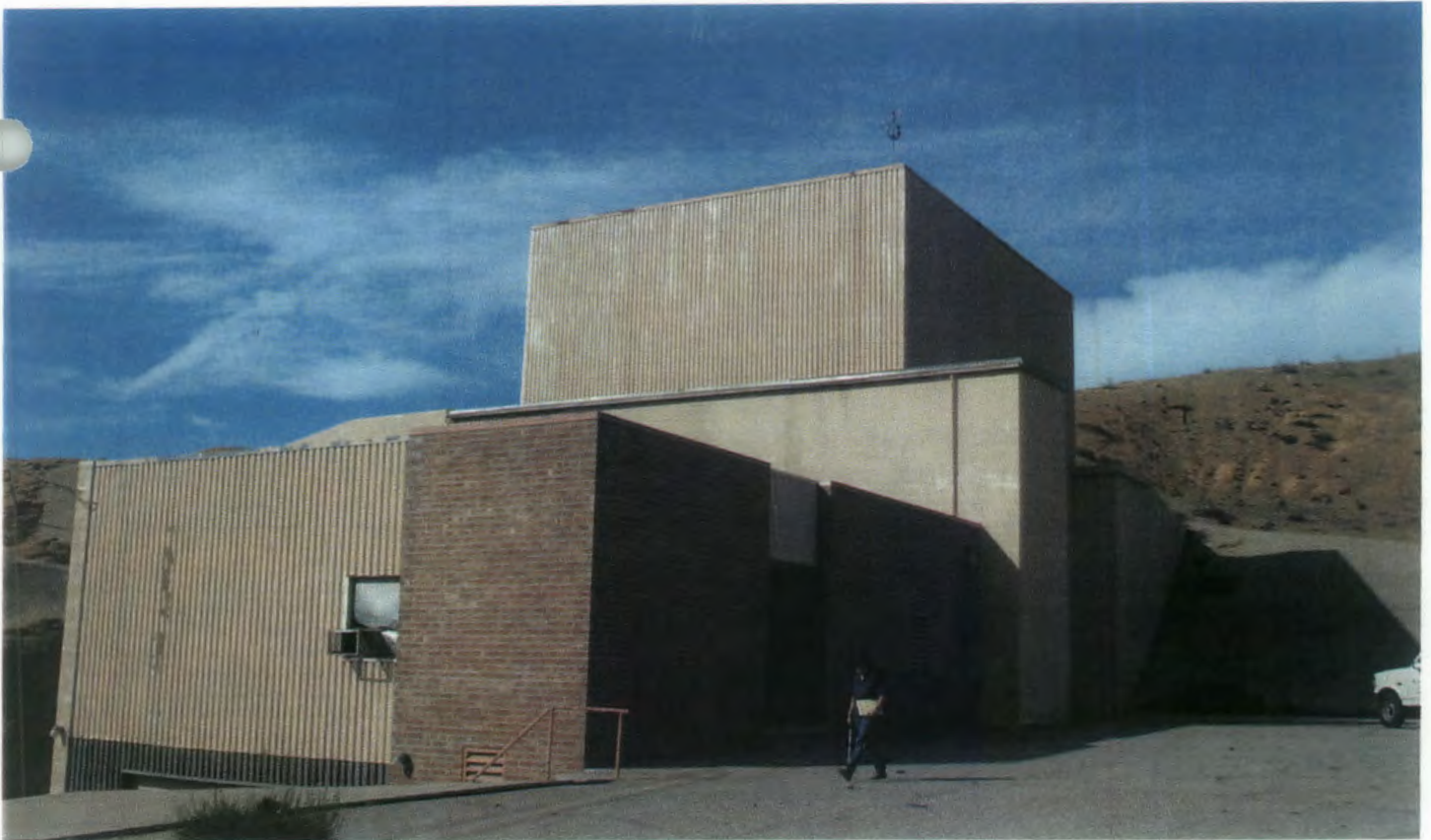
Site 1, Bldg. 303, Exterior Lead Paint on Steel/Concrete Walls; Asbestos Containing Red Brick Grout/Mortar & Asbestos Containing Wall Putty/Caulking
