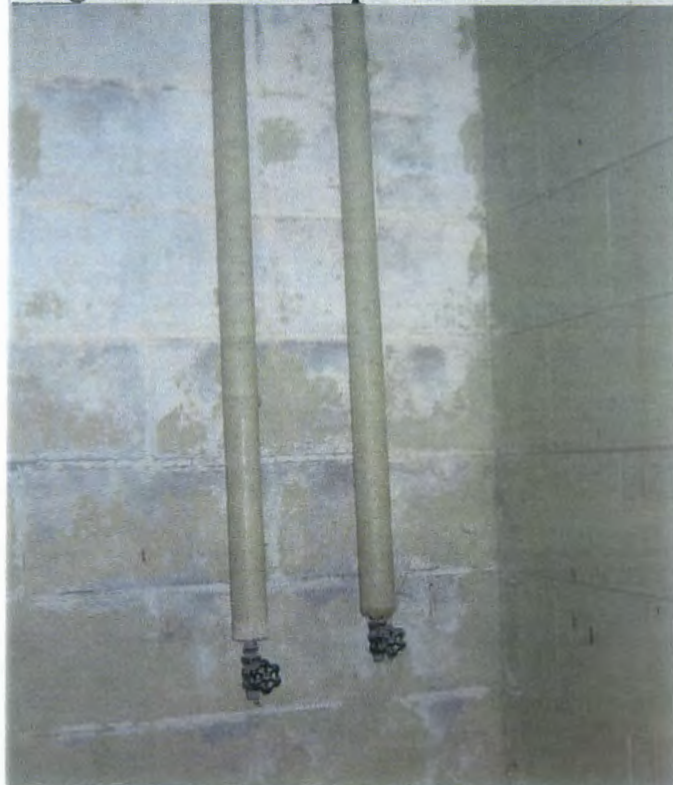
Site 1, Bldg. 303, Asbestos Containing Pipe Elbow Insulation
