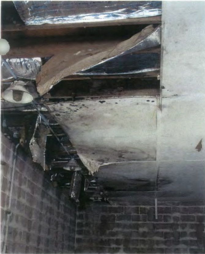
Site 1, Bldg. 312, Mold Growth on Ceiling Components
