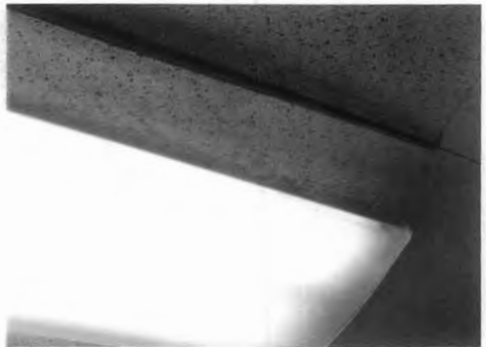
Site 1, Bldg. 315, Mold Growth on Interior Ceiling Components
