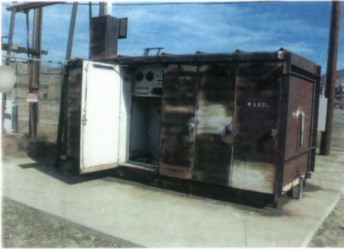
Site 1, Lead Paint on all Metal Components
