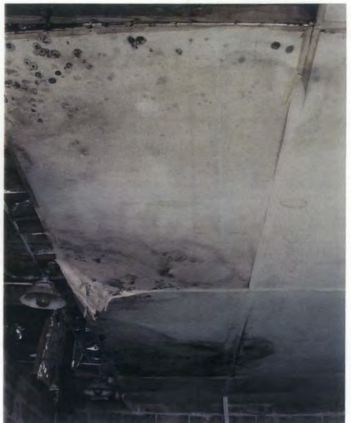
Site 1, Bldg. 312, Mold Growth on Ceiling Components
