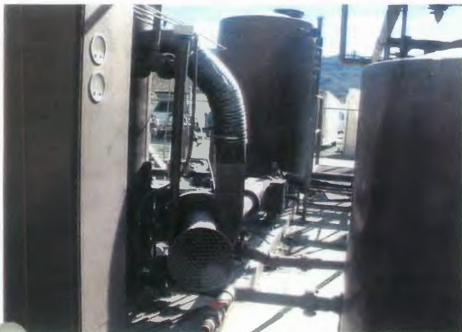
Site 1, Lead Paint on all Metal Components
