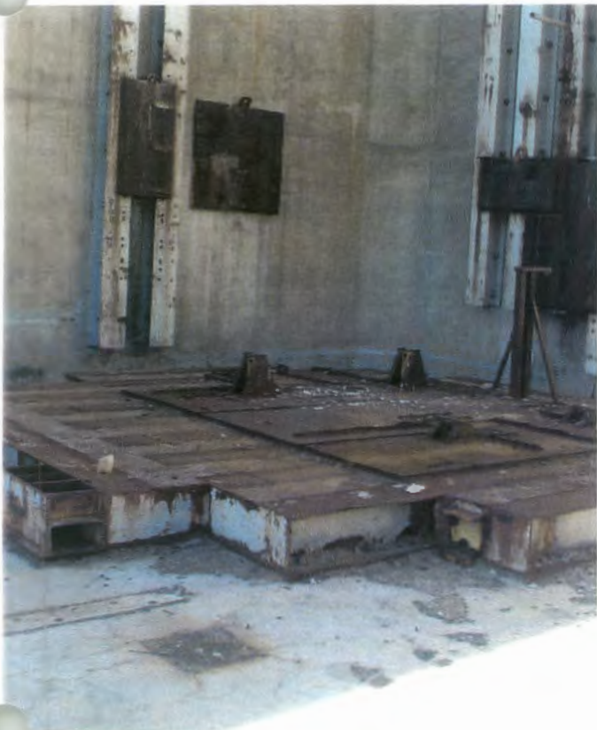
Site 1, Bldg. 308, Lead Paint on Walls & Steel Components
