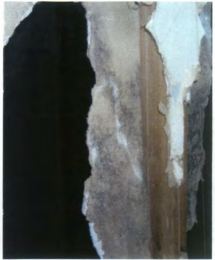
Site 1, Bldg 305, Asbestos Containing Drywall Joint Compound & Mold Growth
