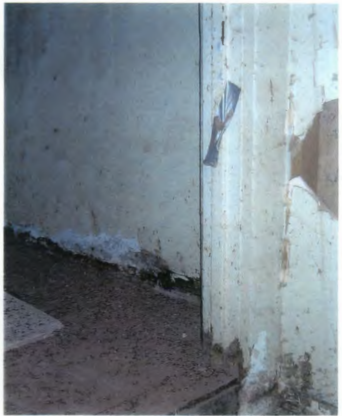
Site 1, Bldg. 305, Asbestos Containing Drywall Joint Compound
