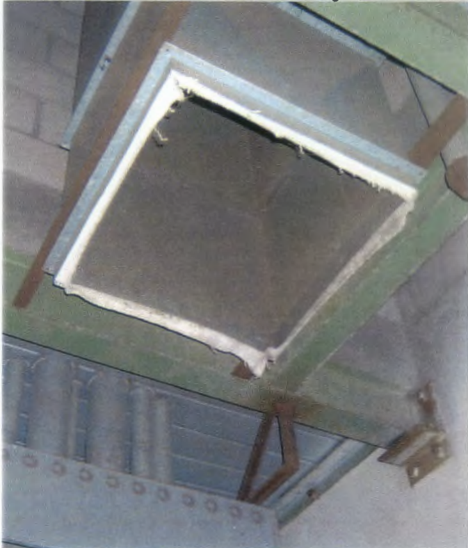
Site 1, Bldg. 303, Asbestos Containing HVAC Vibration Damper Cloth
