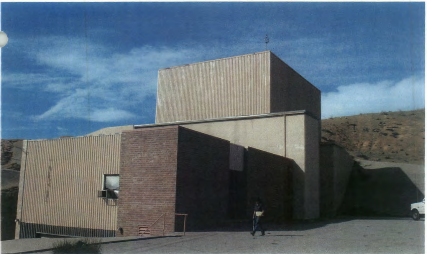
Site 1, Bldg. 303, Exterior Lead Paint on Steel/Concrete Walls; Asbestos Containing Red Brick Grout/Mortar & Asbestos Containing Wall Putty/Caulking
