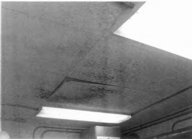
Site 1, Bldg. 315, Mold Growth on Interior Ceiling Components
