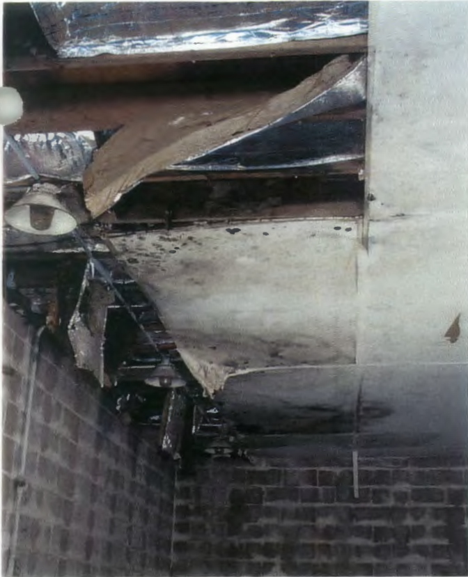
Site 1, Bldg. 312, Mold Growth on Ceiling Components
