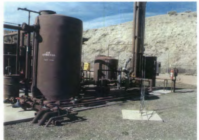
Site 1, Lead Paint on all Metal Components
