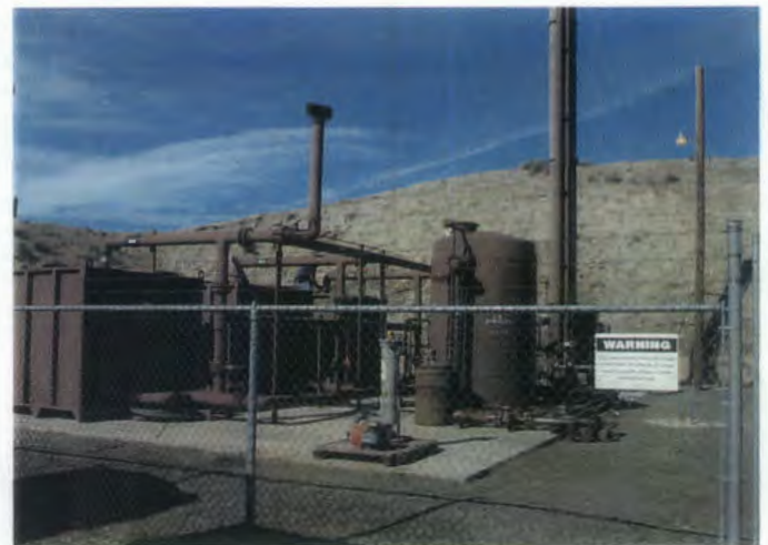
Site 1, Lead Paint on all Metal Components
