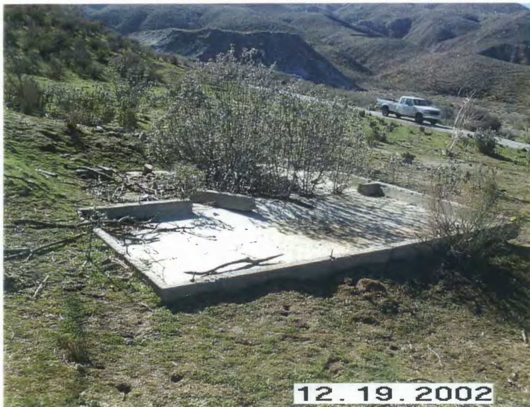
Photograph 19. Typical Pad with Protruding Bolts (Old Structure)
