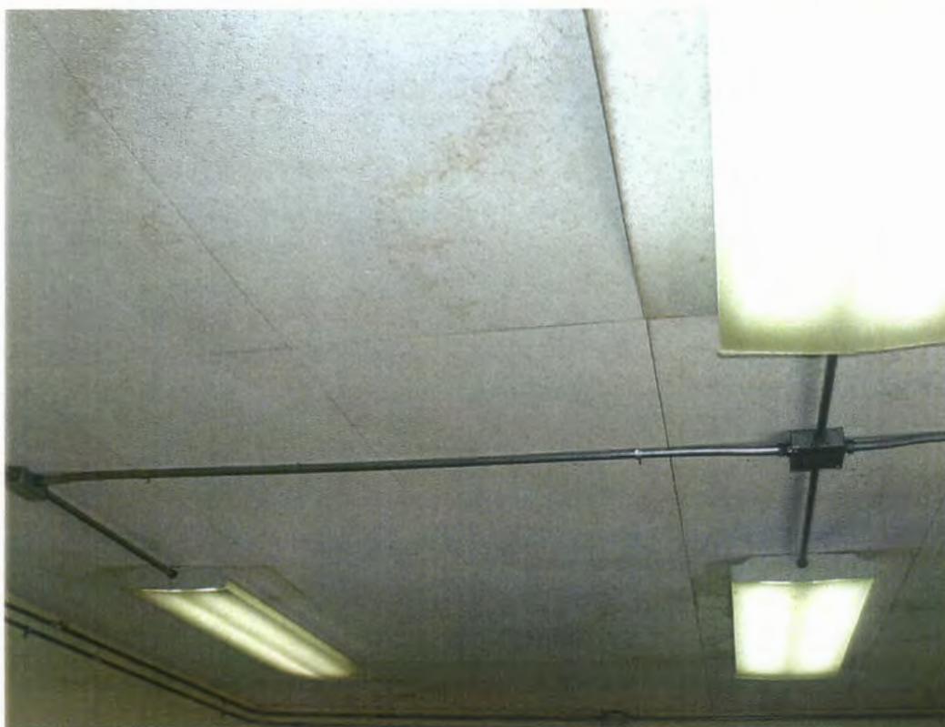
Photograph 4. Fluorescent Light Fixtures (Toxics)
