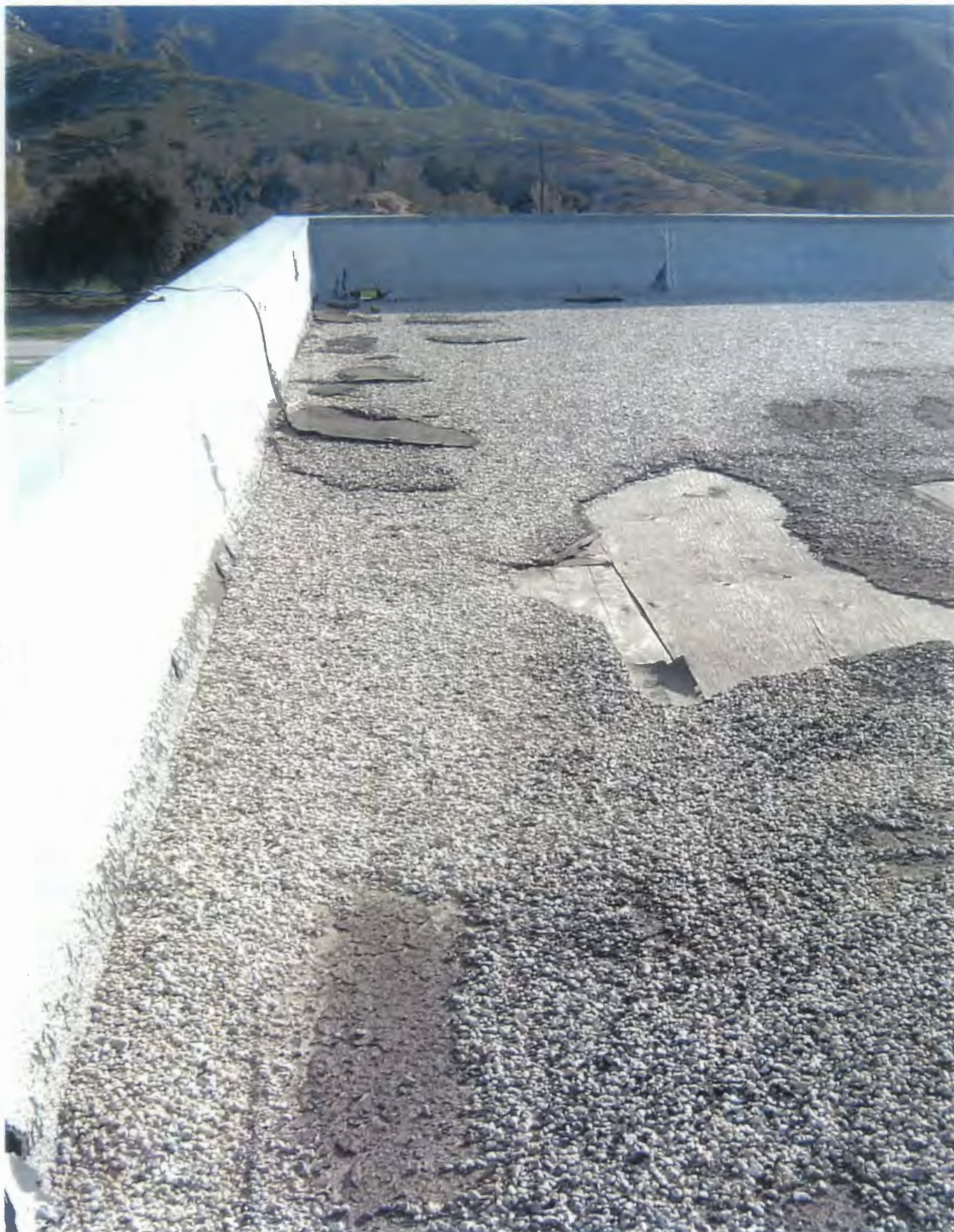
Site 1, Bldg. 312, Asbestos Containing Gray Roof Patch/Penetration Mastics
