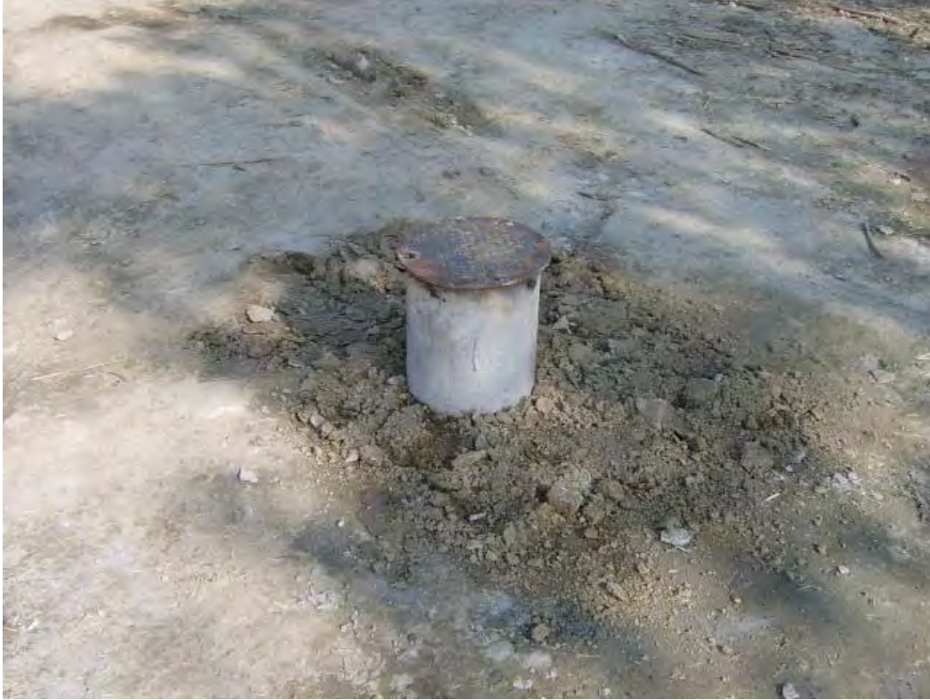
Photo 3: Well W-1-1 after abandonment completion
