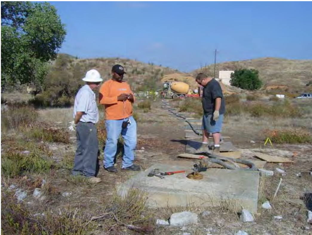
Photo 4: Well W-1-2 being abandoned by pressure grouting. Well is fitted with a pressure cap and grout is pumped under pressure into well casing and annular space.
