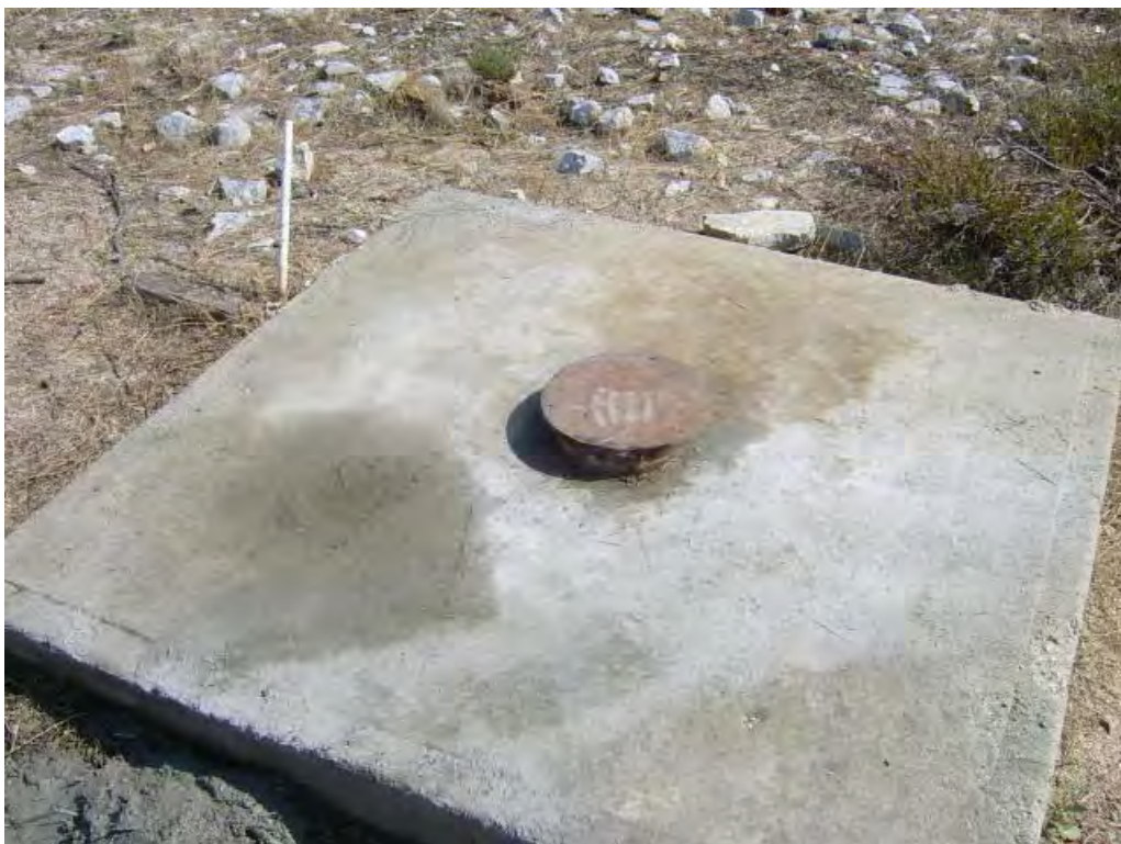
Photo 7: Well W-1-2 after completion of well abandonment.
