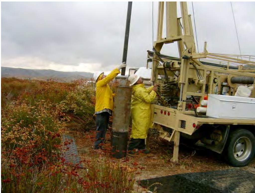
Photo 9: Preparation of Well W-1-5 for abandonment: Placement of tremmie pipe in well to pump in sealing grout.
