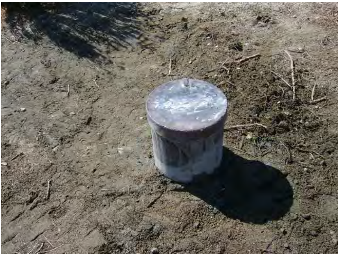
Photo 11: Well W-1-5 after completion of well abandonment.
