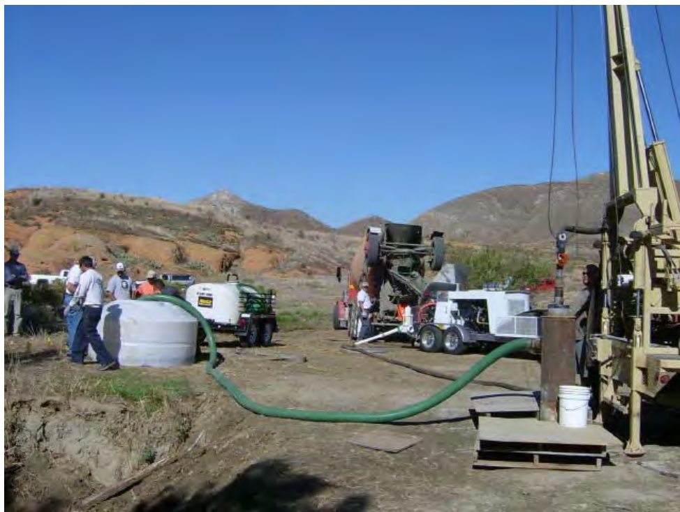
Photo 2: Well abandonment process at Well W-1-1
