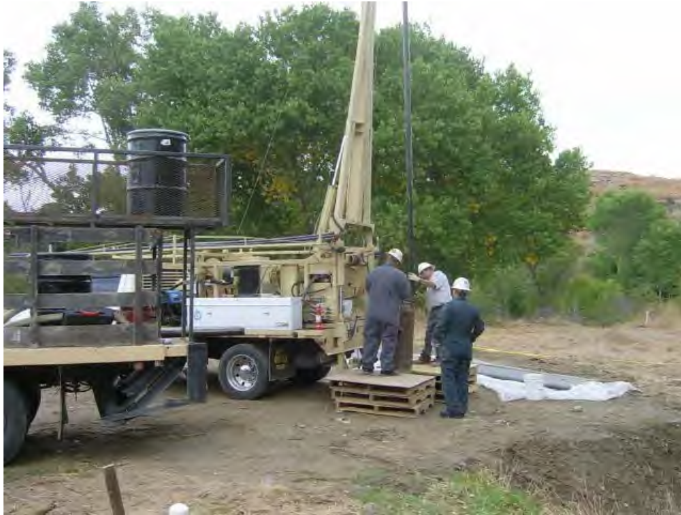
Photo 1: Preparing Well W-1-1 for abandonment. Pump and piping removed from well, casing extension to capture displaced water installed, and tremmie pipe lowered into well to pump in grout.
