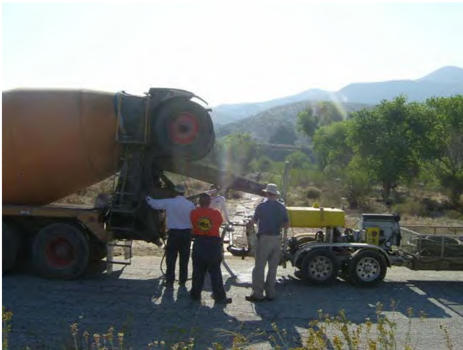
Photo 5: Well W-1-2 being abandoned by pressure grouting. Excessive SKR burrows and surrounding soil type prevented vehicular access to the well location to abandon using tremmie pipe.
