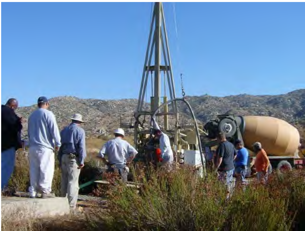
Photo 10: Well W-1-5 abandonment process proceeding.
