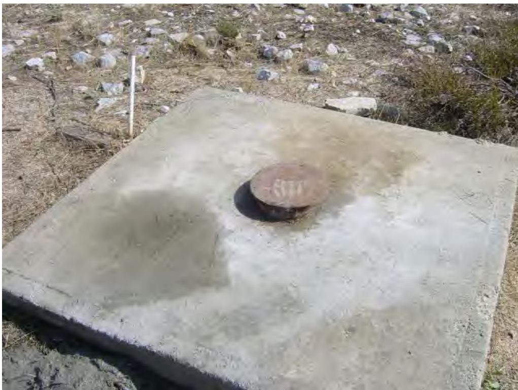
Photo 7: Well W-1-2 after completion of well abandonment.
