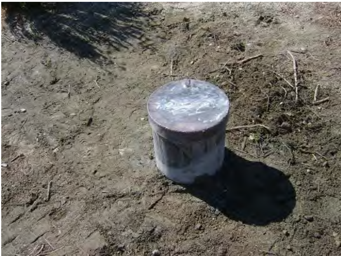
Photo 11: Well W-1-5 after completion of well abandonment.
