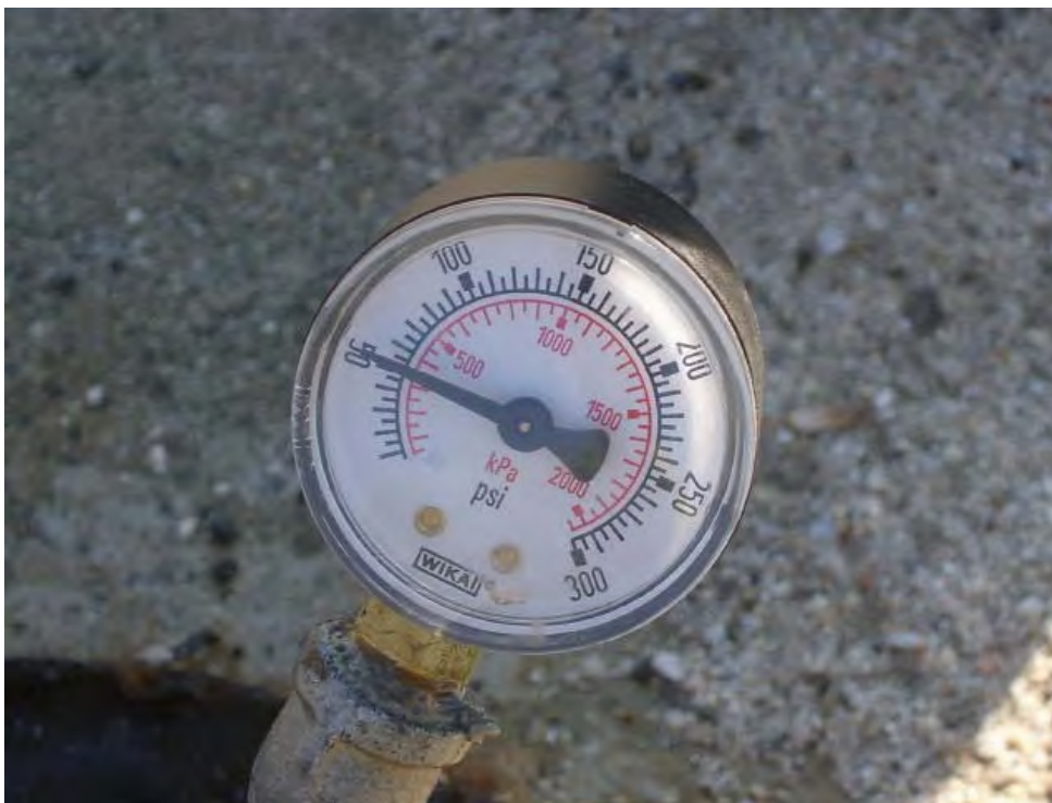
Photo 6: Grout pressure maintained after pumping Well W-1-2 casing and annular space full of grout
