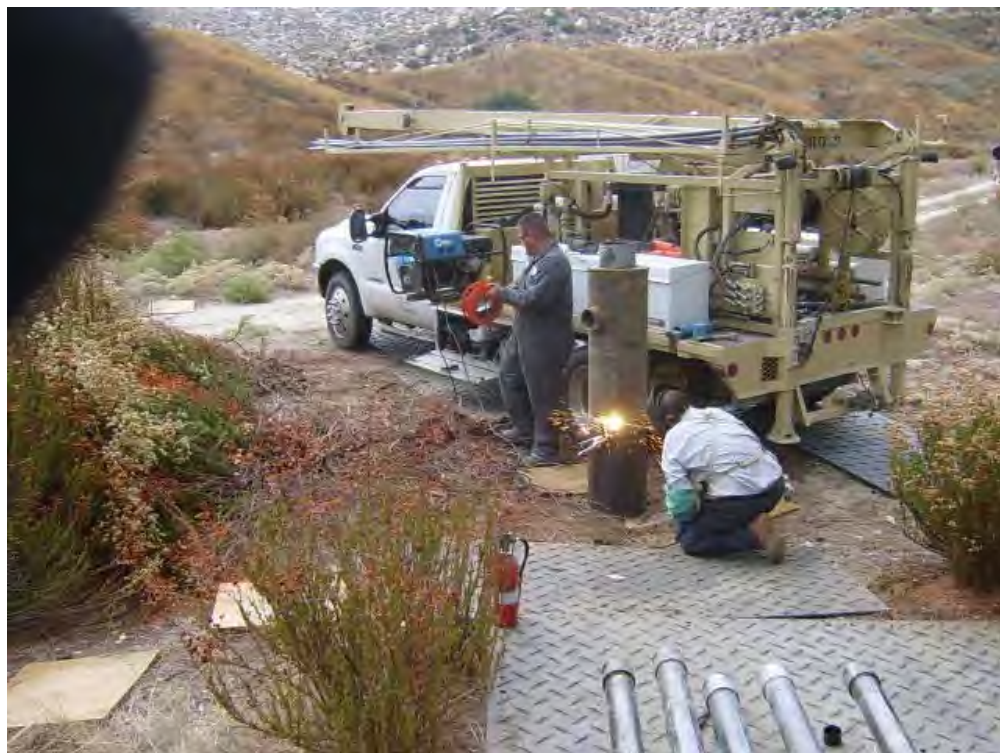
Photo 8: Preparation of Well W-1-5 for abandonment: Fitment of casing extension to capture displaced water during grout filling.
