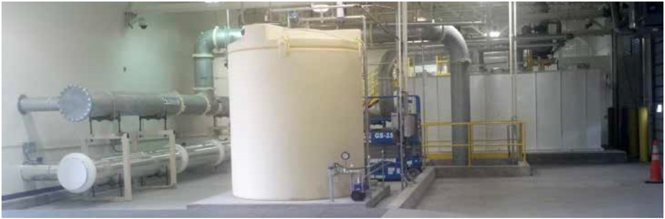
The sub-slab depressurization system (SSDS) ensures safe air quality inside the main building
