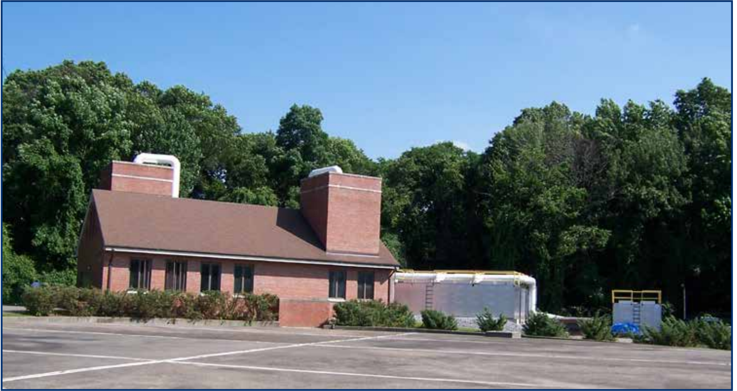
Off-Site (OU2) Groundwater Treatment System
