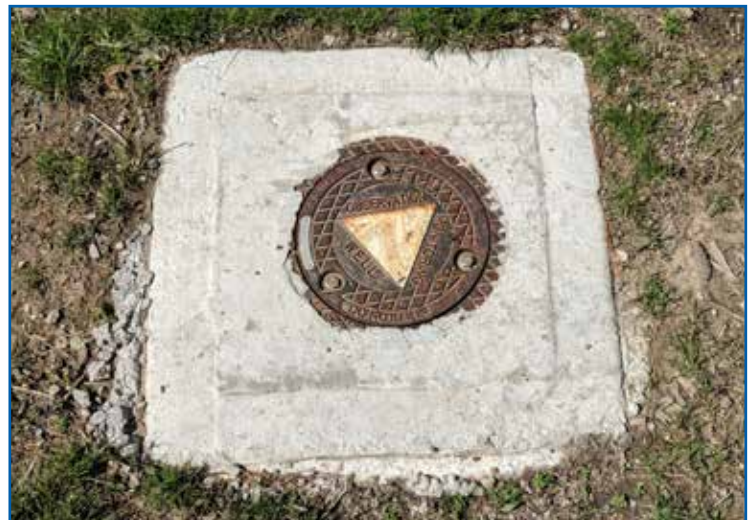
Once installed, the monitoring well sits level with the ground.
