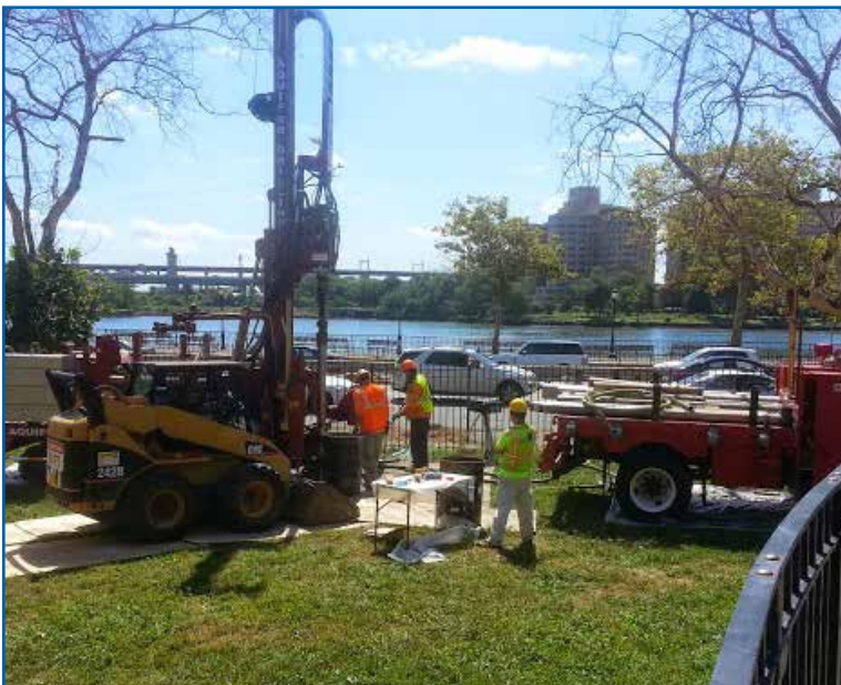
Monitoring well installation equipment is shown as an example.
