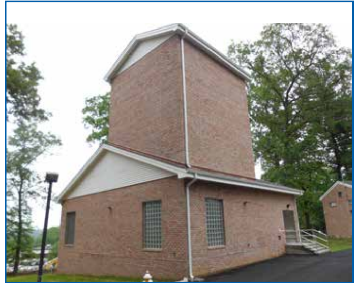
New Manhasset-Lakeville Water District water treatment facility funded by Lockheed Martin to provide clean water to their customers.
