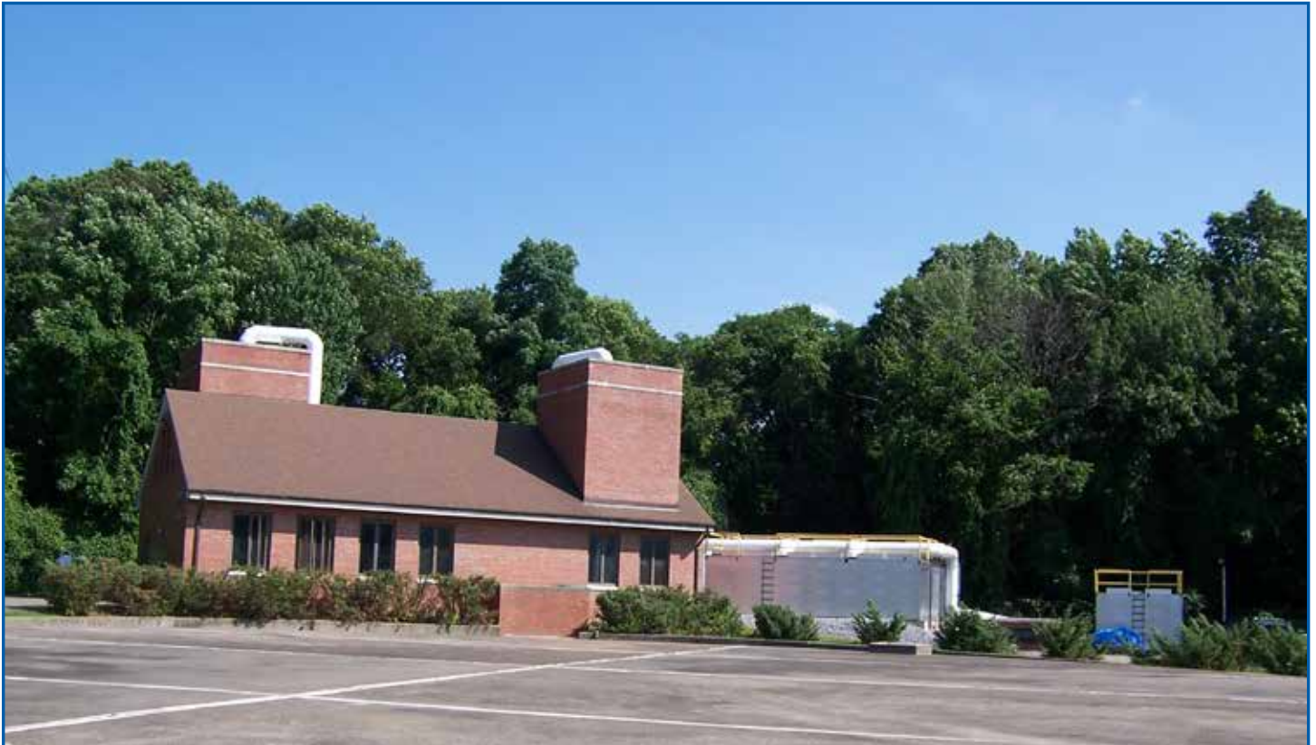
Off-Site (OU-2) Groundwater Treatment System
