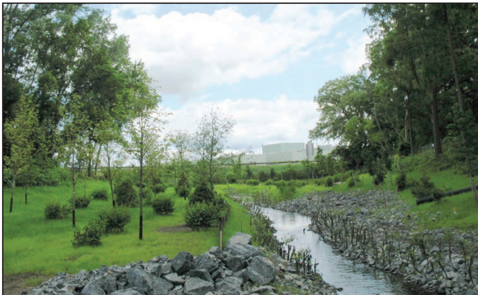
Fully restored upstream portion of wooded area near NYS Thruway.
