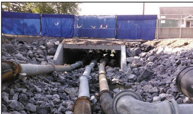
*Bypass pump piping running through the new concrete box culvert underneath Brookview Lane.*
