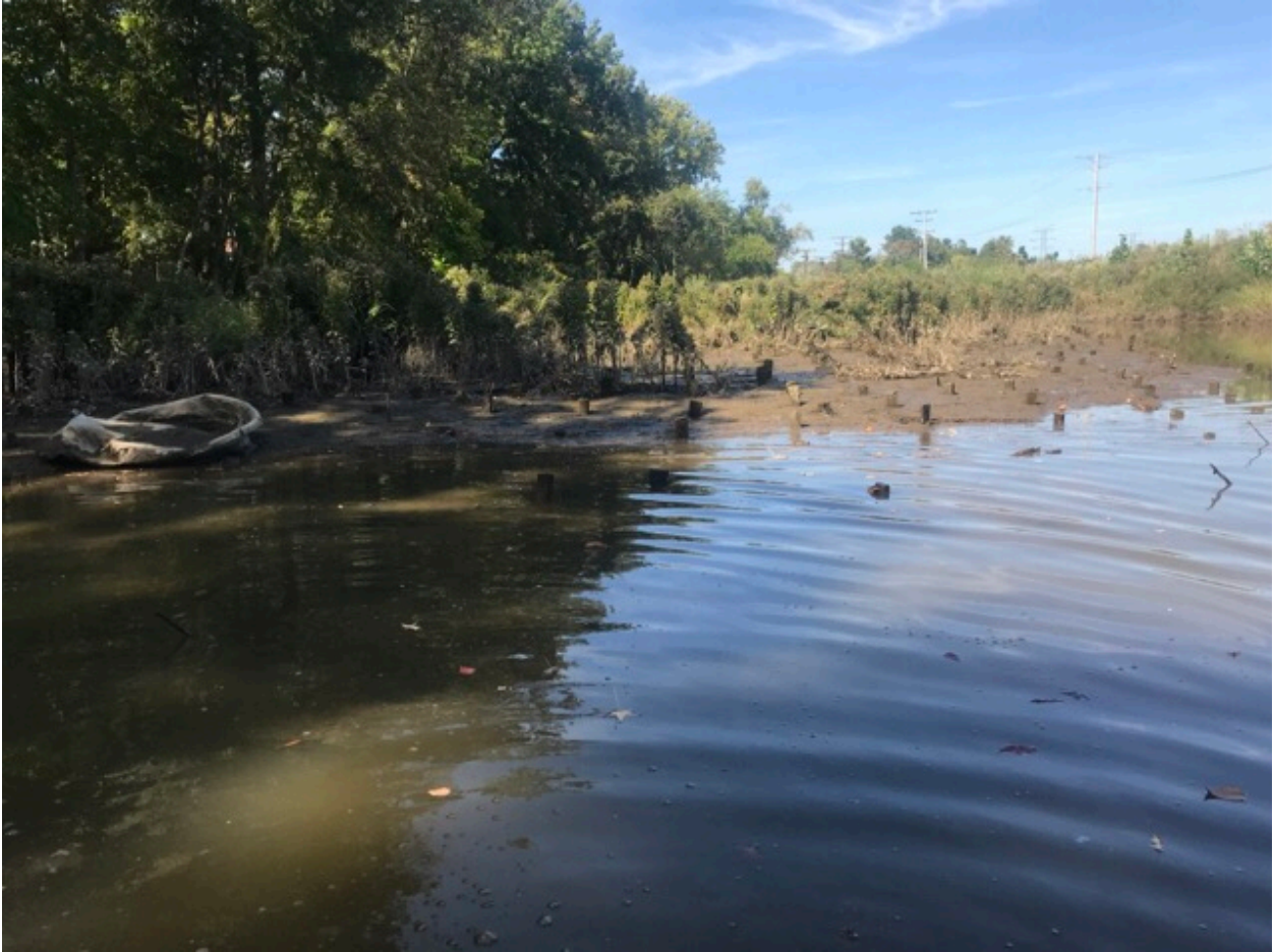
Figure A-29. Right streambank, upstream view at Station 09+26.
