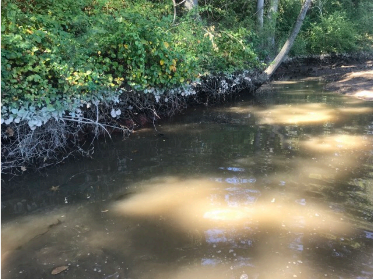
Figure A-25. Right streambank, upstream view at Station 05+93.
