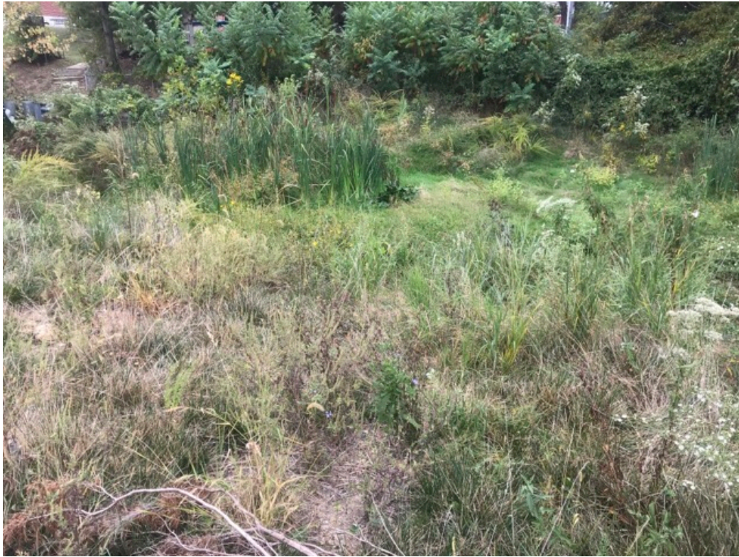
Figure A-102. View from top of floodplain, left streambank at Station 01+30, 2018 (top) and 2019 (bottom).
