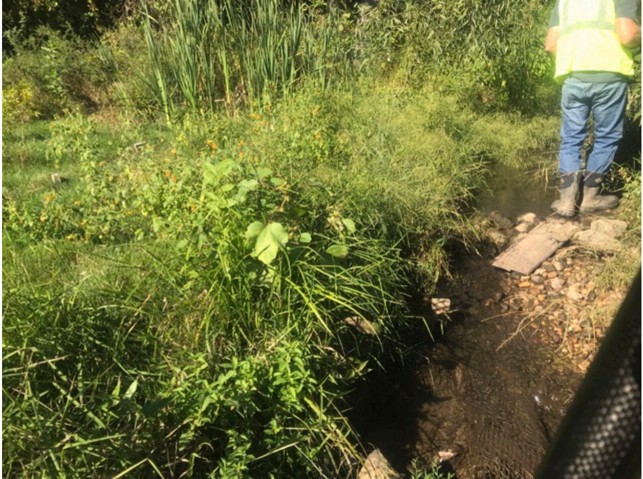
Figure A-4. Right streambank at Station 01+46.
