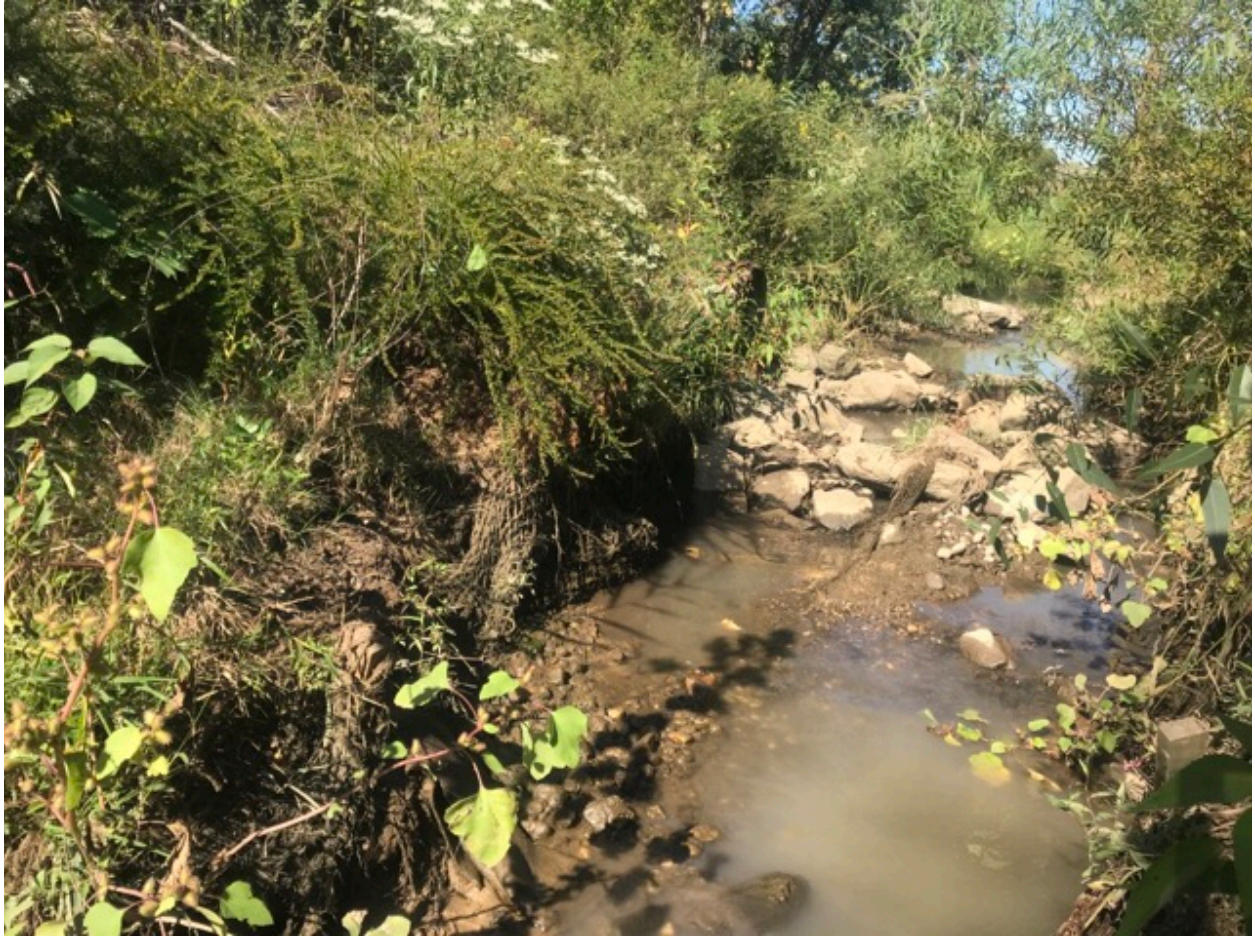
Figure A-14. Right streambank, upstream view at Station 02+27.
