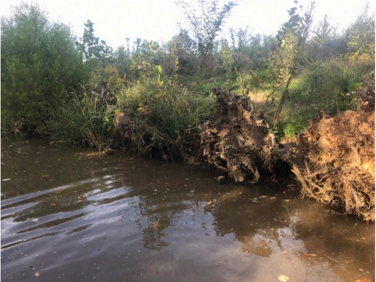
Figure A-22. Left streambank at Station 04+86.
