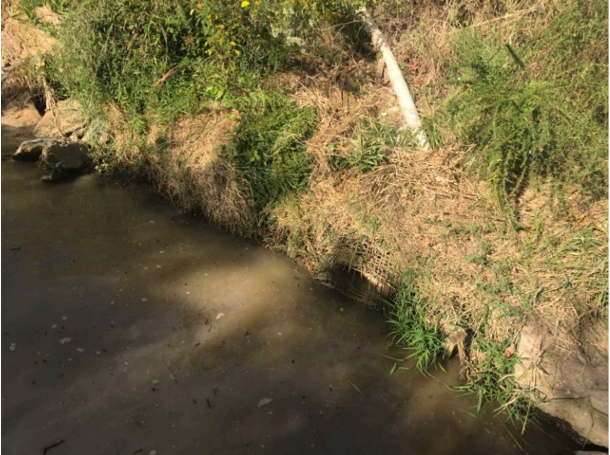
Figure A-10. Left streambank at Station 01+91.
