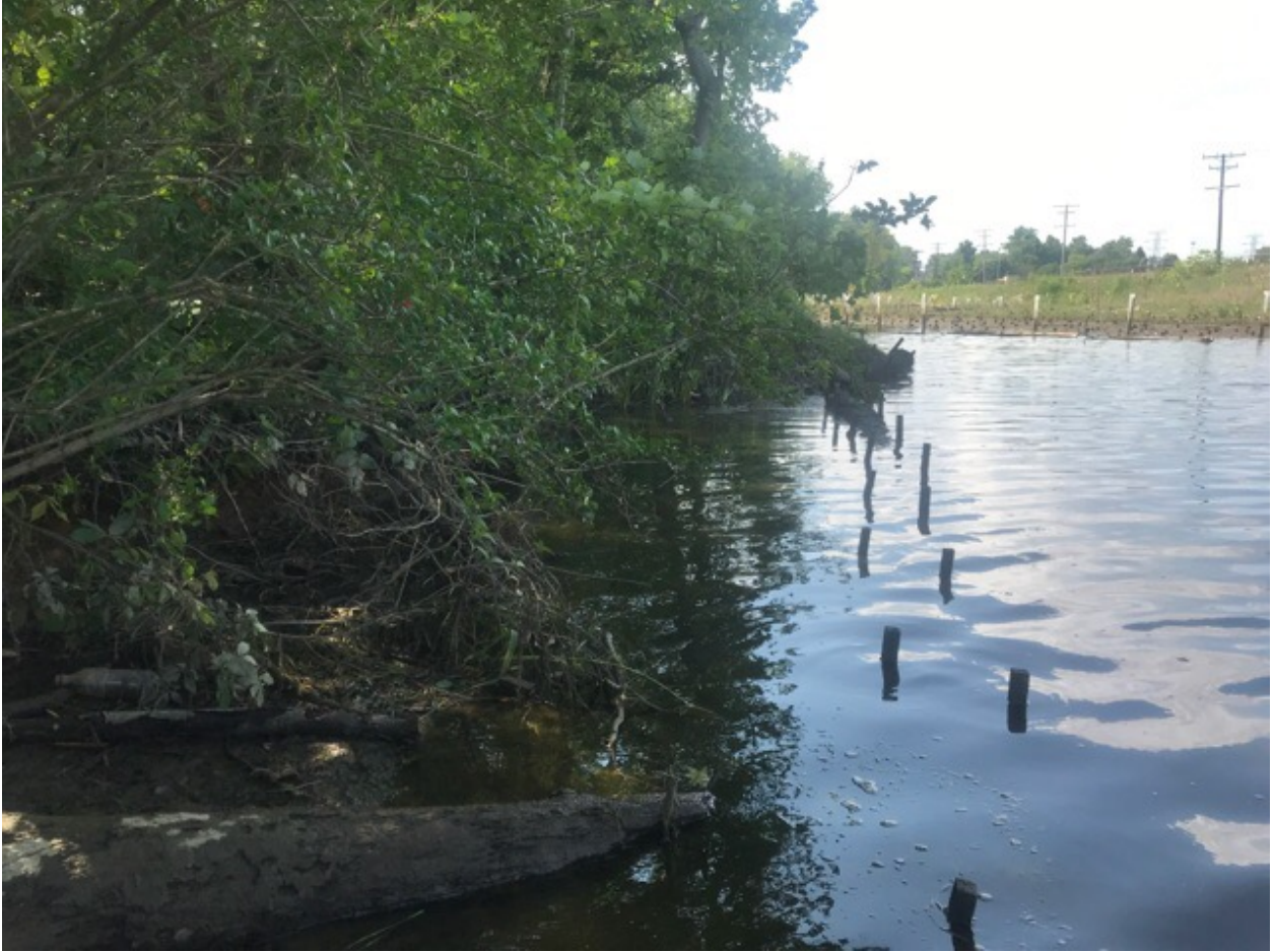
Figure A-28. Right streambank at Station 07+38.
