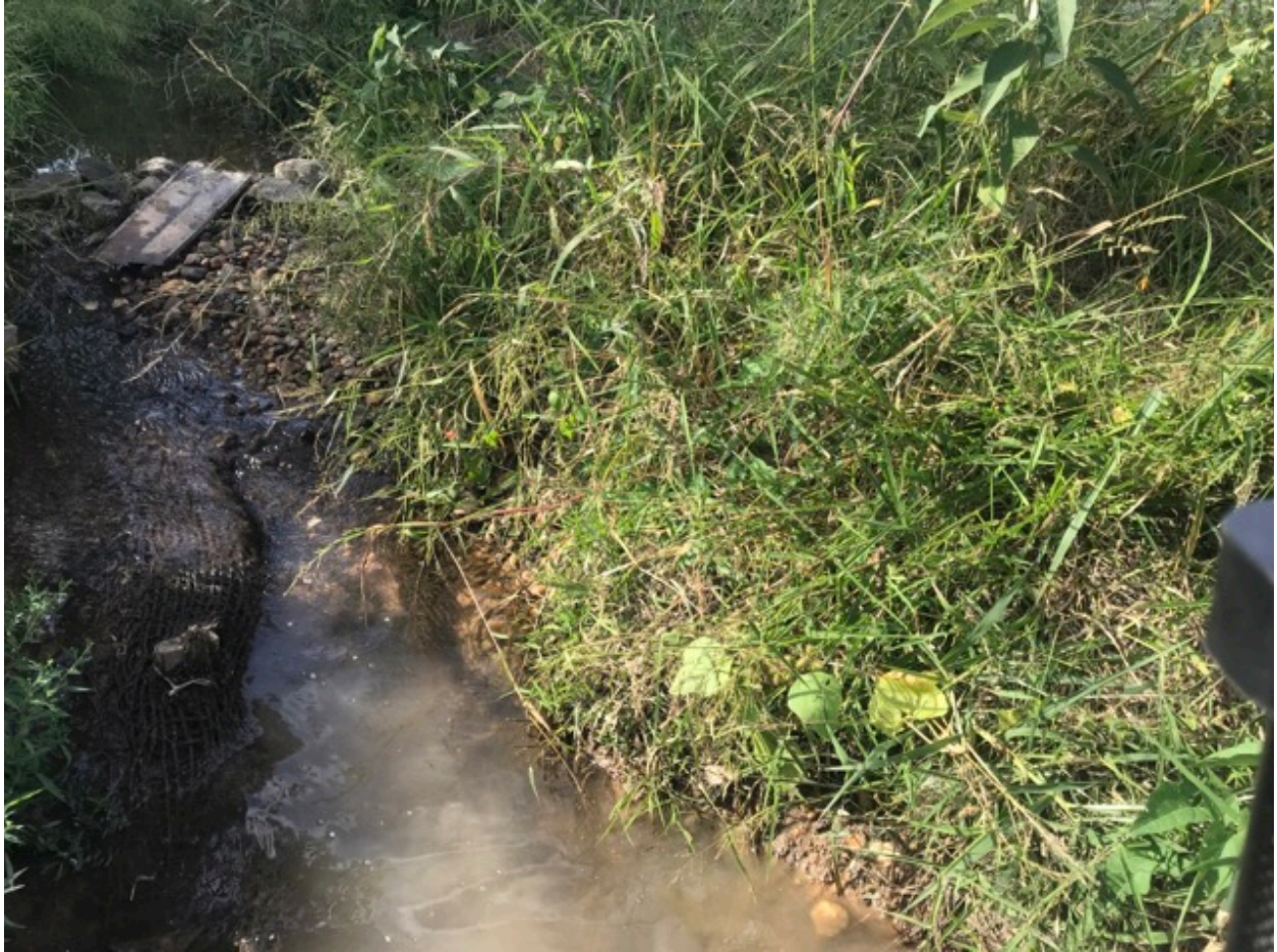
Figure A-5. Left streambank at Station 01+52.
