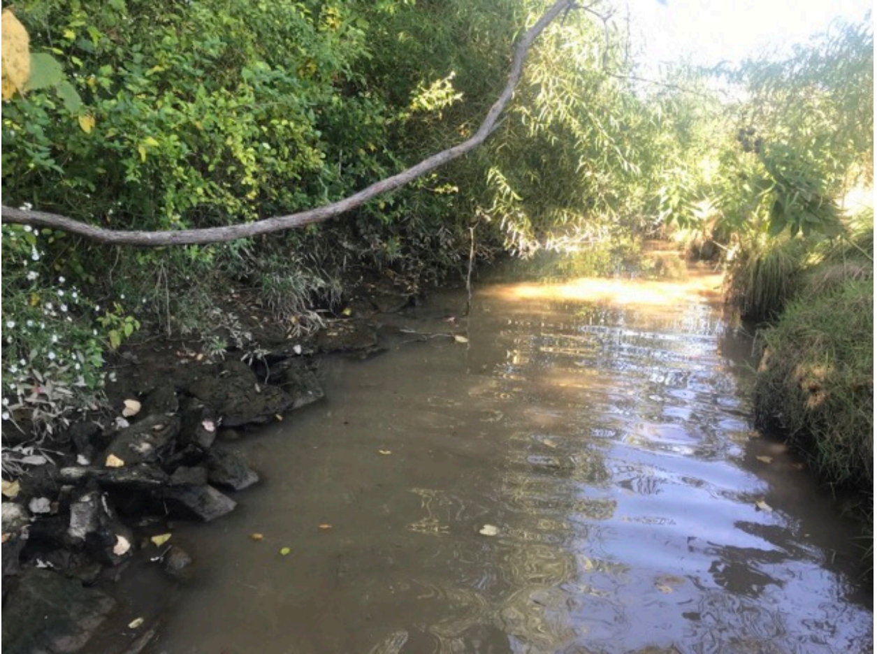
Figure A-16. Right streambank, upstream view at Station 03+80.
