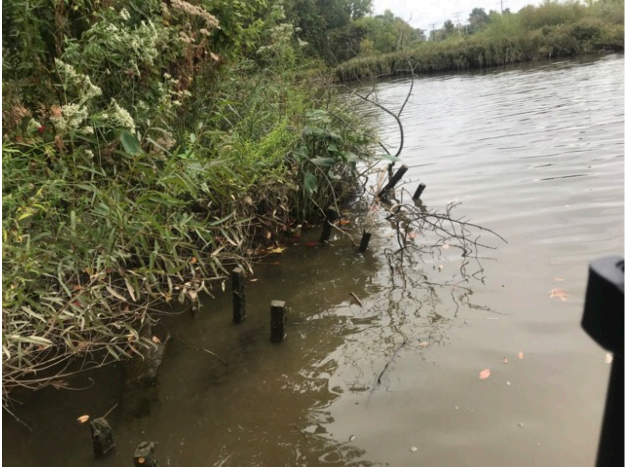
Figure A-34. Right streambank, upstream view at Station 10+97.
