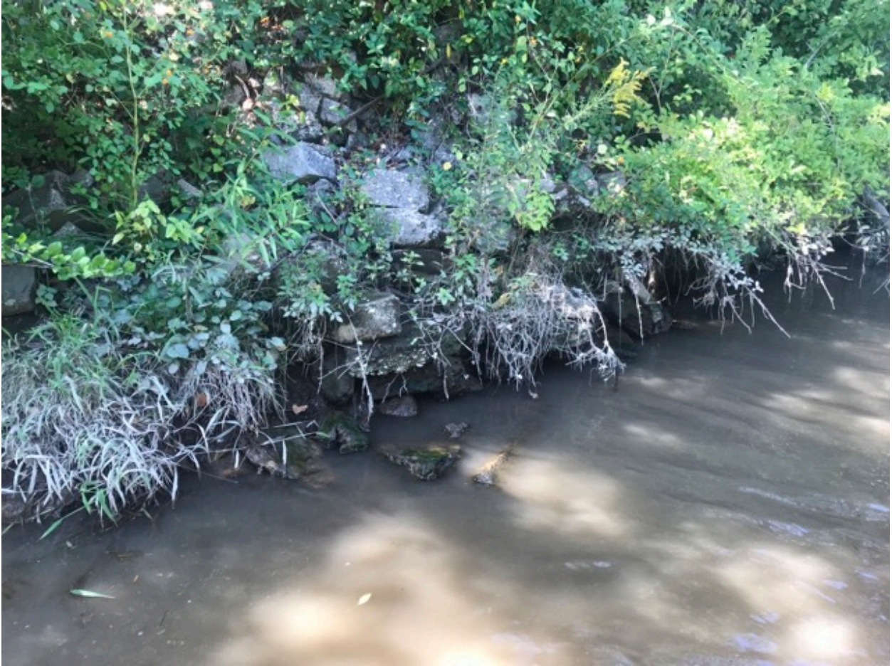
Figure A-19. Right streambank at Station 04+19.
