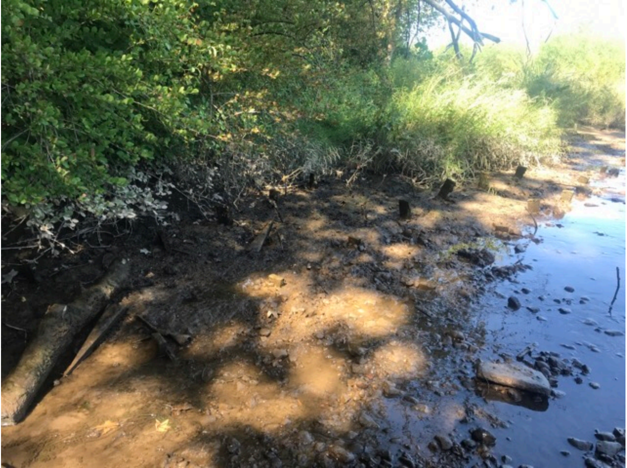
Figure A-24. Right streambank, upstream view at Station 05+41.
