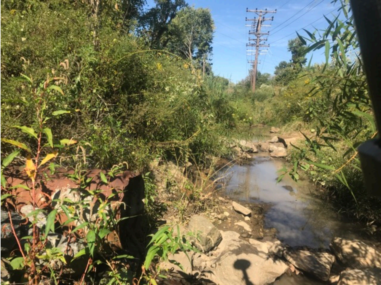
Figure A-12. Right streambank, upstream view at Station 02+14.
