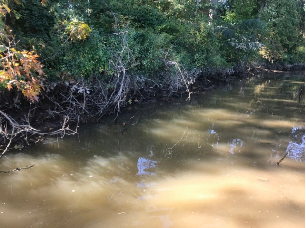
Figure A-26. Right streambank at Station 06+82.
