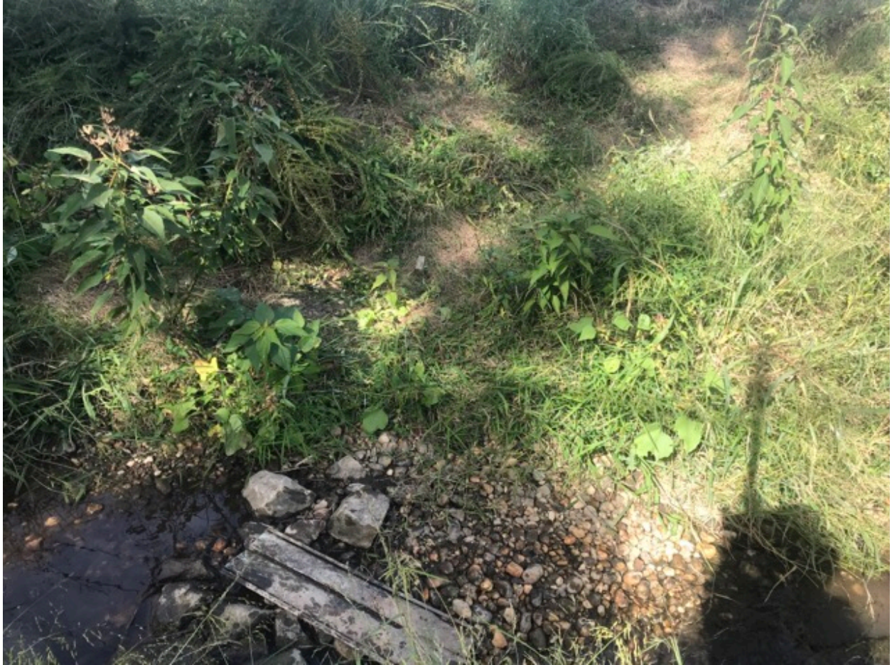
Figure A-3. Left streambank at Station 01+45.
