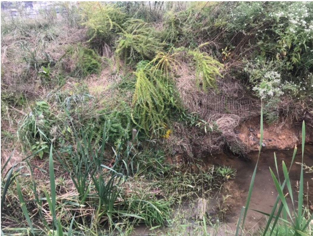
Figure A-72. Soil eroding from under the matting on the lower left bank at Station 01+55, 2018 (top) and 2019 (bottom).
