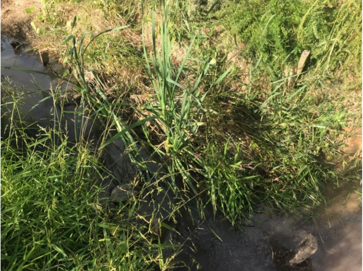
Figure A-8. Left streambank at Station 01+66.
