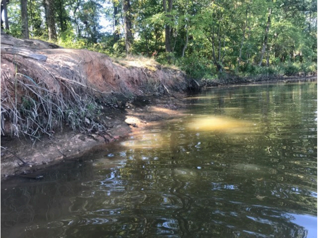
Figure A-32. Right streambank, upstream view at Station 09+98.
