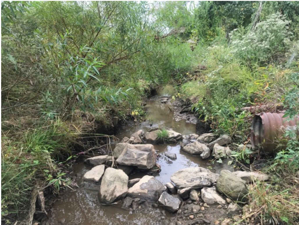
Figure A-75. Downstream view from thalweg at Station 02+00, 2018 (top) and 2019 (bottom).
