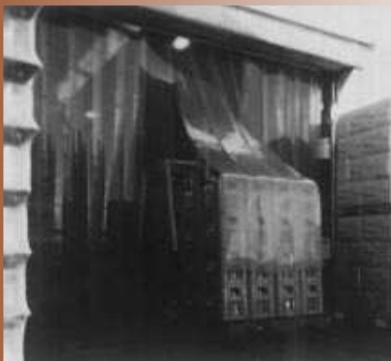
Clear vinyl strip installed on loading dock door allows easy access while offering thermal protection and noise reduction.
