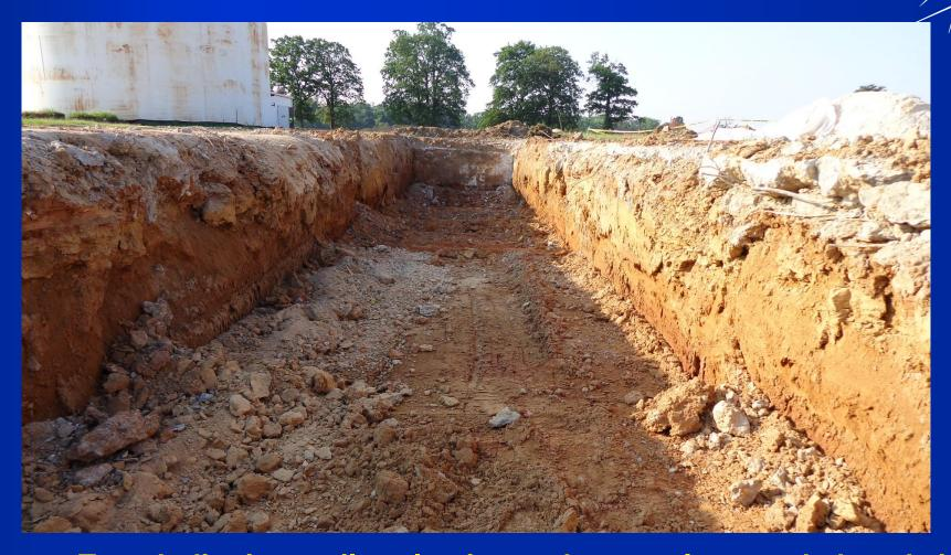
Trench digging, soil evaluation and removal as needed, and site preparation began in June 2013 in preparation for groundwater treatment system construction. Initial work was performed at Block E, the location of the former Building D, in the area near the water tower.
