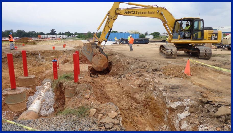
The second unexpected underground storage tank, which had contained TCE, was removed for proper disposal.
