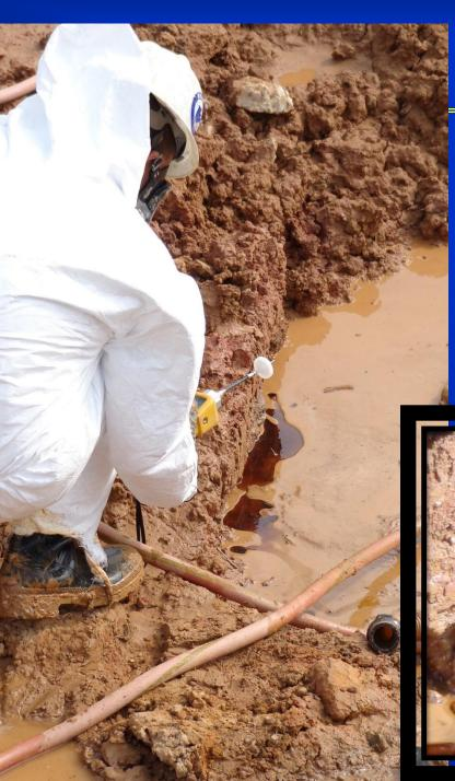
A second unexpected underground storage tank contained trichloroethene (TCE), water and sediment, requiring additional worker protection measures be taken, and expanded air monitoring to help identify contaminants. The tank contents were drained and properly disposed.
