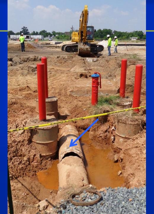
A broken storm pipe is discovered and needed repair before being returned to use.
