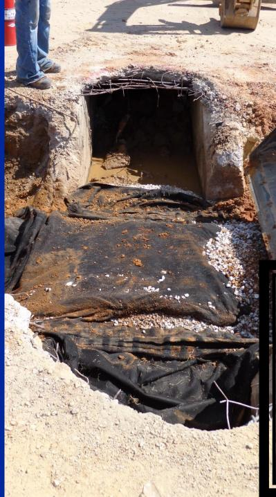
Complications uncovered during construction included discovery of ventilation ducts (left), French drains (below), and other infrastructure located beneath former Building D, which unfortunately served to collect
