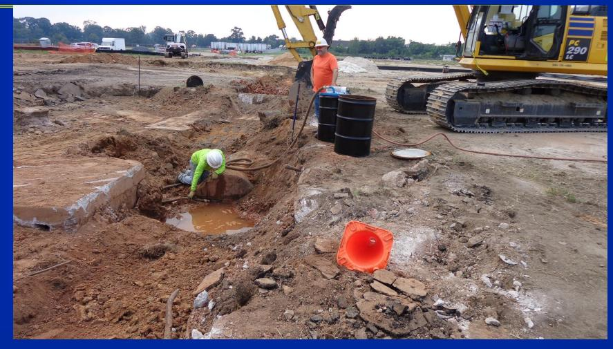
The first unexpected underground storage tank held waste water and had stored petroleum/diesel. Contents were drained, drummed and tested for proper disposal.
