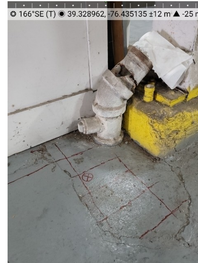
Rebar locations at 4-DHB
