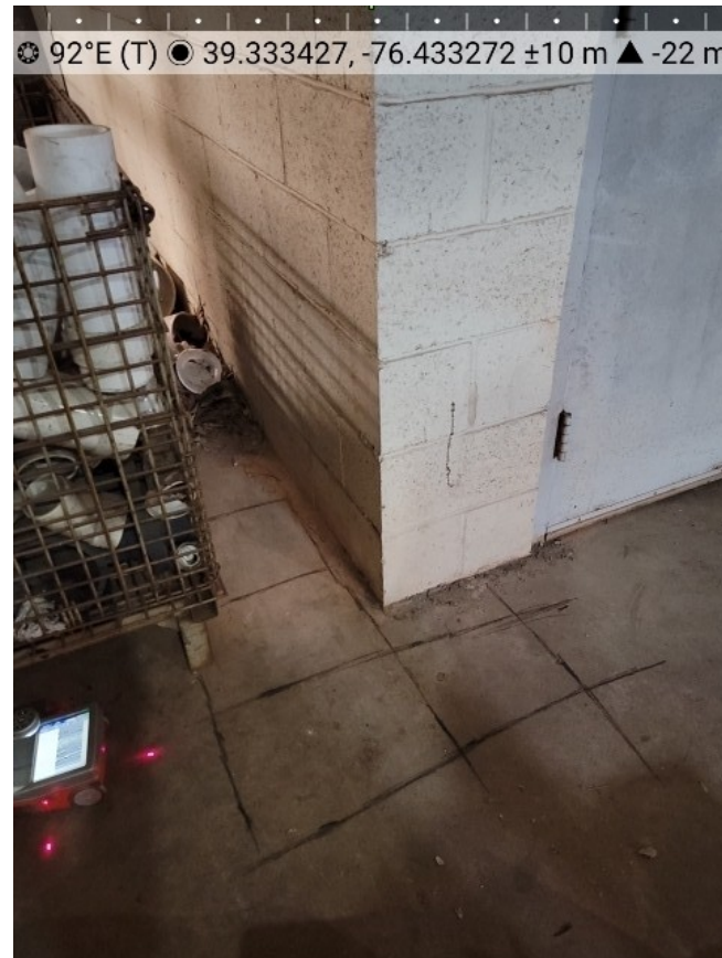
Rebar locations at 6-DHB
