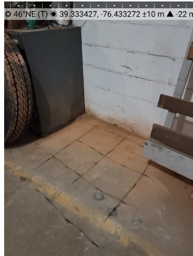
Rebar locations at 7-DHB
