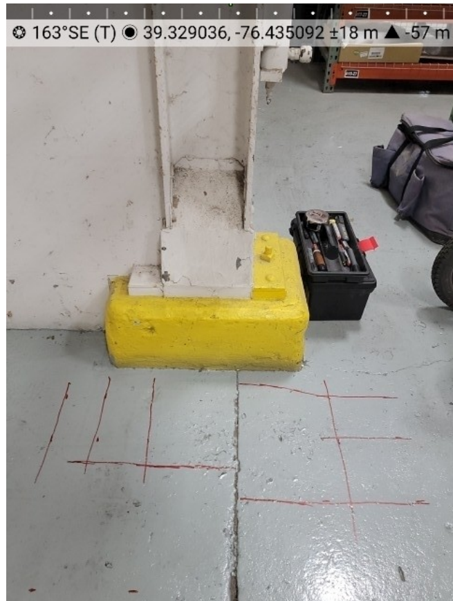
Rebar locations at 5-DHB
