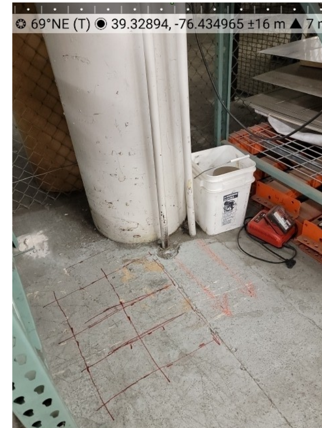
Rebar and water lines at 1-C
