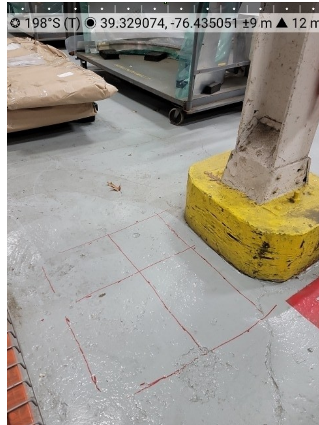
Rebar locations at 3-DHB
