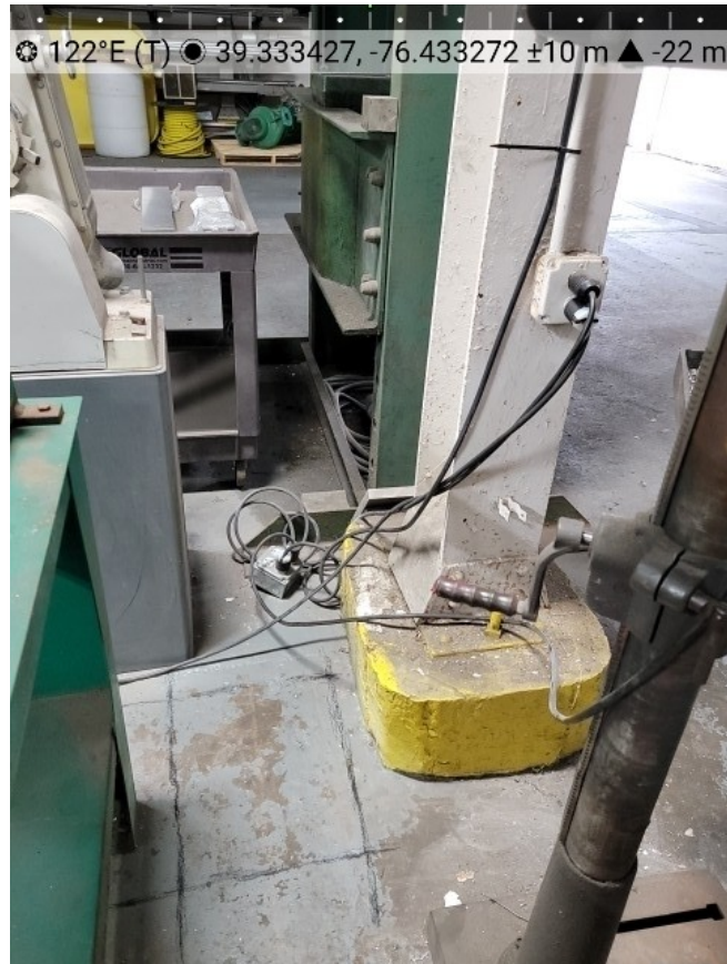
Rebar locations at 1-DHB
