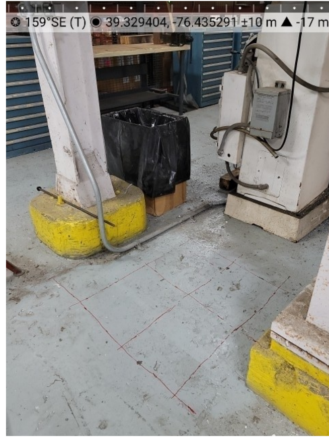
Rebar locations at 2-DHB
