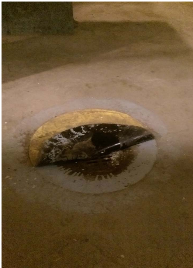
Photo 4 – Large cover plate (CP) with 92.11 ppb detection of trichloroethene using the Frog 4000™ .
