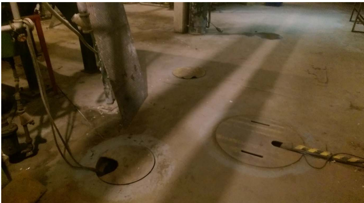
Photo 6 – Broad view of three features (cover plate, sump pit, and floor drain) with elevated trichloroethene detections using the Frog 4000™ near column D24.
