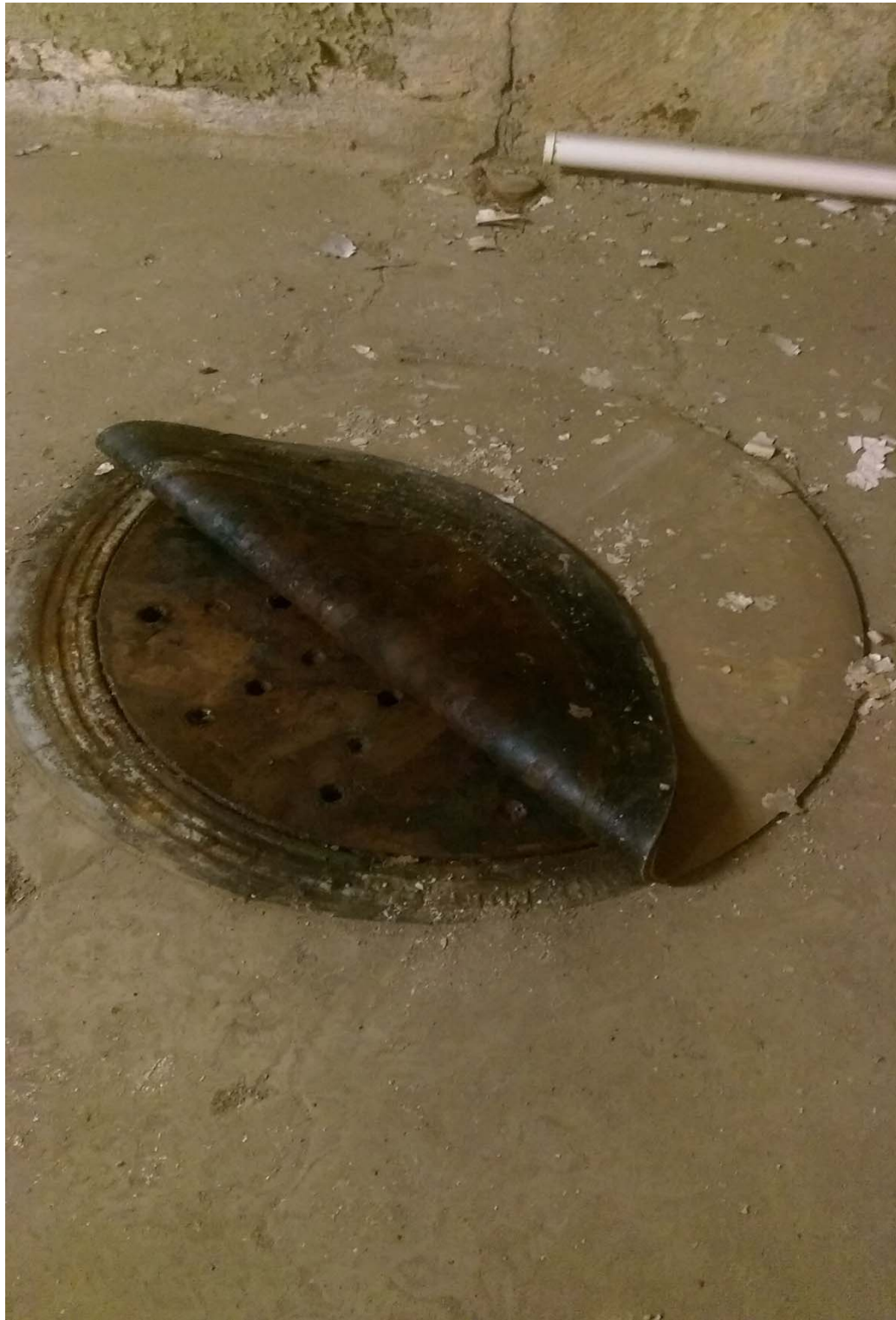
Photo 2 – Possible sanitary grate with previous 16 ppb trichloroethene (TCE) hit during first HAPSITE™ survey. Recent Frog 4000™ survey TCE detections were 9.69 ppb and 13.67 ppb with cover open, 9.82 ppb in the breathing zone, and 5.10 ppb when covered.
