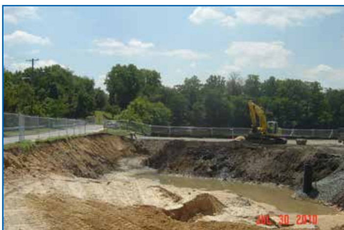
Deep soil excavation will use either sheet piles pictured above or sloped side walls pictured below.
