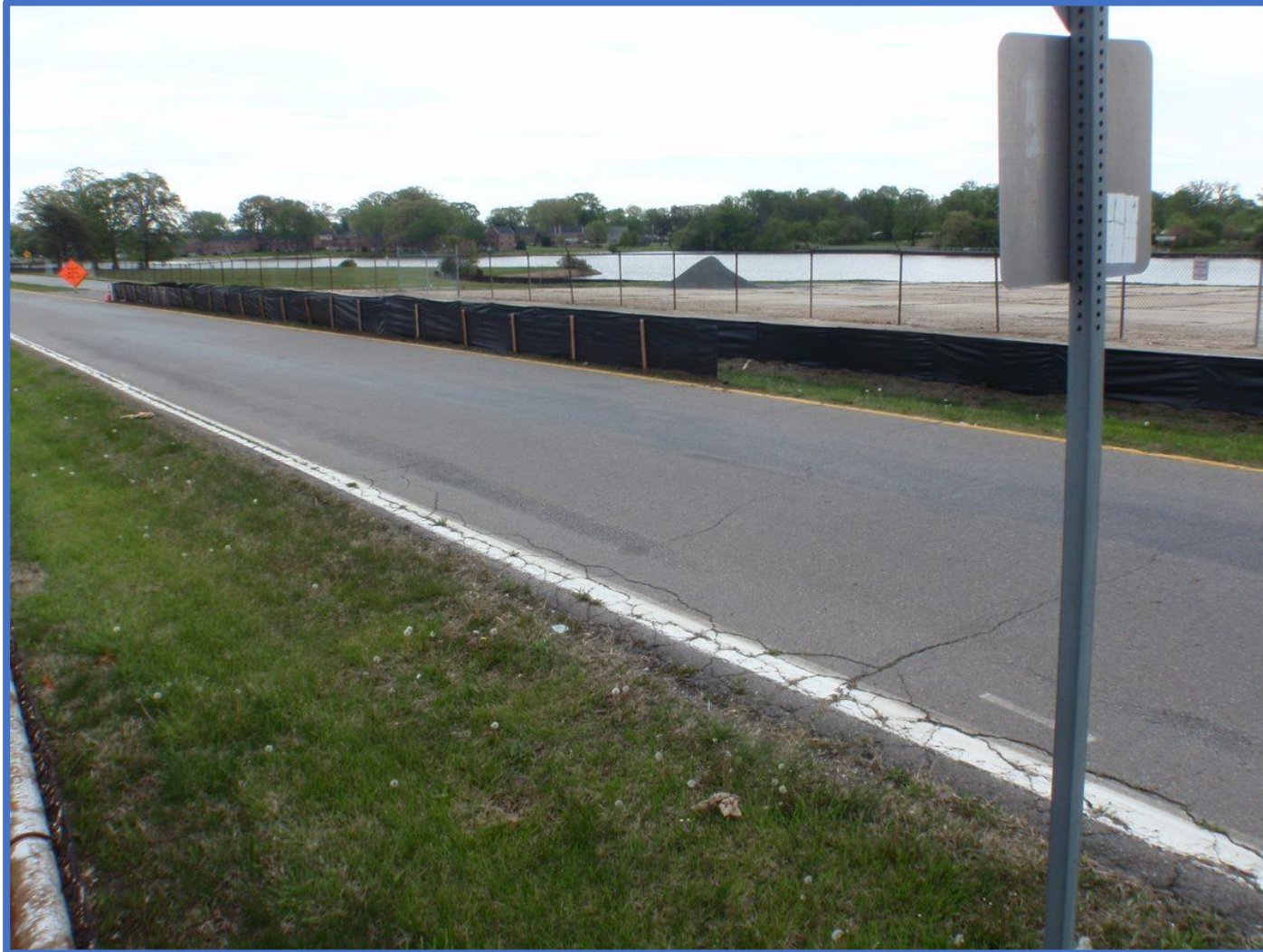
Silt fences protect the surrounding area from storm water runoff.
