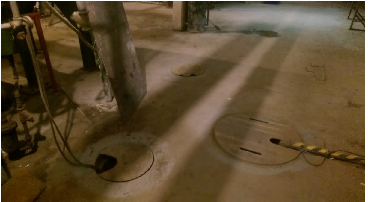
Photo 6 – Broad view of three floor features (SP1, FD1 and other sump) located near column D24.
