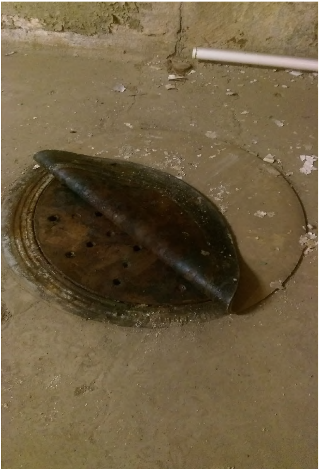
Photo 2 – Storm drain lid (SD1) located west of Column D26.
