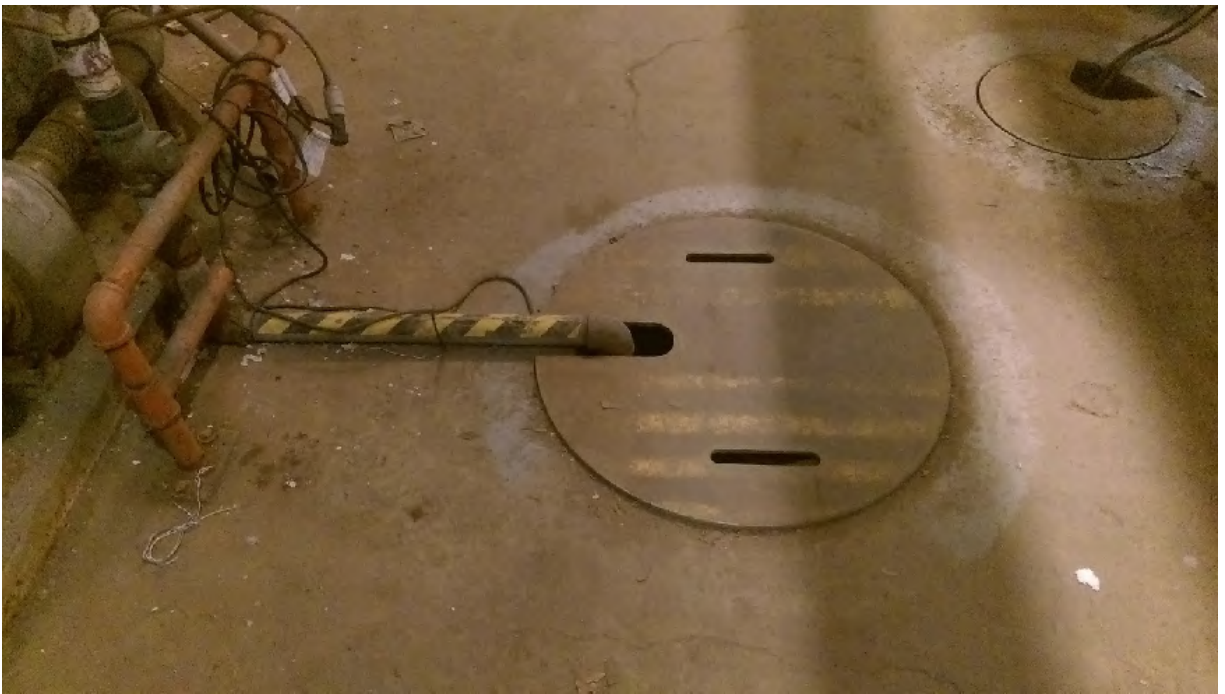
Photo 4 – Large cover plate (SP1) located near Column D24.
