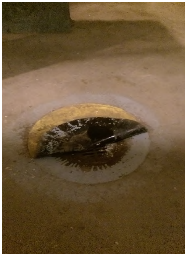
Photo 5 – Covered floor drain (FD1) located near Column D24.
