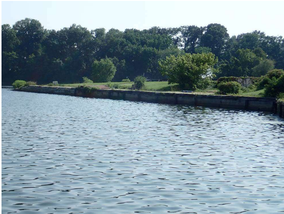
Photograph 5. Seawall Section “H”, looking west.
