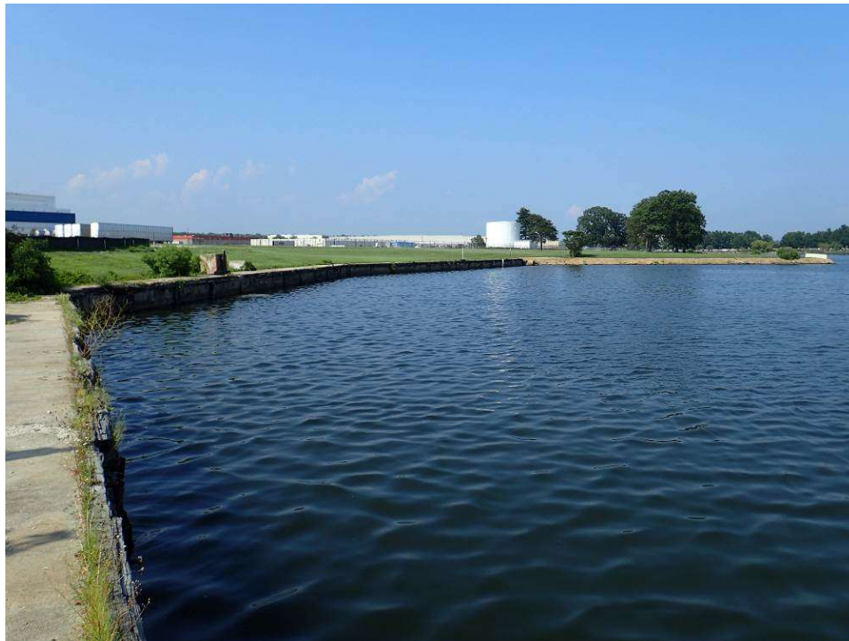
Photograph 2. Seawall Sections “E”, “F”, “G” and “H”, looking northeast.
