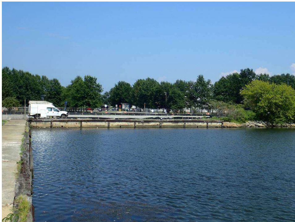
Photograph 4. Seawall Sections “A” and “B” (foreground), looking northwest.
