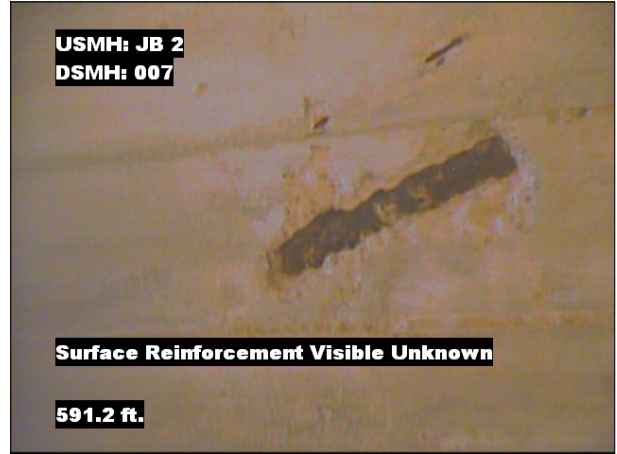
Photo: JB_2_007_SRVZ_591.2.jpg, VCR No.: 1 591.2FT, Surface Reinforcement Visible Unknown, at 12 o'clock, within 8 inches: NO
