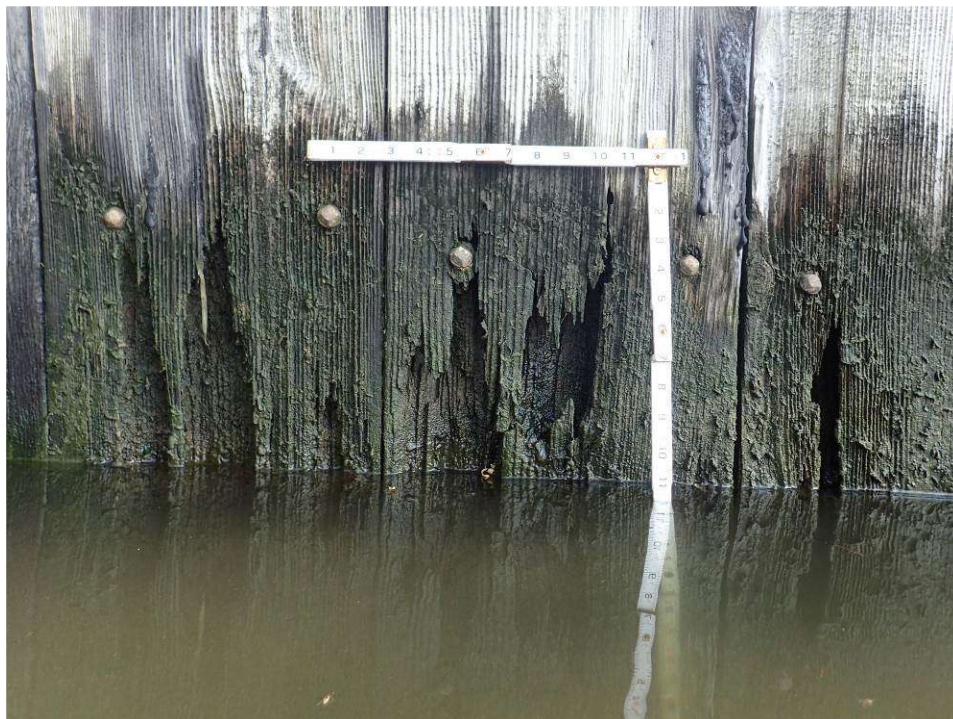
Photograph 8. Typical timber seawall detail at waterline.
