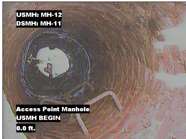
Photo: MH-12_MH-11_AMH_0.0.jpg, VCR No.: 1 0FT, Manhole
