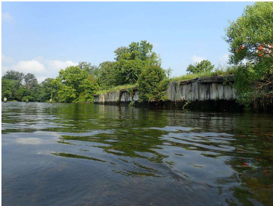
Photograph 6. Separate timber wall located west of Section “H”, looking north
