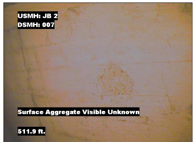
Photo: JB_2_007_SAVZ_511.9.jpg, VCR No.: 1 511.9FT, Surface Aggregate Visible Unknown, at 12 o'clock, within 8 inches: NO
