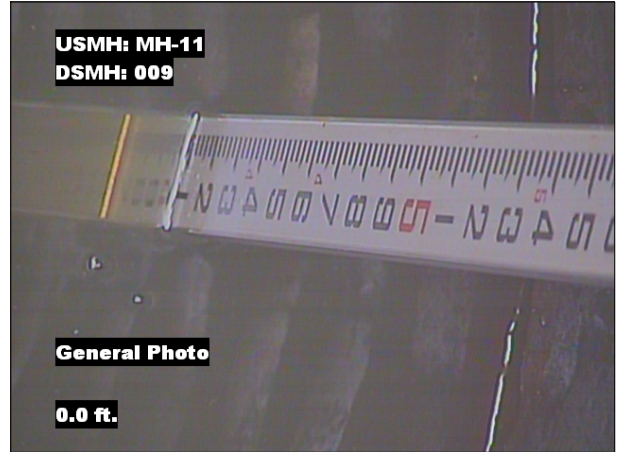
Photo: MH-11_009_MGP_0.0.jpg, VCR No.: 1 0FT, General Photograph
