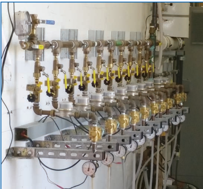
Equipment inside the trailer distributes lactate (sugars) and water through a system of underground injection wells to activate bioremediation.
