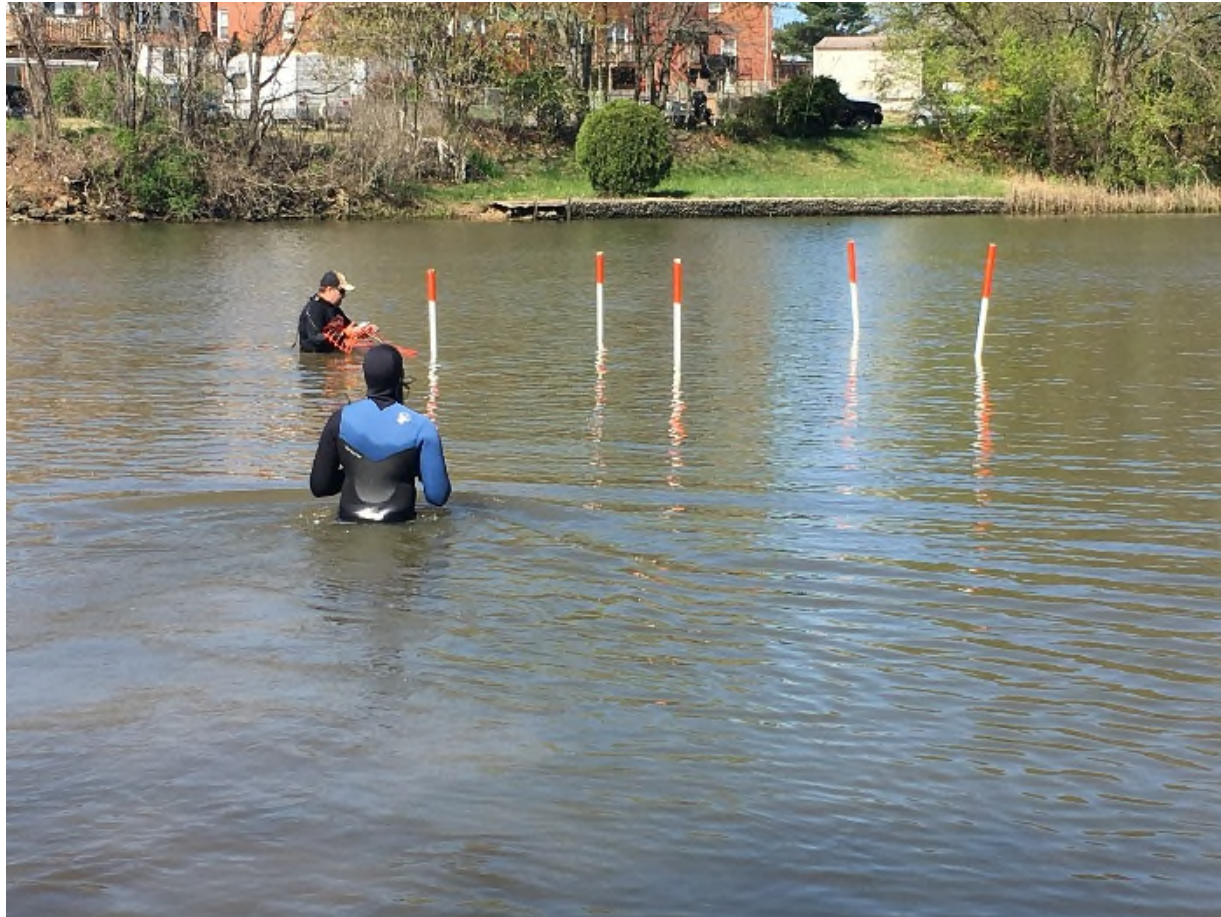
Figure 8 Constructing Exclosure in Cow Pen Creek
