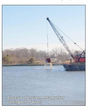
dredging for this project. While both methods have advantages and neither is perfect, the United States Army Corps of Engineers (USACE) states that the two methods are considered equal in terms of the quantity of sediments stirred up in the waterway (USACE, 2008 - Technical Guidelines for Environmental Dredging of Contaminated Sediments).
