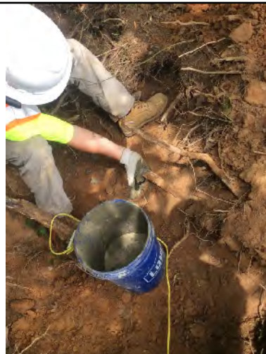
Non-shrink grout used to seal pipe prior to backfilling.
