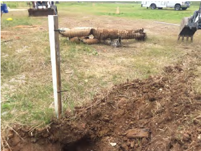
Eta piping removed from the bank
