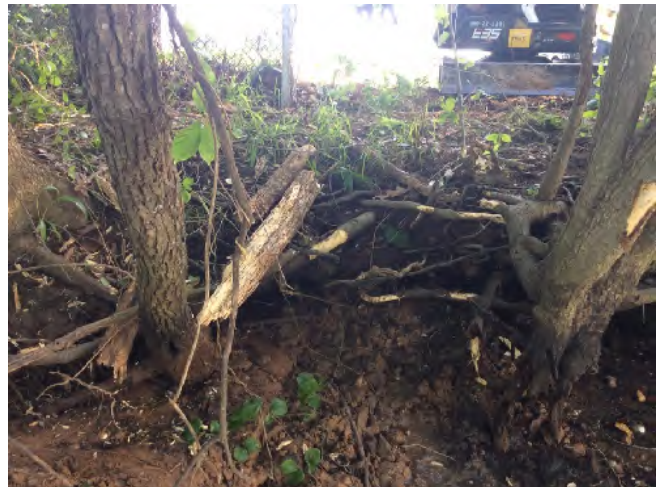
Bank after protruding terra cotta piping was removed
