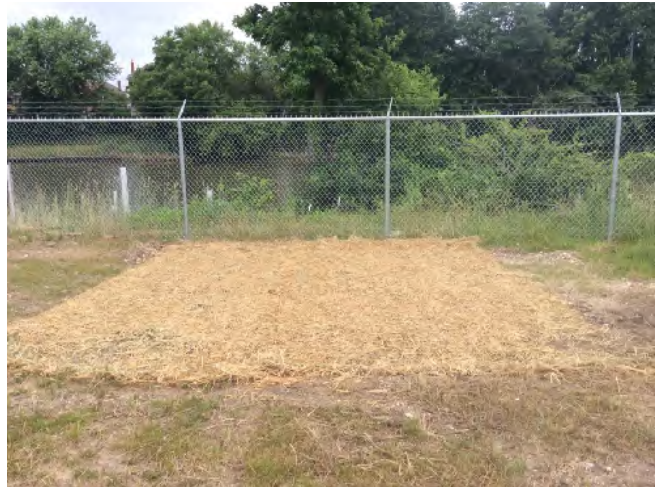
Disturbed area restored with curl-x and grass seed
