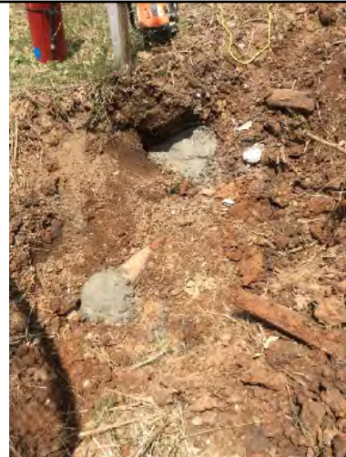
Eta north and south saw cut and filled with concrete.
