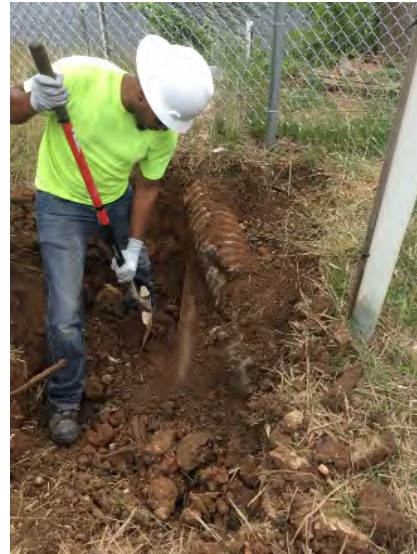
Eta north and south located via mini excavator and hand digging.
