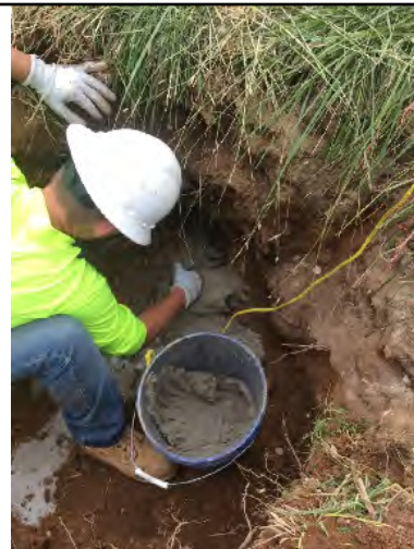
6" CMP sealed with concrete.
