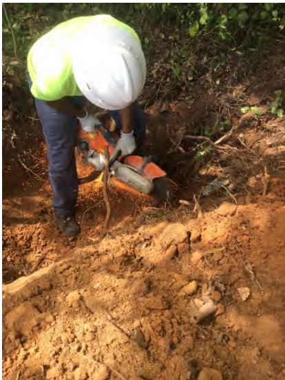
Steel pipe saw cut and removed.
