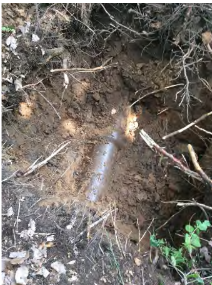
Terra cotta pipe located inside perimeter fence
