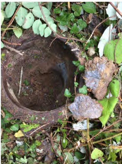
Surface vertical pipe to zeta located and already filled with grout
