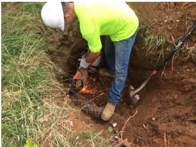
Elite personnel saw cutting 6" CMP
