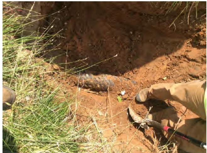
6" pipe located via mini excavator
