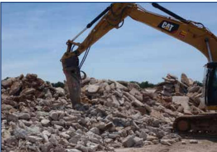
Uncontaminated concrete is broken into manageable sized pieces then removed and recycled offsite or reused onsite for fill.
