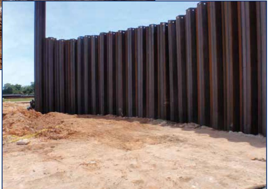
*Temporary shoring is installed where deeper soils are to be removed. The area shown here will be excavated to 20 feet deep, and is the deepest excavation.*
