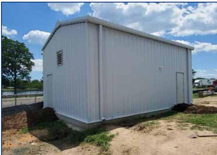
*The building is under roof and walls have been erected and insulated.*
