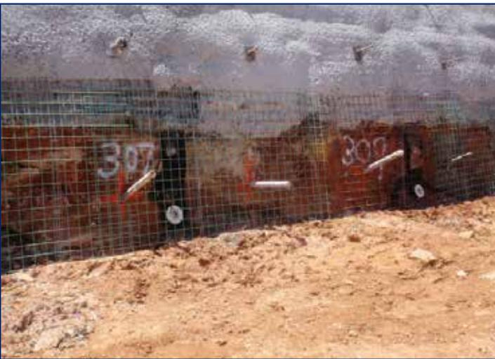
*A soil nail wall has been installed to create a stable side wall for the excavation area. The western portion of the Block E work area is adjacent to Tilley Chemical, and a steep wall has been temporarily created where soil needed to be removed to access the underlying former building slab.*
