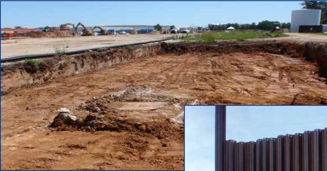
*Soil removal depth relies on former investigations. Once soil is removed to the anticipated depth, the floor and side walls are sampled to confirm contamination removal meets planned goals.*
