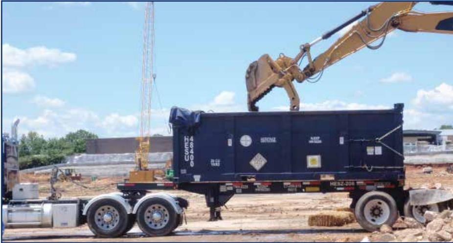
Soils contaminated with polychlorinated biphenyls (PCBs) are stored onsite in a lined and contained area, then loaded into lined trucks (above), then covered with tarp (right) before leaving the site for disposal at a licensed landfill. Truck containers are shipped by rail for most of their trip to the landfill.
