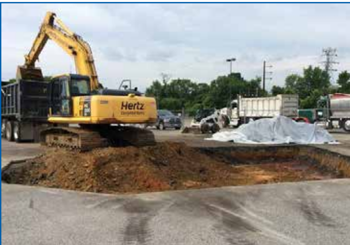
Excavation under asphalt parking lot in Block H
