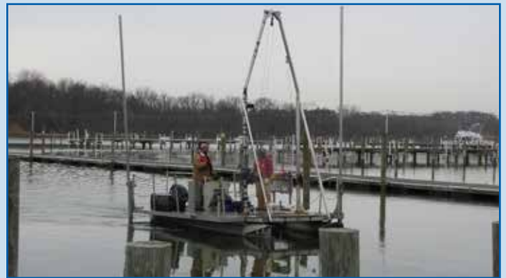
Pontoon boat heads out to install water flow sensors
