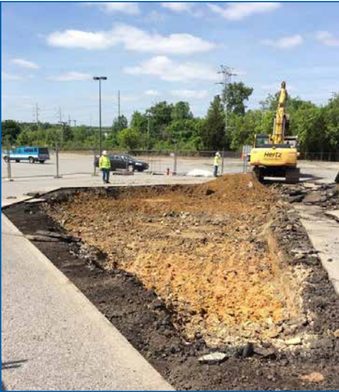
Excavation under asphalt parking lot in Block H
