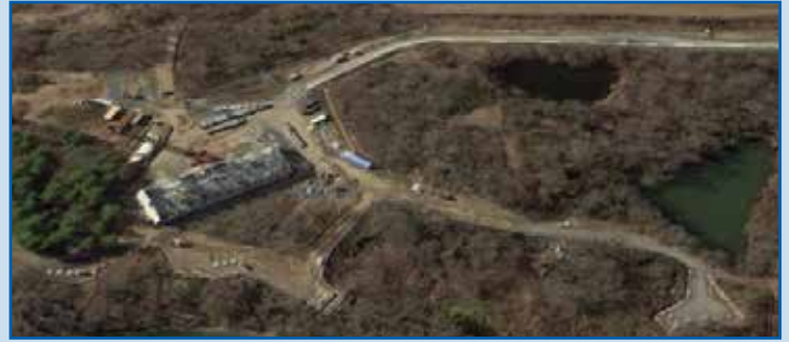
Martin State Airport groundwater treatment plant under construction.
