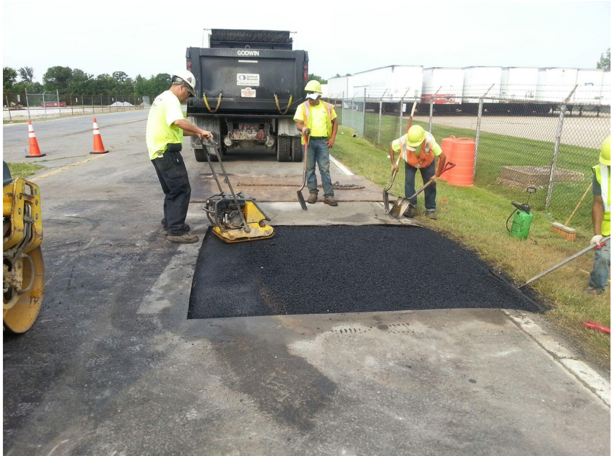
Vibratory tamping of first course hot-mix asphalt (bituminous concrete)
