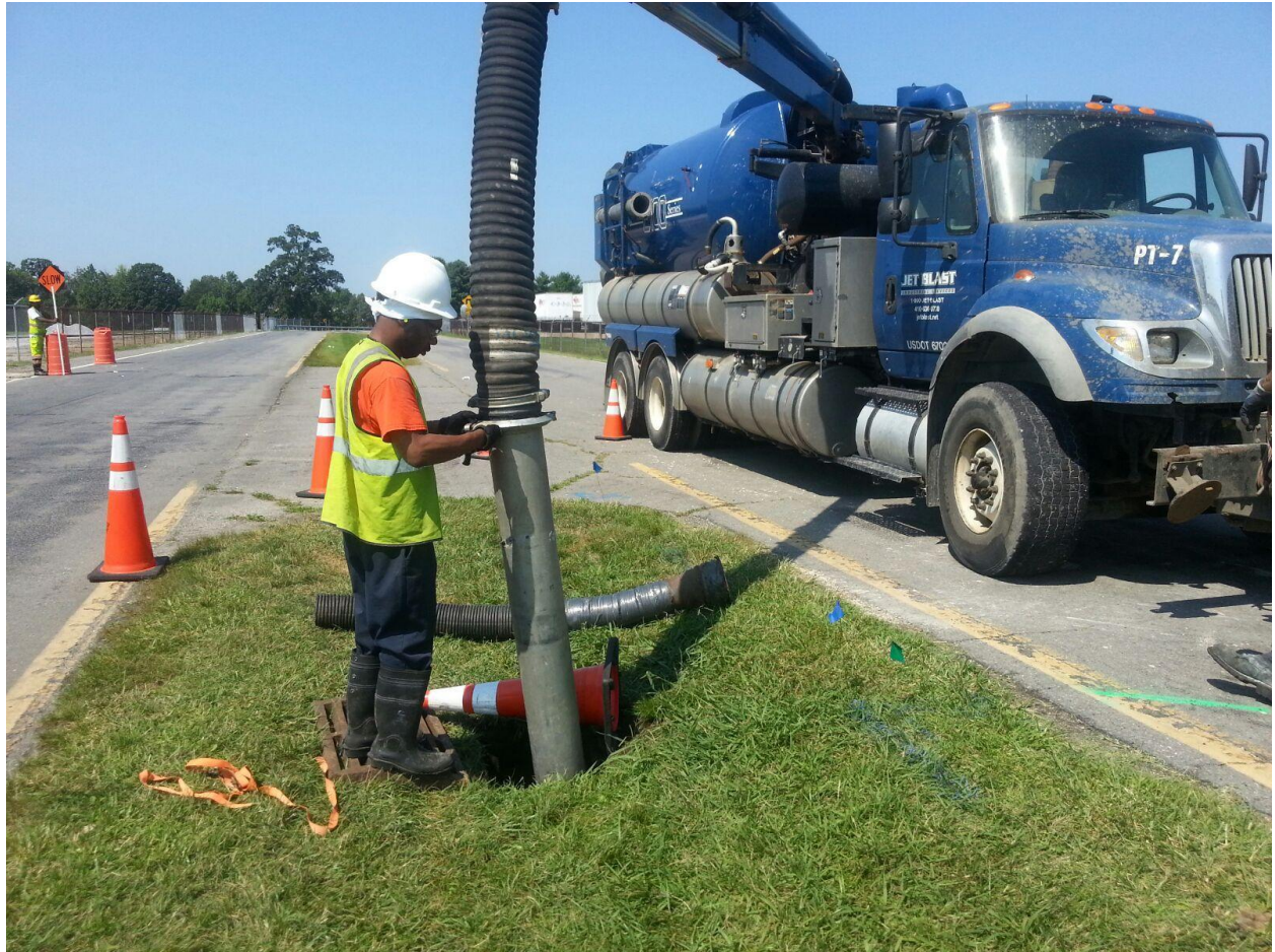
Vacuum truck removing water and residual sediment at catch basin IL-30
