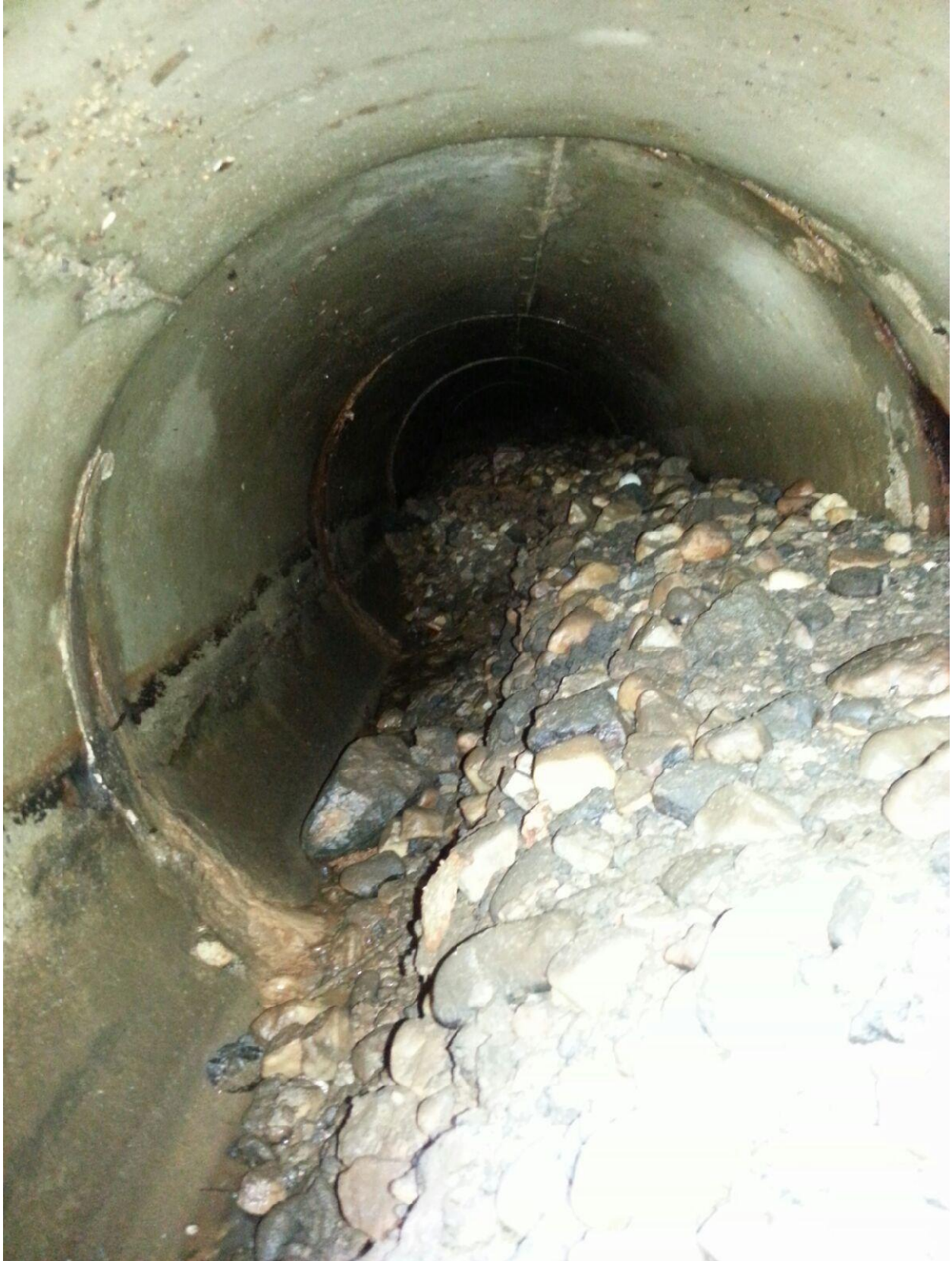
Sediment accumulation in storm drain pipe IL-30A-looking north (upstream)
