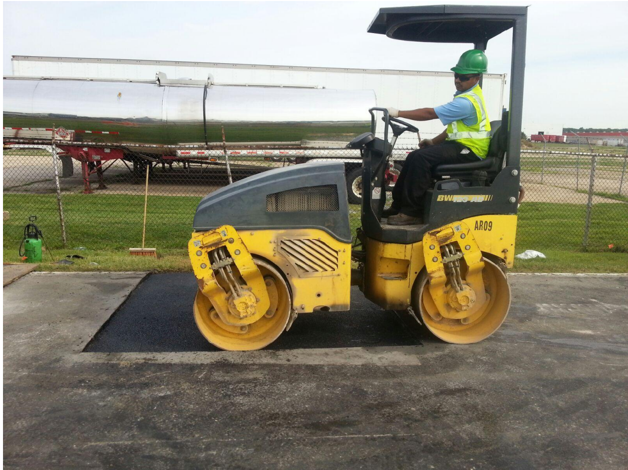
Mechanical drum rolling of first course hot-mix asphalt (bituminous concrete)
