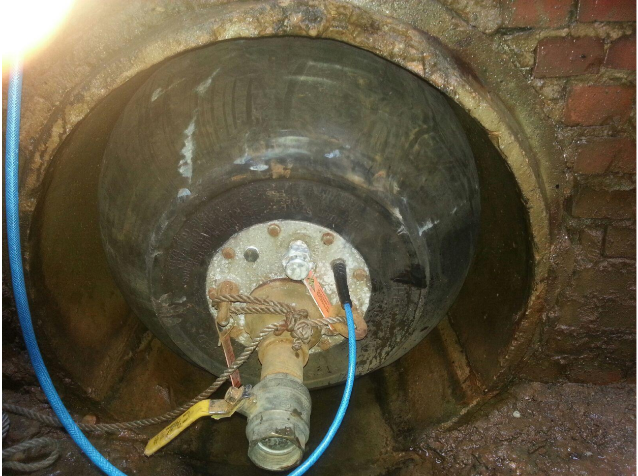
Temporary inflatable commercial-grade sewer plug in MH-3
