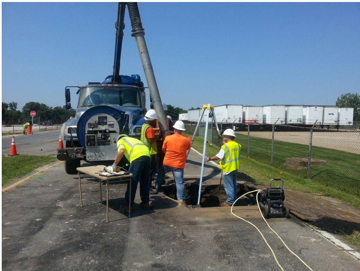
Vacuum truck removing water and residual sediment at catch basin IL-30A
