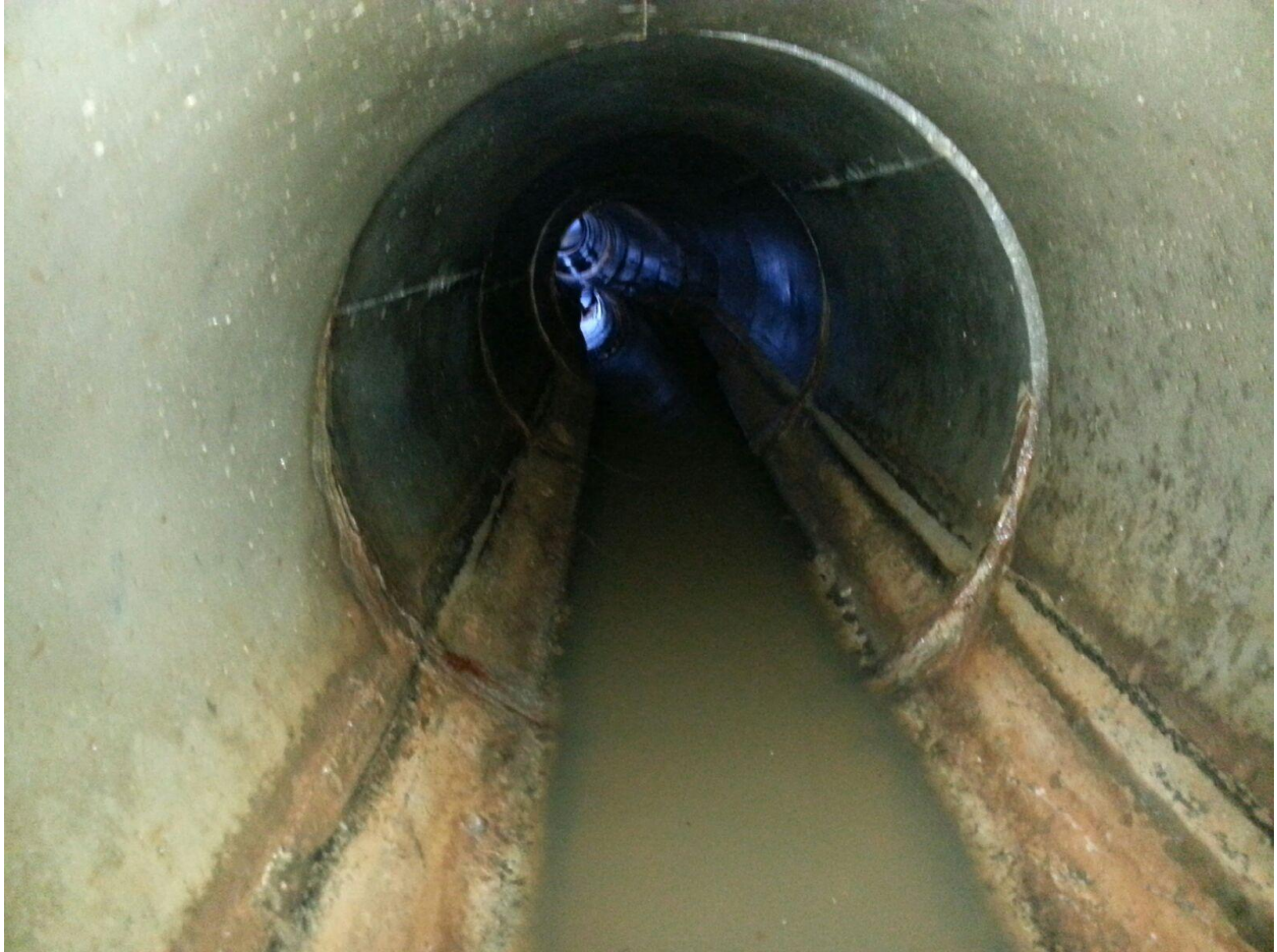
Post-cleaning condition of pipe looking downstream from IL-30A towards IL-30
