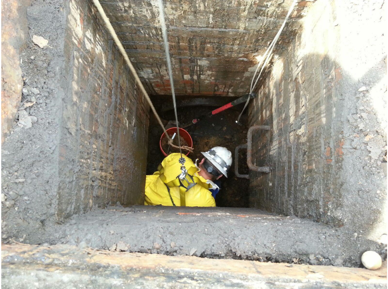
Removing sediment from IL-30A
