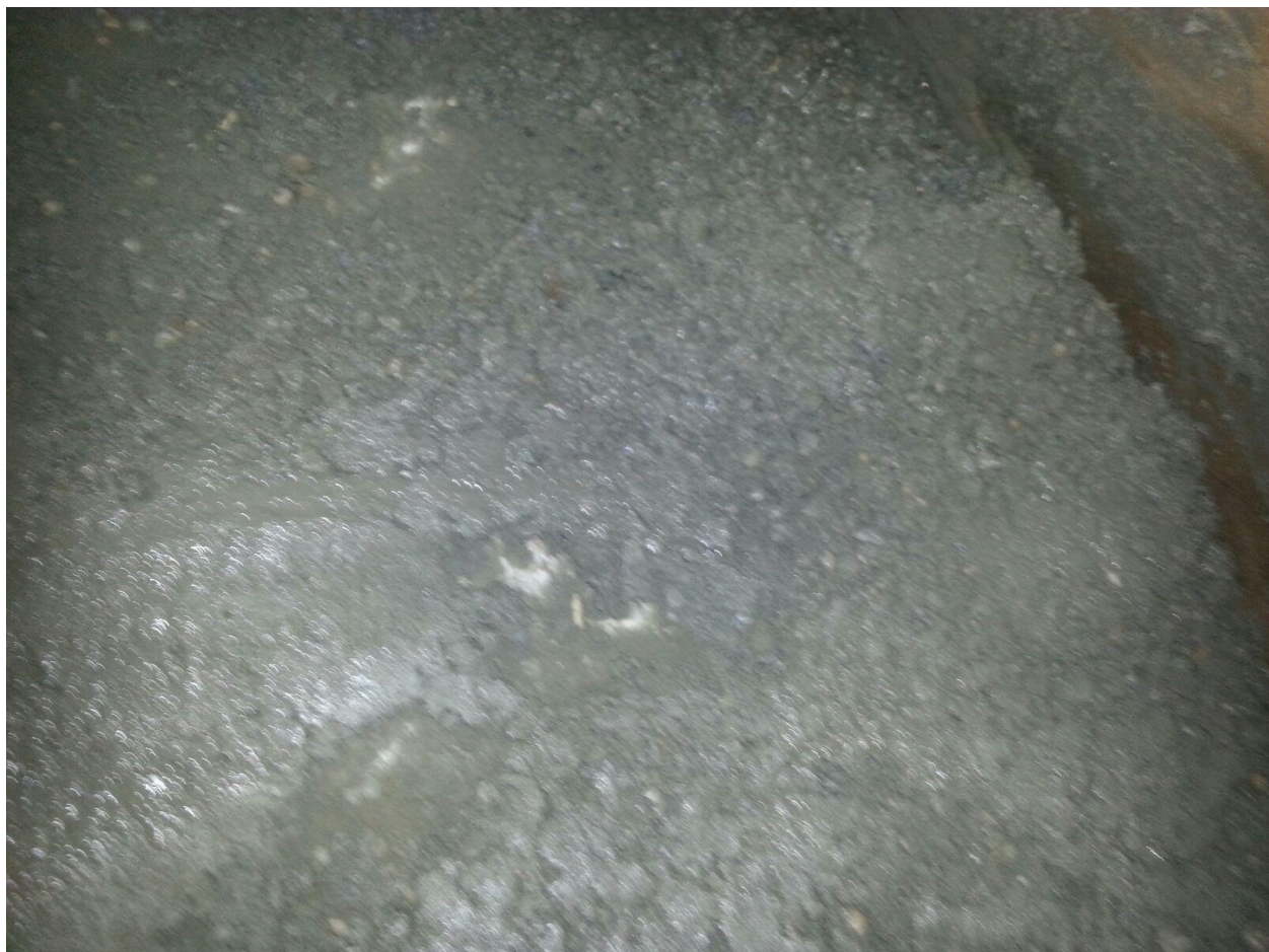
Concrete plug in IL-30A
