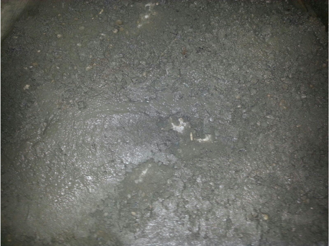
Concrete plug in IL-30A
