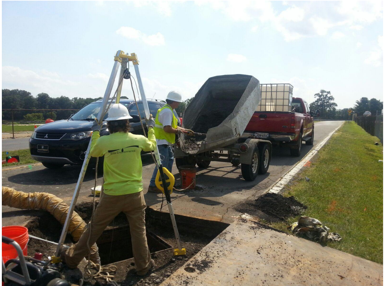
Adding concrete for plug at IL-30A
