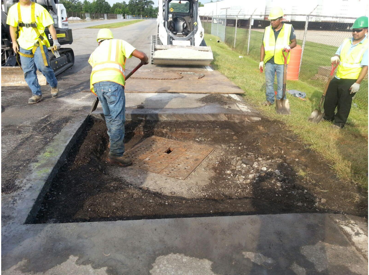
Site preparation for backfilling and paving
