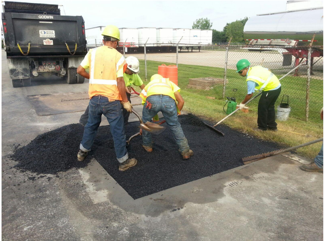
Application of first course of hot-mix asphalt (bituminous concrete)
