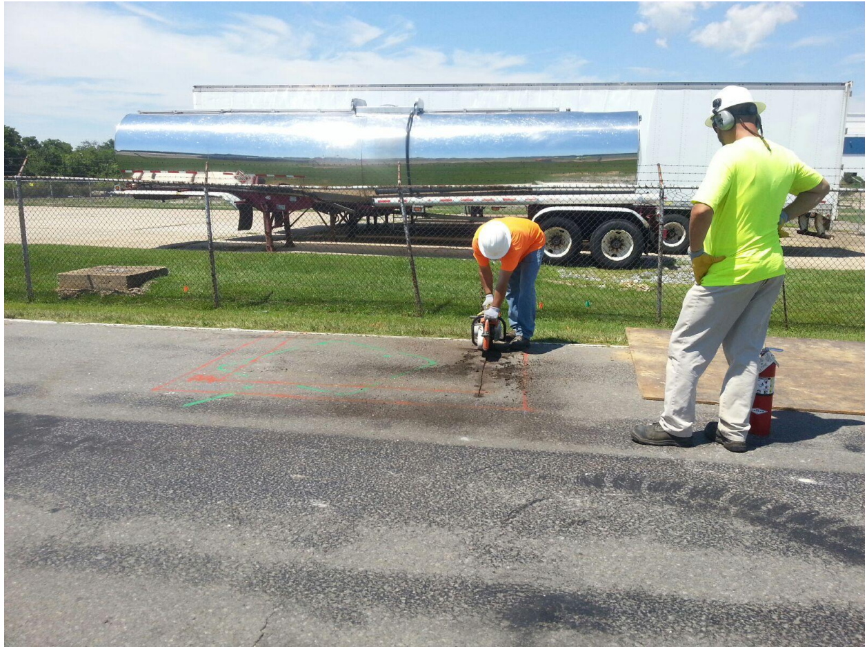
Saw cutting pavement to access storm drain catch basin IL-30A
