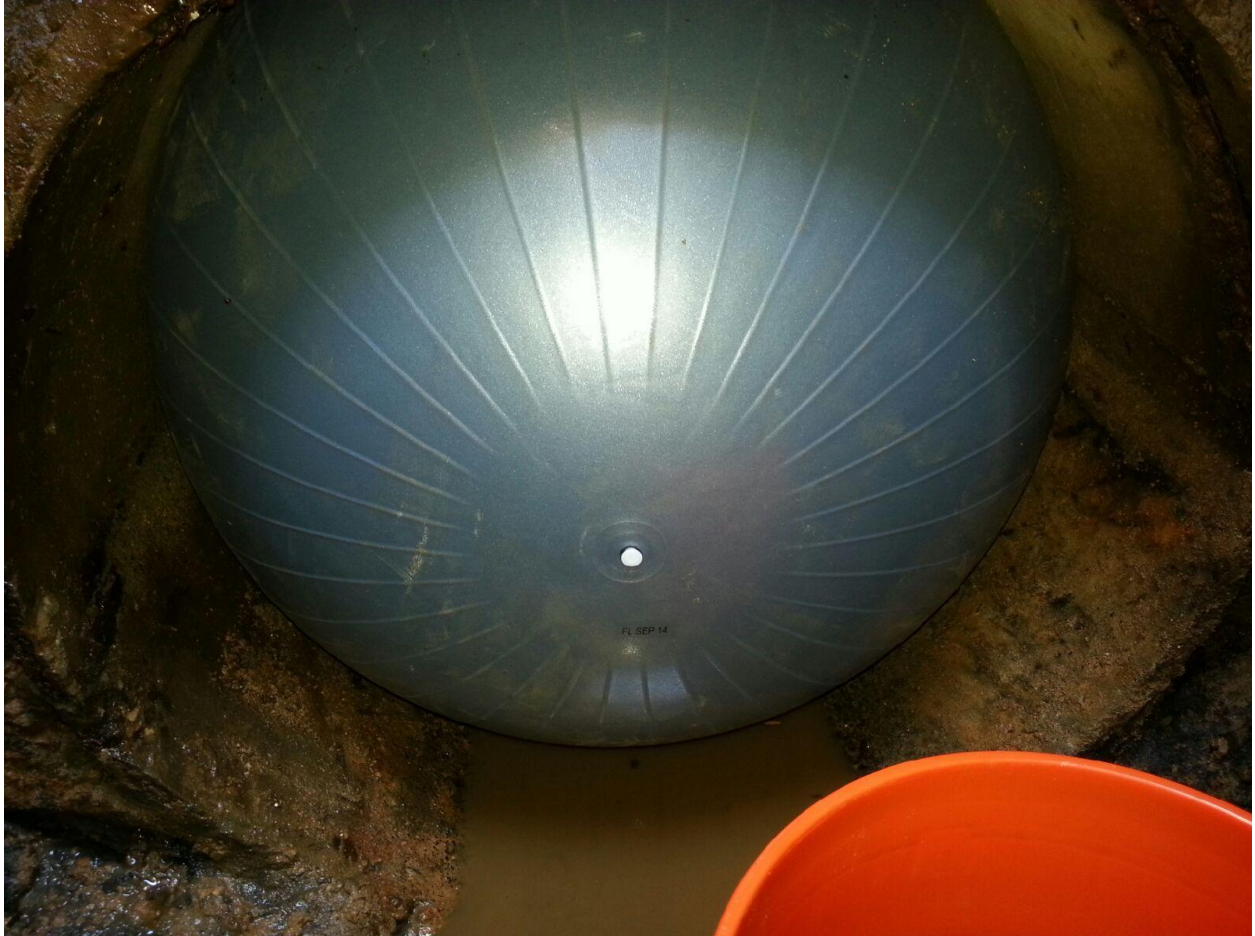
Temporary inflatable sewer plug installed in upstream pipe of IL-30A for cleaning.
