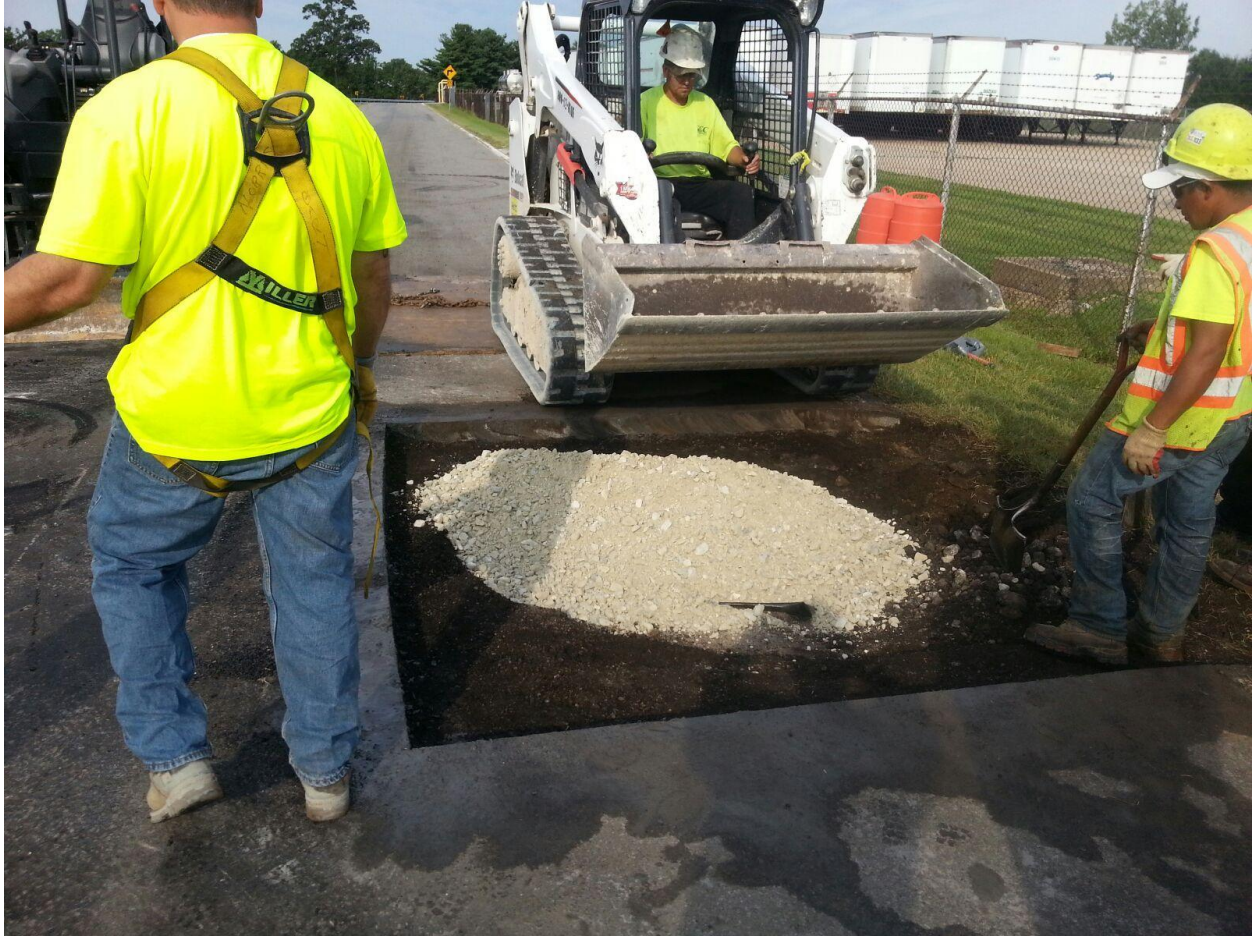
Placing graded aggregate base (CR-6) to level with existing sub-base
