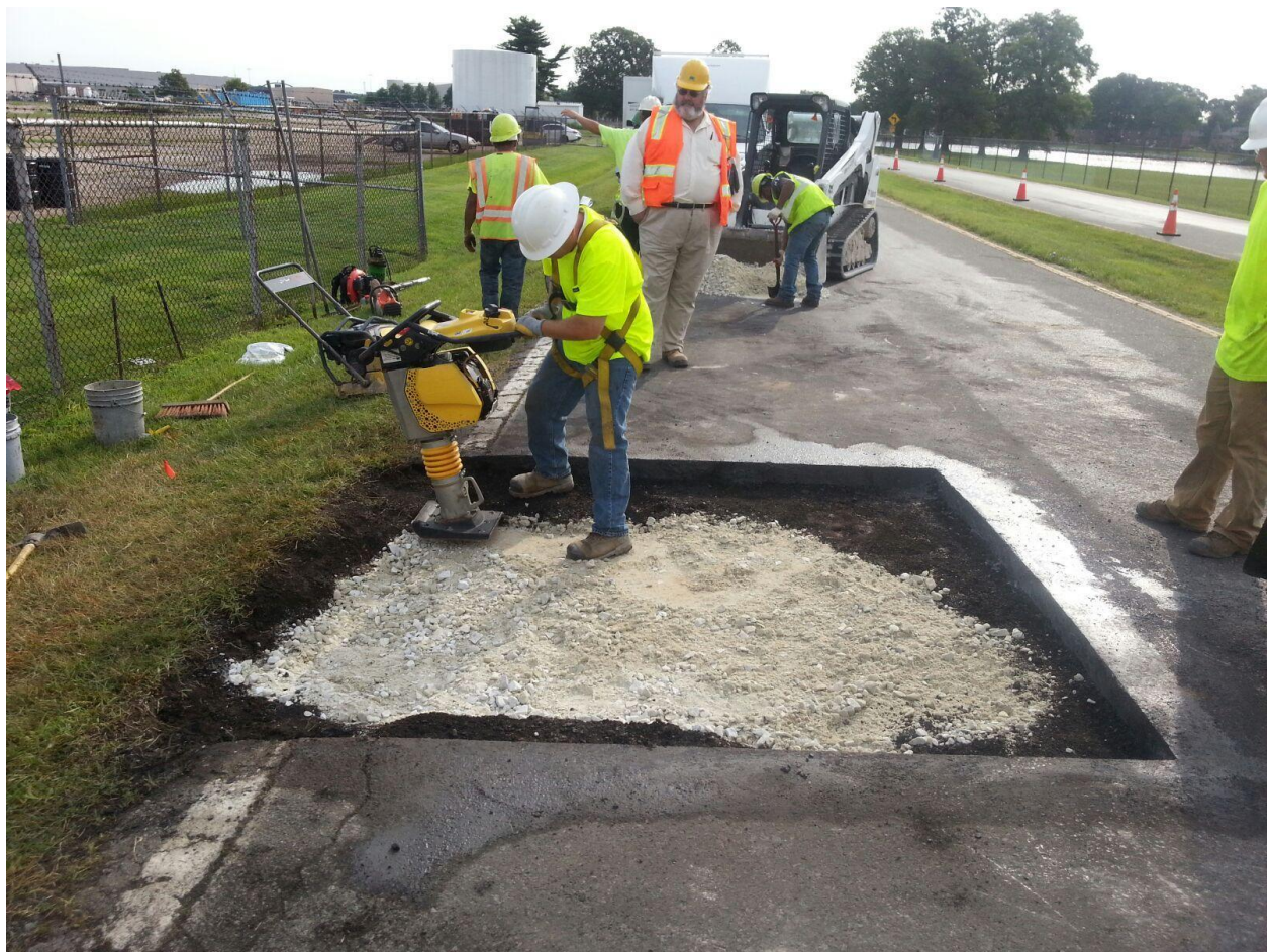
Mechanized tamping of CR-6 for compaction
