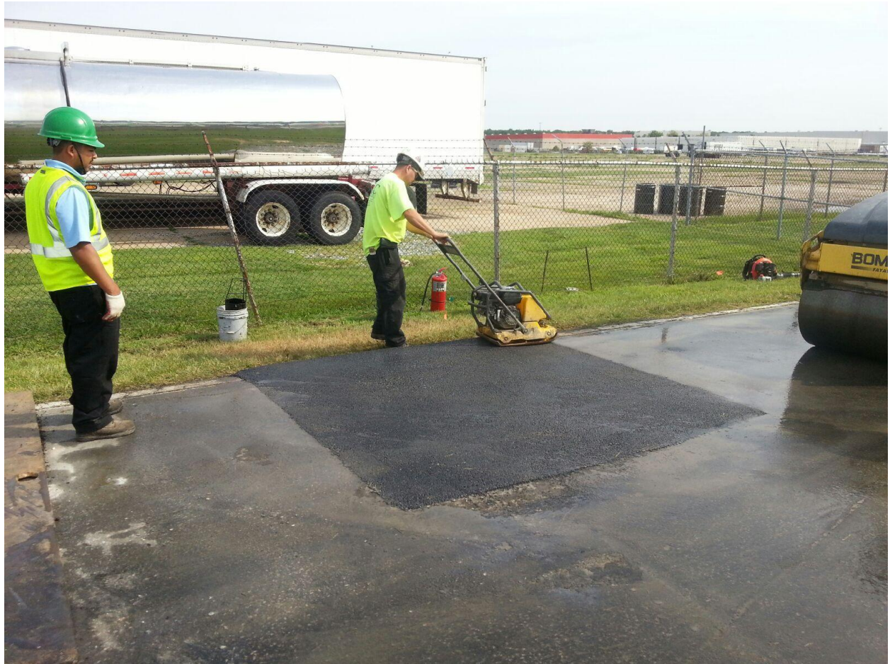
Mechanized tamping of surface pavement application. Subsequently rolled using mechanized drum roller shown in right side of photograph.
