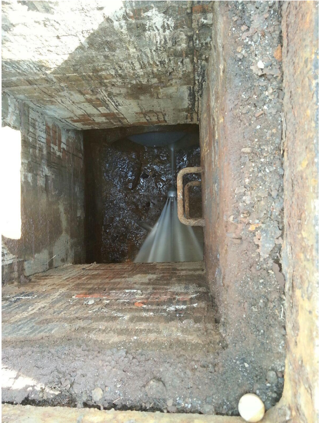
Looking down into interior of IL-30A with activated high pressure hydraulic cleaning head
