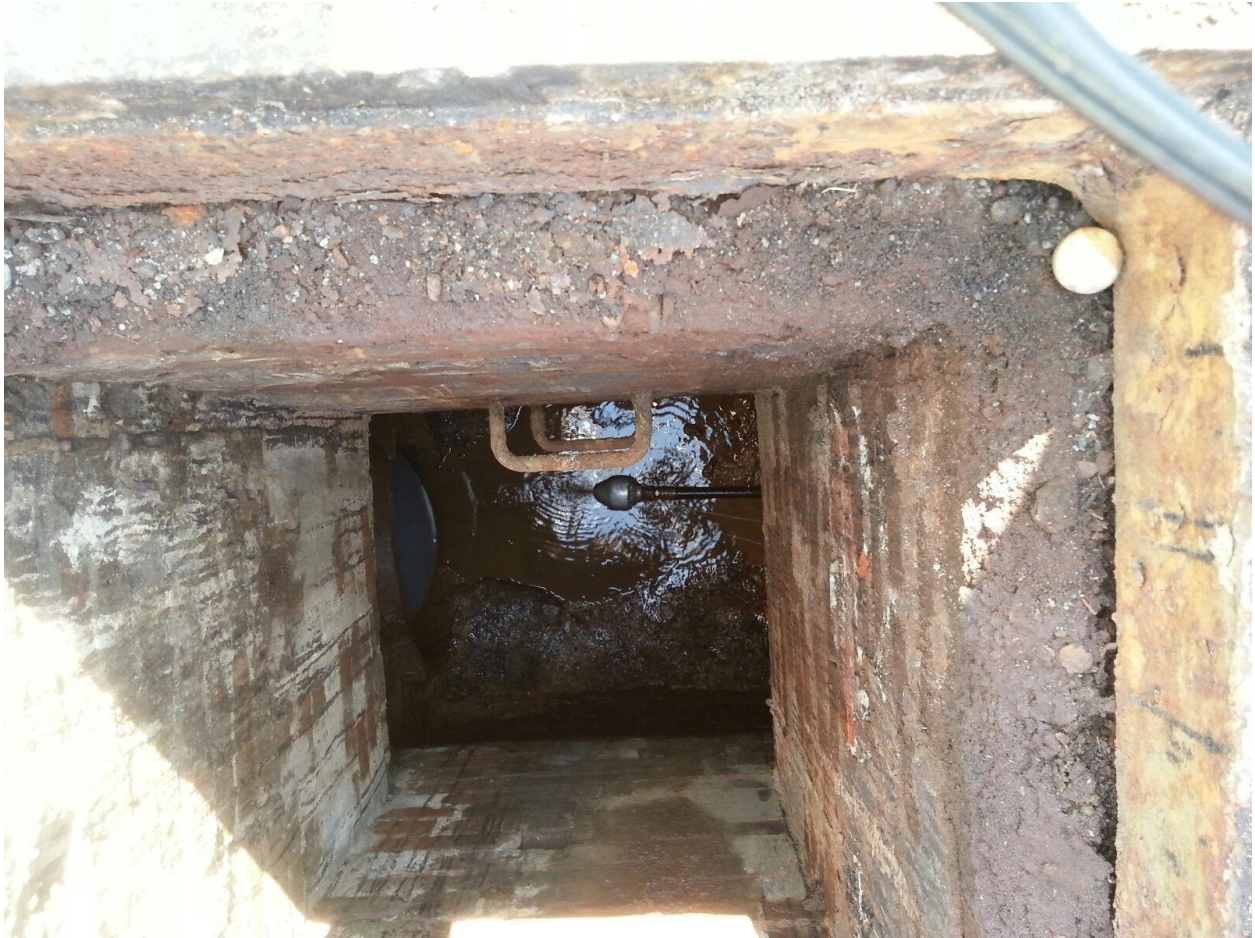
Looking down into interior of IL-30A with high-pressure hydraulic cleaning head (unactivated)
