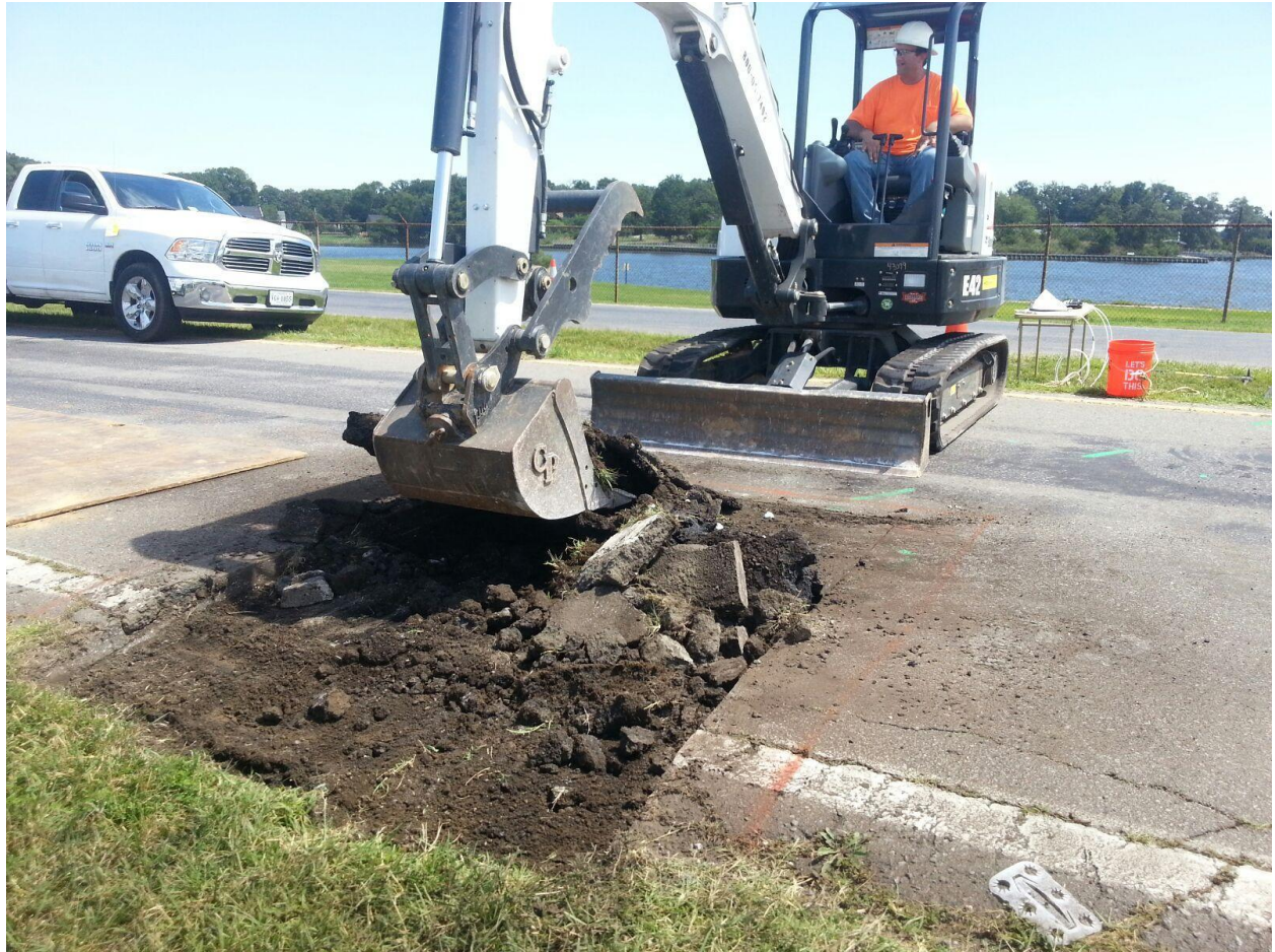
Removing pavement from location of IL-30A
