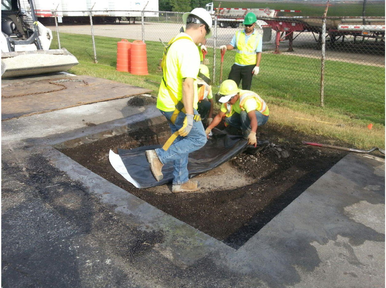
Geomembrane cover to prevent migration of graded aggregate base (CR-6) into storm drain
