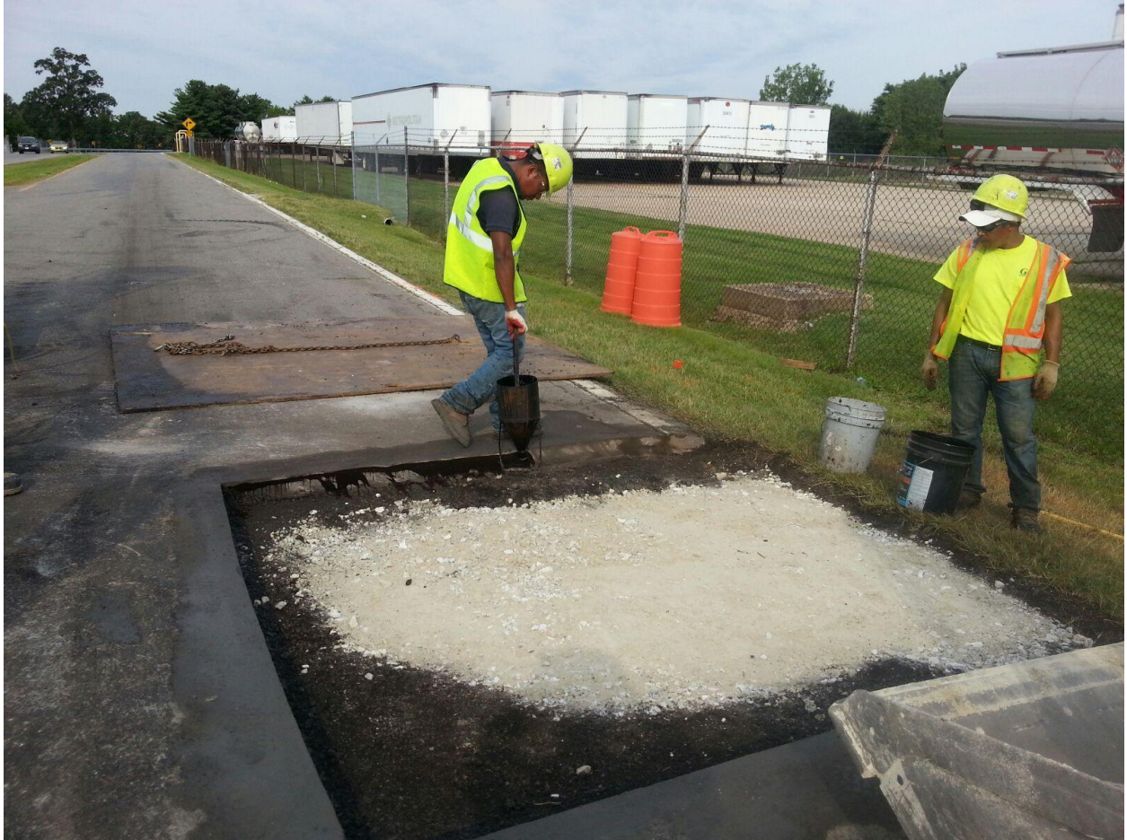
Application of tack seal along perimeter of bound pavement
