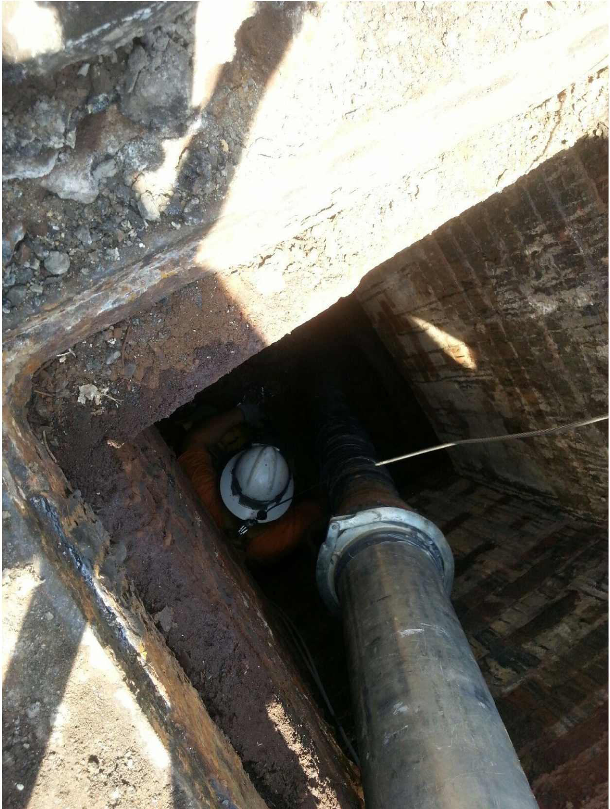
Vacuum truck removing water and residual sediment at catch basin IL-30A
