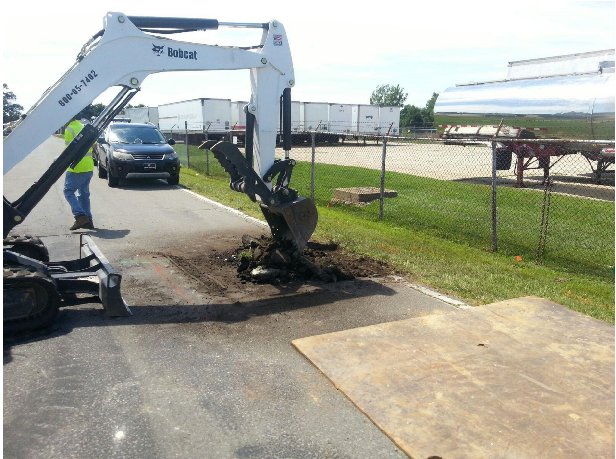
Removing pavement from location of IL-30A
