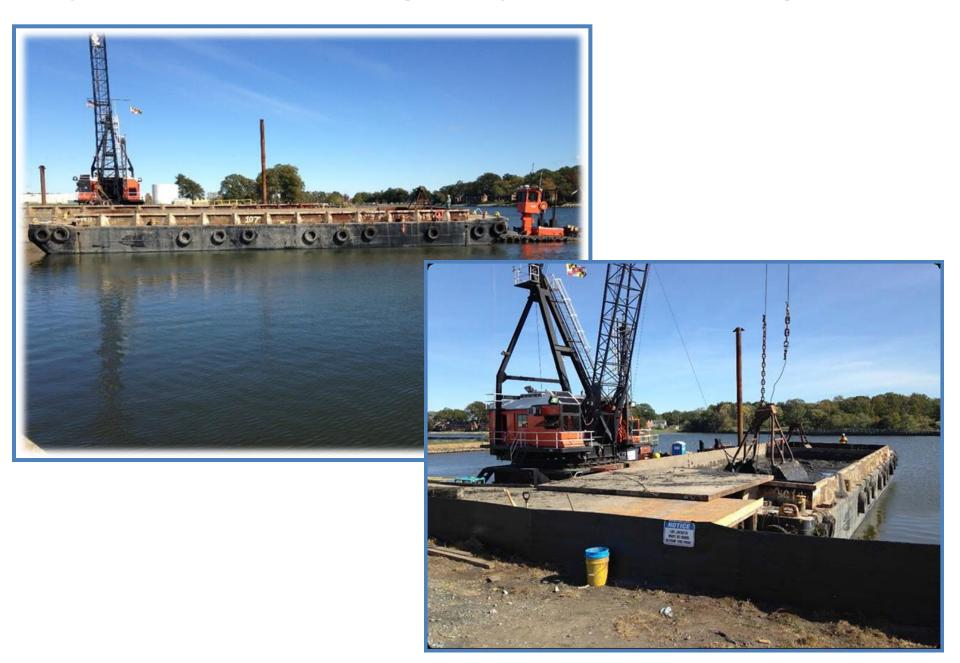
Using an apron to contain spillage, dredged sediments are offloaded from the barge. Haul trucks are positioned for sediment transfer at the spill apron.
