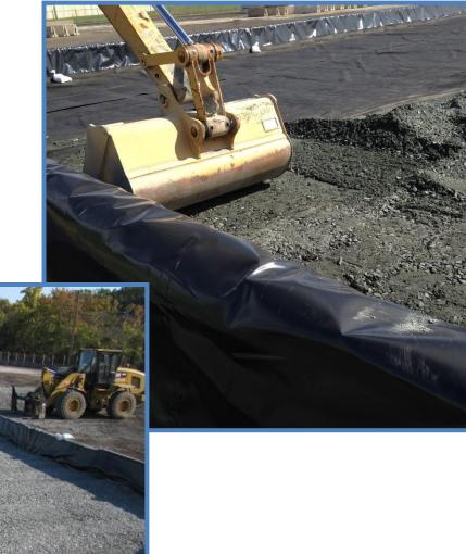
The construction area haul road is constructed of protective plastic sheeting covered by gravel. All of this will be removed at project completion.
