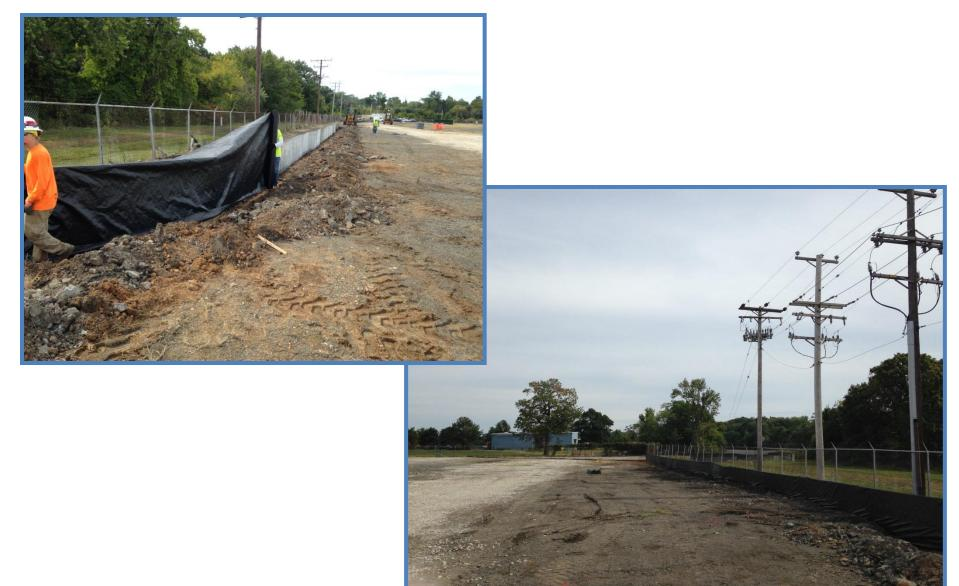
Other methods used to protect work areas included installing temporary asphalt berms, filter logs, and plastic sheeting anchored with rocks to protect rainwater outlets.
