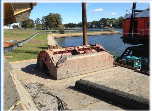
Sediment dredging began at the lower portion of Cow Pen Creek; sediments are loaded onto a barge, where sediments are stored, for transport to the offloading area.
