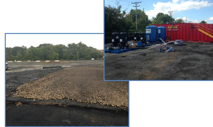
Sediment mixing bins were constructed using Jersey barriers and multiple layers of plastic sheeting.
