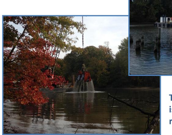
The environmental bucket is draining water but retaining sediment.
