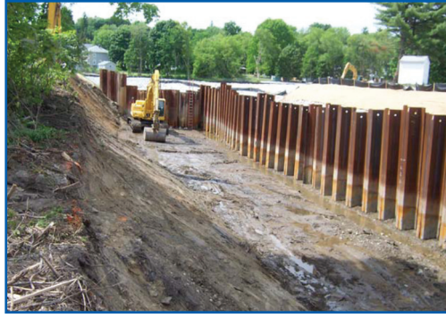
A temporary coffer dam also creates a dry work area.
