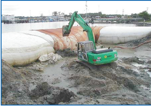
A temporary bladder dam creates a dry work area.
