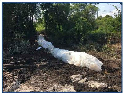
The lower part of the creek is wider, so the lower dam needed to be larger and was created by filling a bladder dam with water. Temporary barriers and fencing were installed to protect the community by preventing access to the
