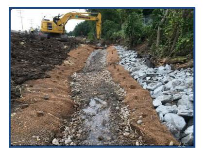
Final stream reconstruction included seeding; placing erosion matting and straw within the wetlands and floodplain areas; and conducting the final as-built survey.
