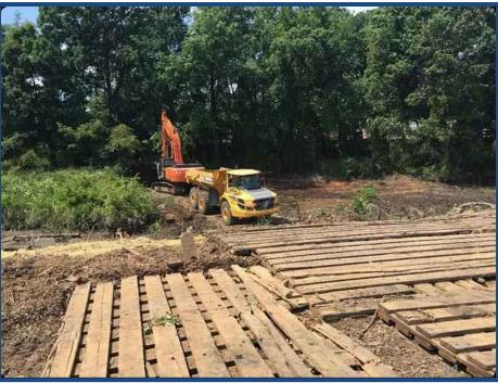
To determine whether excavation was complete, surveys confirmed both the width and depth from which sediment was removed. Post-excavation samples were then sent for laboratory analysis to confirm whether cleanup goals were achieved; several locations required additional excavation to
