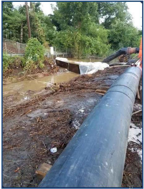
Heavy rains occurred again on Aug. 15, 18 and 21. The repaired dams held, so flood water had to be pumped out of the first excavation segment, sent to the treatment system, then discharged to the creek.
