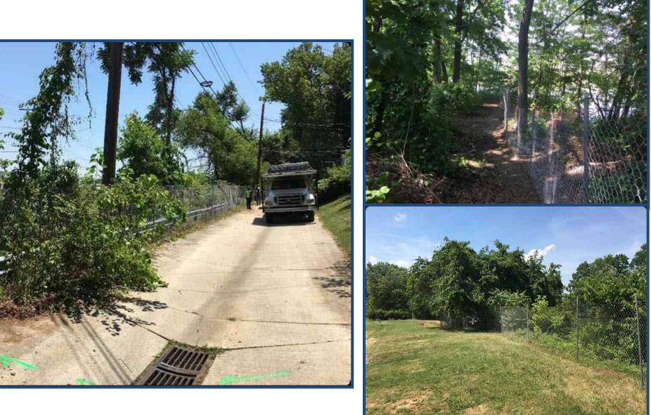
Before excavation began, vegetation was cleared along the east side of Cow Pen Creek to create access for large equipment. Trees and mulch were stockpiled for reuse during creek restoration.
