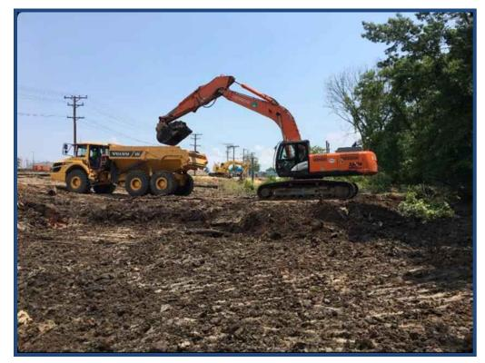
Loaded trucks hauled excavated sediment upland to handling bins, where sediment was mixed with drying agents and placed in loading trucks for offsite disposal at licensed landfills.
