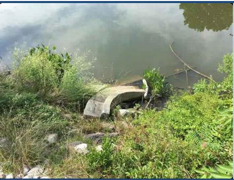
Before work began in the creek, water was drawn down within the individual excavation segment, and fish were collected, counted, identified and placed in the creek below the dammed-off work area.
