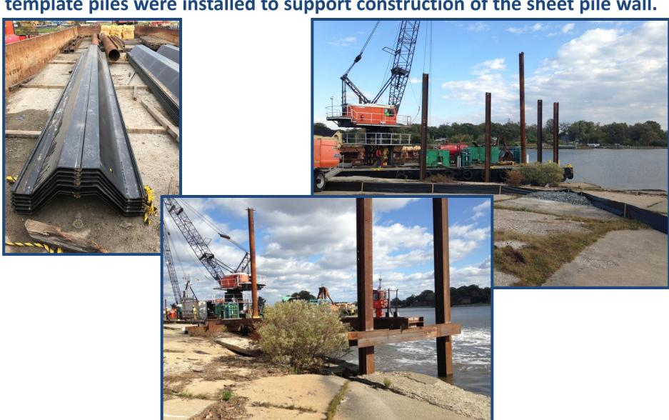
A crane positioned the sheet piles, and a vibrating hammer drove them to the planned depth.
