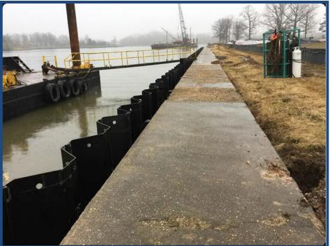
Spaces between the new sheet pile and the old bulk head were filled with gravel.
