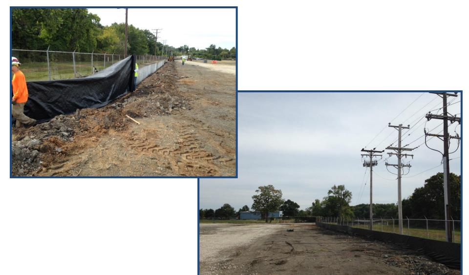
Other methods used to protect work areas included installing temporary asphalt berms, filter logs, and plastic sheeting anchored with rocks to protect rainwater outlets.
