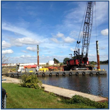
Dredging equipment arrived, then barges and cranes. A silt curtain was installed across the width of Dark Head Cove.
