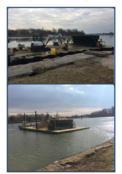
The hoppers were filled with sand using conveyors and barged to dredged areas for placement.
