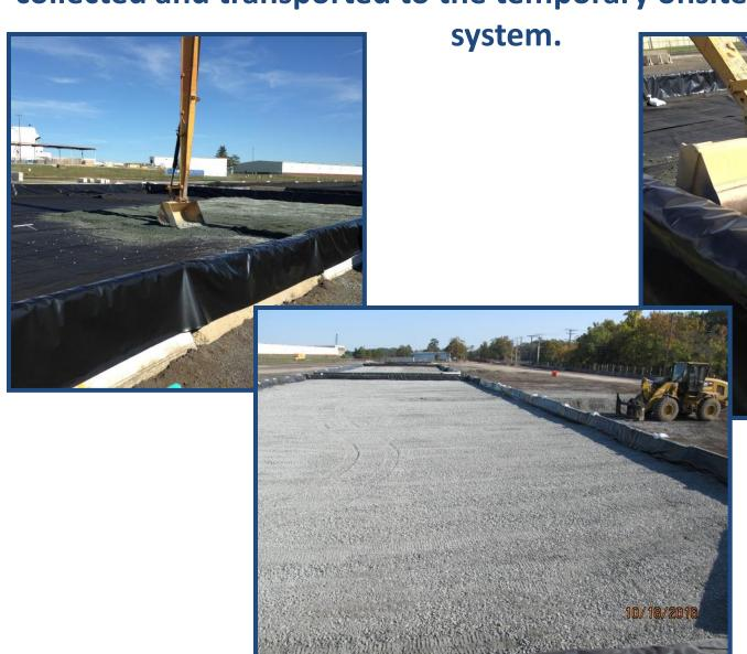
A temporary haul road was built with protective plastic sheeting and covered by gravel.
