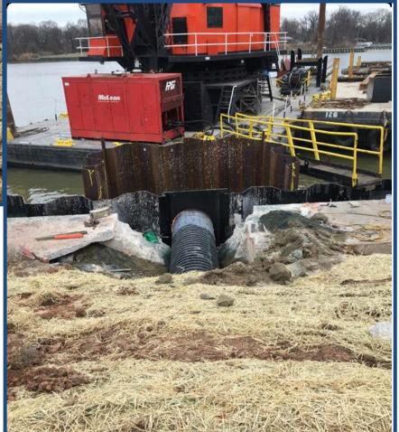
In Tax Block D, the area closest to Martin State Airport, a large double-piped outfall (009) was repaired.
