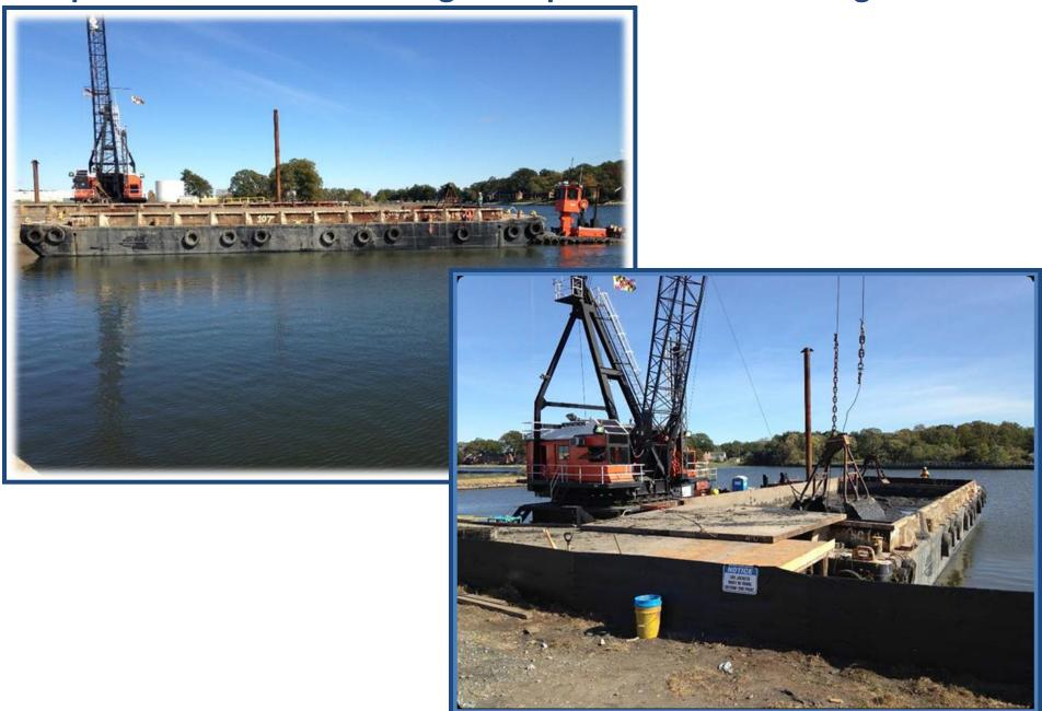
Using an apron to contain spillage, dredged sediments were offloaded from the barge. Haul trucks were positioned for sediment transfer at the spill apron.
