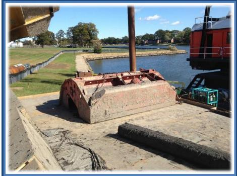
Sediment dredging began at the lower portion of Cow Pen Creek. The material was loaded onto a barge for storage, then transported to the offloading area.
