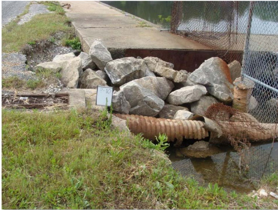
Photo 30. DHC Station 25+00, looking southeast at Outfall 07 (48 inch corrugated metal pipe).
