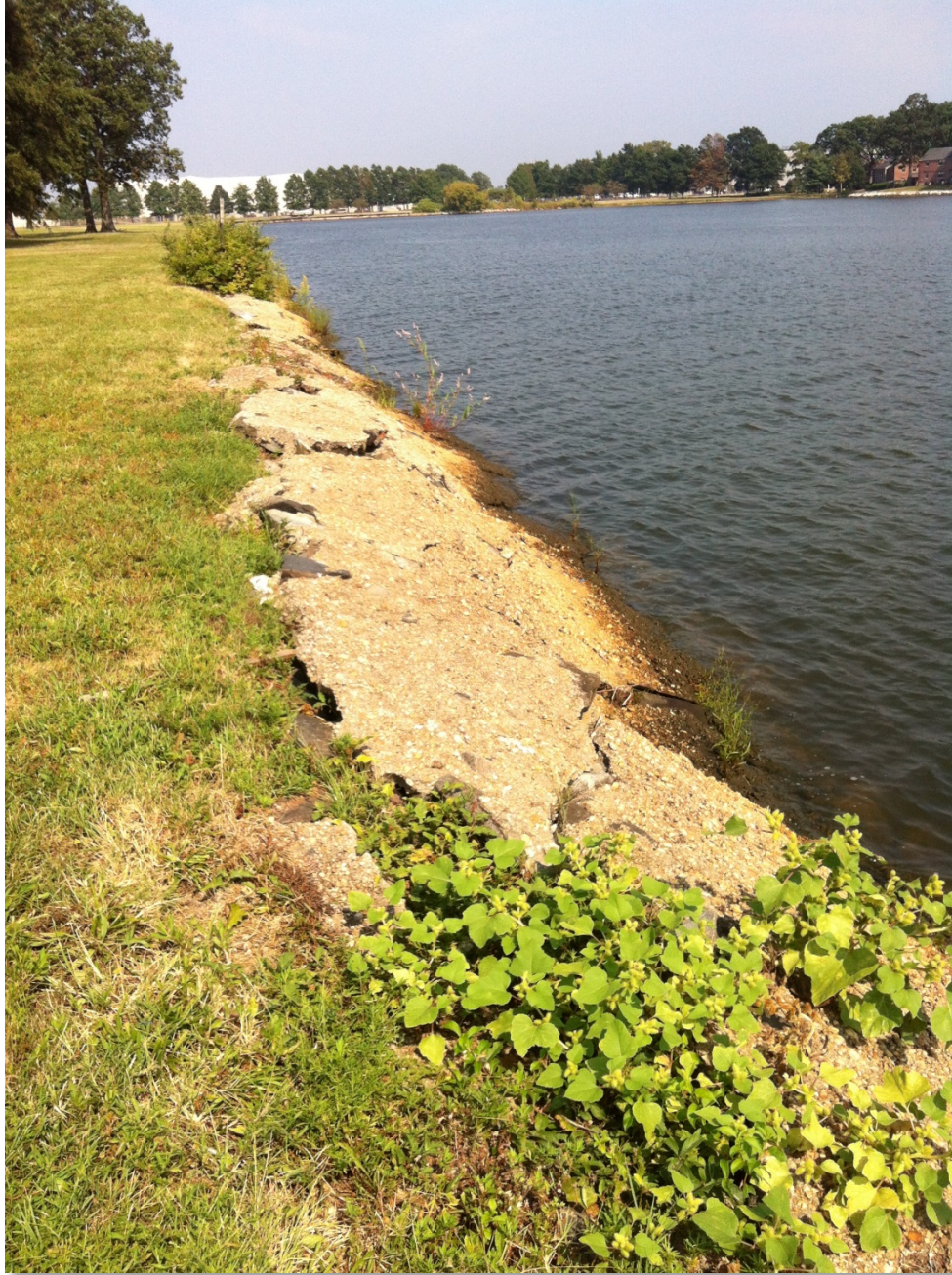
Photo 24. DHC Station 13+00, looking northeast along riprap with concrete overlay.
