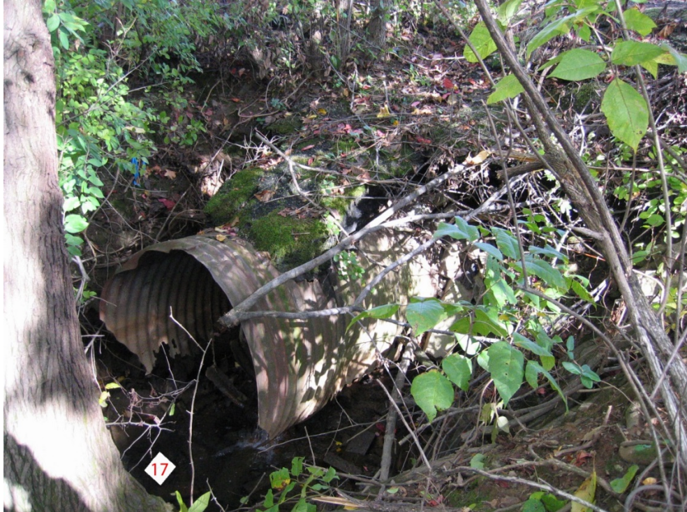
Photo 12. CPC Station 18+65, Outfall 004 (42 inch corrugated metal pipe).
