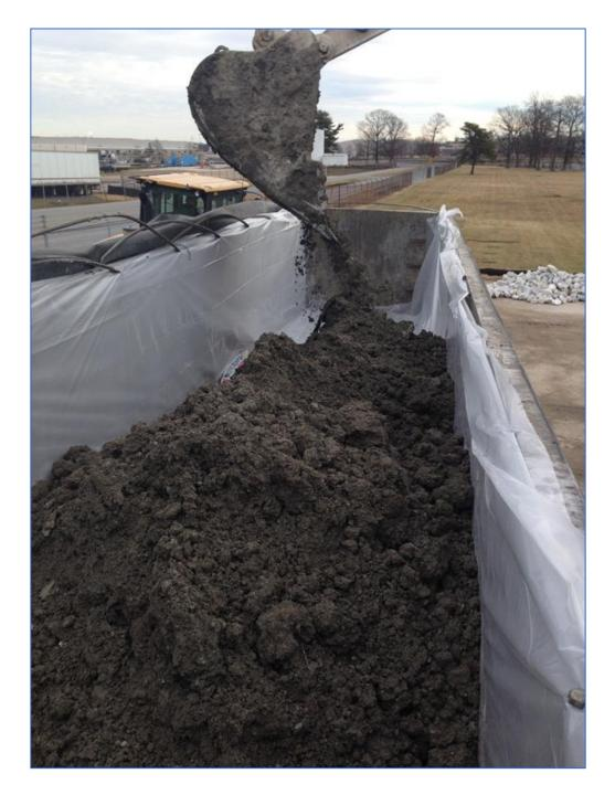
Trucks were weighed before leaving the site to haul sediment to the landfill. 9,928 tons, or 421 truckloads, were transported to the landfill as part of this project.
