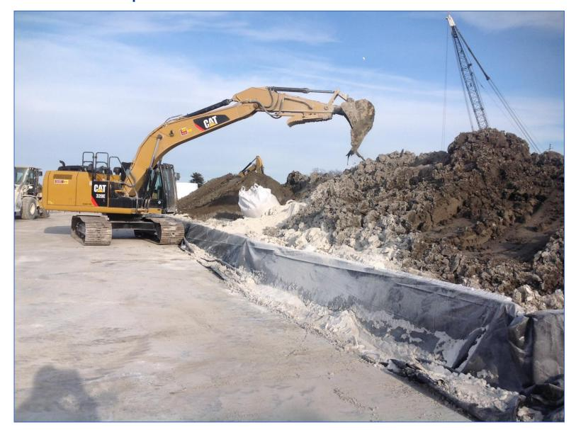
As the dredging equipment moved from area to area, the silt curtains were moved to continue surrounding work zones. Icing within the work area was managed by dredge equipment movement.
