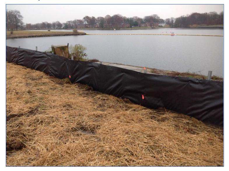
Monitoring was performed before work began to establish what the turbidity level was during "normal" conditions. After work began, the turbidity levels were monitored regularly both inside and outside the work area. This was done to assess what effects the dredge operations might create, and to confirm that water quality requirements were met.
