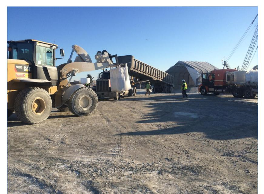
Sediment was mixed with Calciment and Quicklime in the dewatering pad. These additives reduced the moisture, and provided strength and body to the sediment, allowing it to be safely transported and properly disposed in a licensed landfill.
