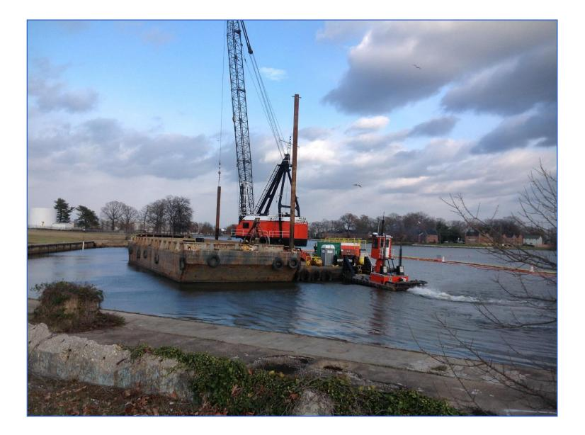
A silt curtain (interior) was placed near the dredge equipment to restrict movement of sediments during the dredging; a second, exterior curtain further restricted silt from leaving the work area; as needed, a third, interior curtain was used.
