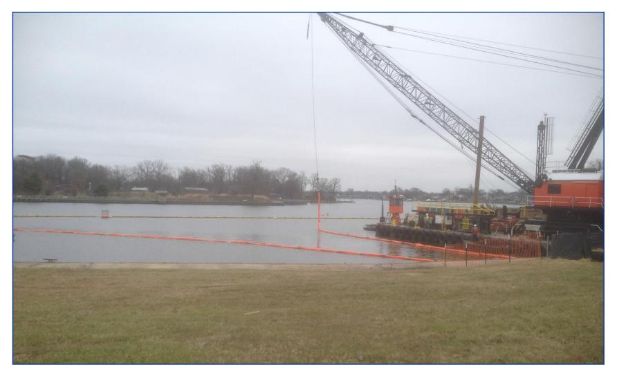
A lined spill apron was installed to capture any spillage of sediments that might occur when sediments were moved from the dredge barge to dump trucks, which then carried the sediments to the dewatering pads. Spillage and eventually the liner were properly disposed in a permitted
