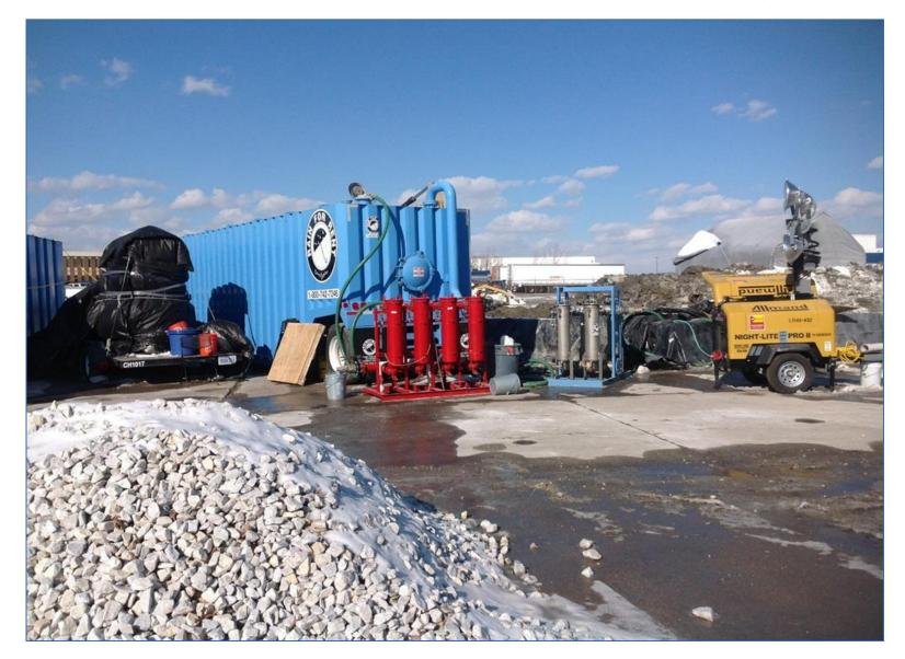
After confirming that treated water met all required criteria, it was pumped from holding tanks into a transport truck, to pump to the sanitary sewer system, which was allowed by permit.
