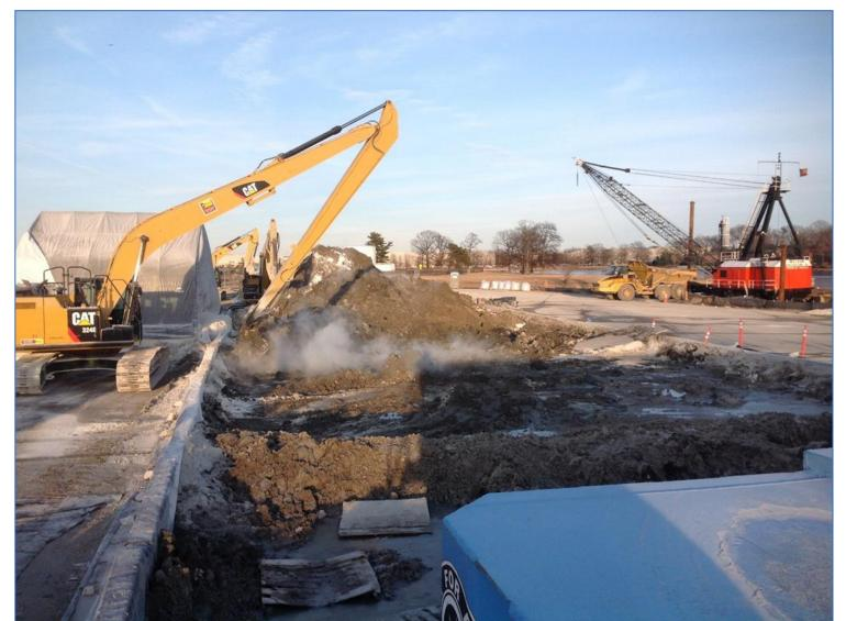
Portland cement amendment, loaded in a super sack, was added to provide strength and body to the sediment in preparation for proper landfill disposal.
