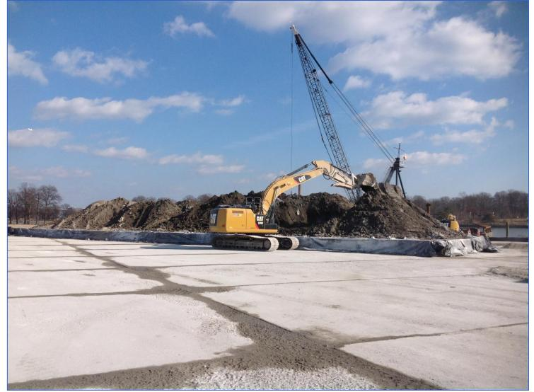
When sediment met landfill disposal criteria, it was loaded into lined dump trucks and covered for transportation.
