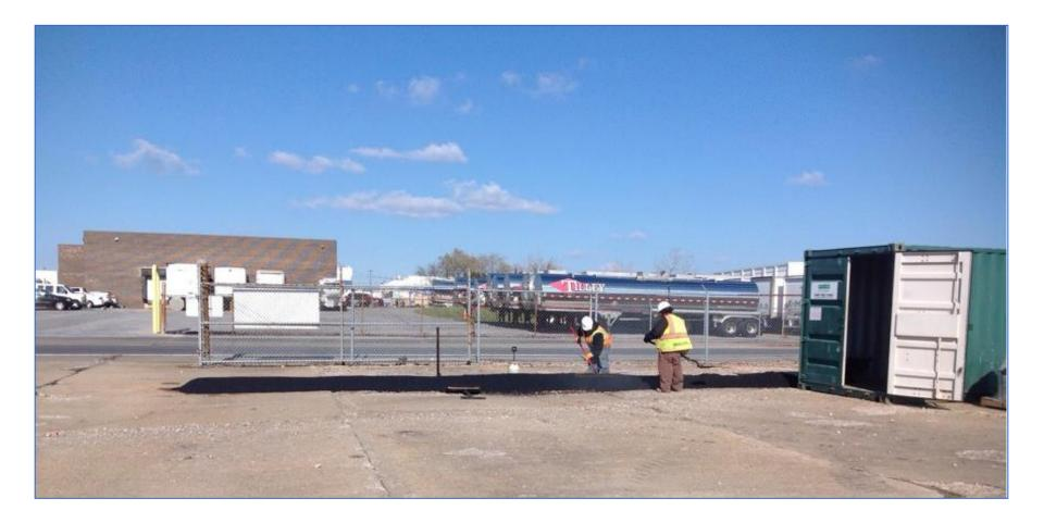
Reinforced super silt fence separated upland work areas and cove, preventing erosion and maintaining sediments upland.
