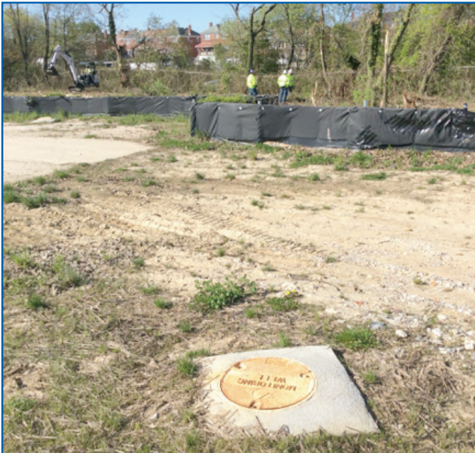
Erosion and sediment control fencing was erected around all work areas.
