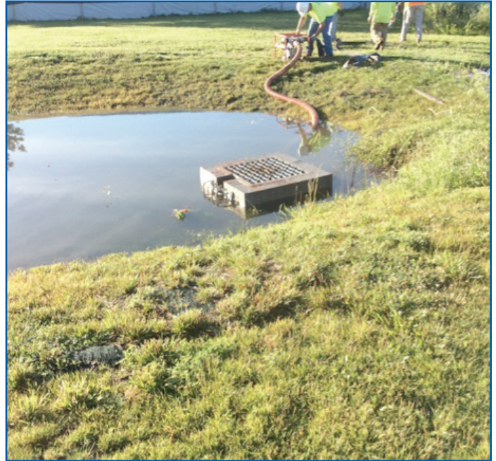
Stormwater was pumped from a swale.
