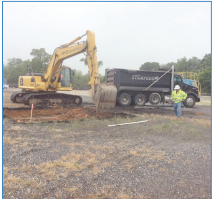
Soil excavations were typically about two-feet deep.
