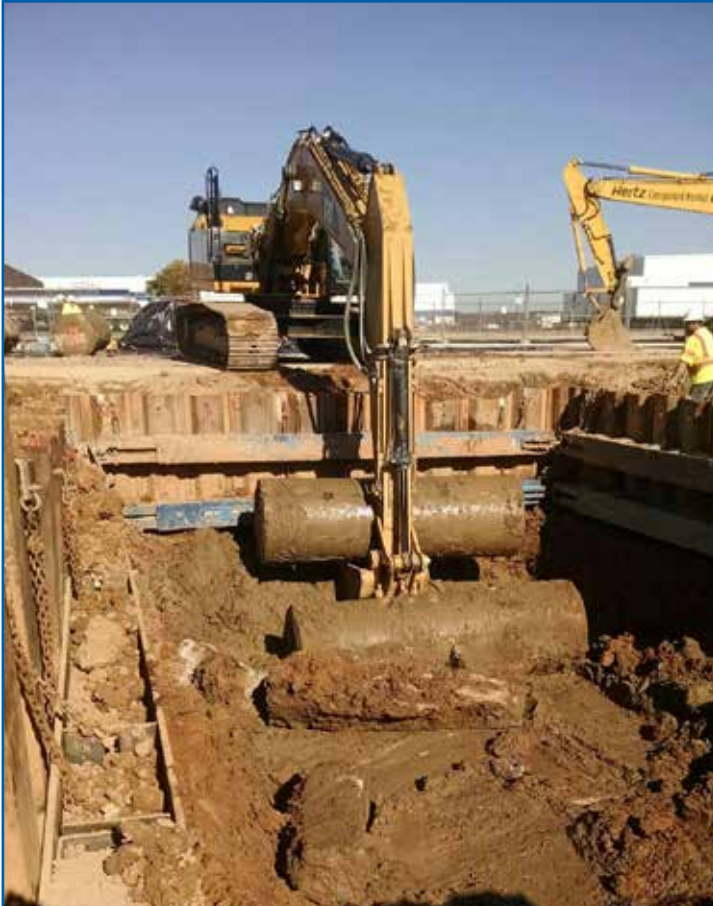
Seven underground storage tanks were removed in Block F.
