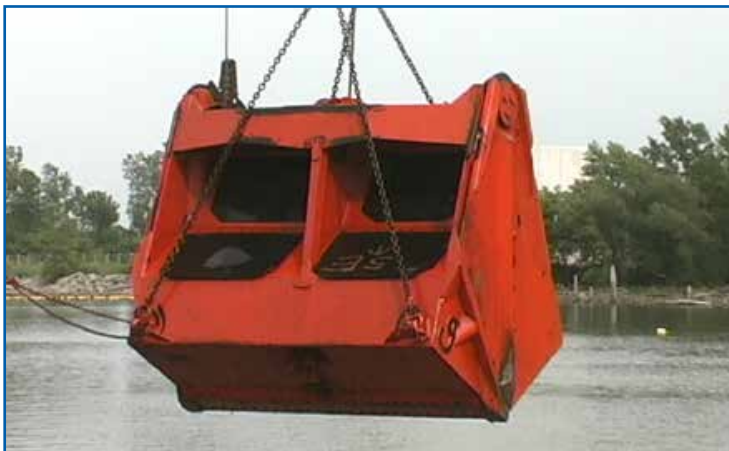
Clamshell bucket dredging.
