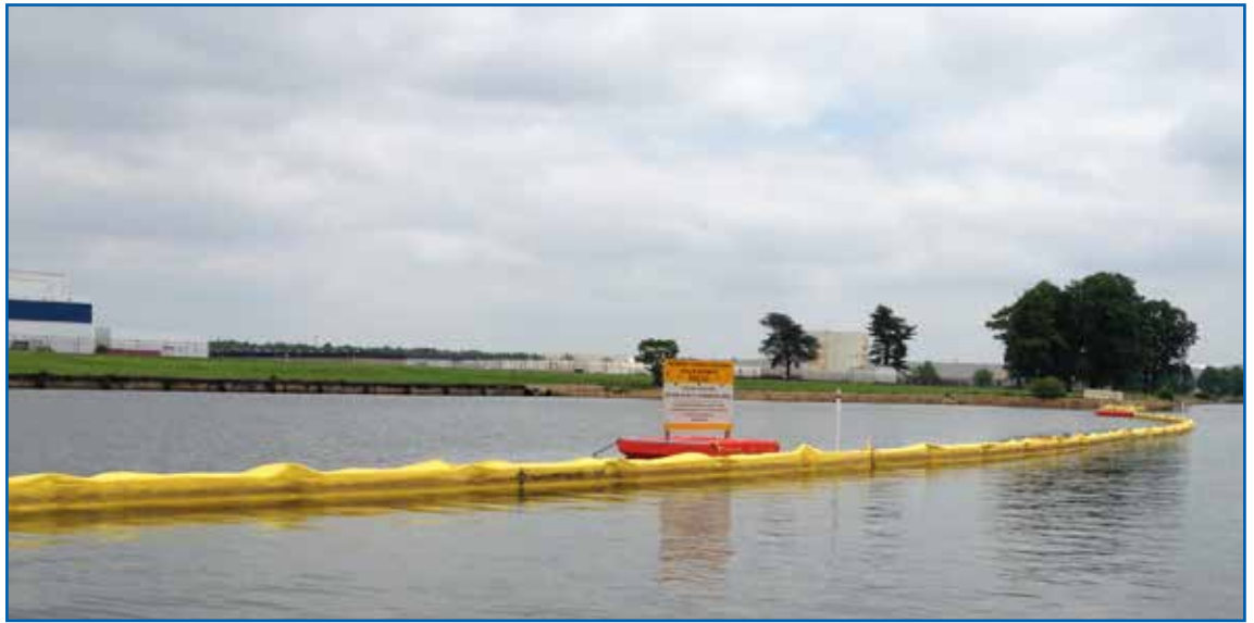
Boom line and silt curtain including informational sign installed.
