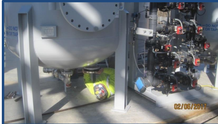
Liquid Phase Granular Activated Carbon Treatment Units
