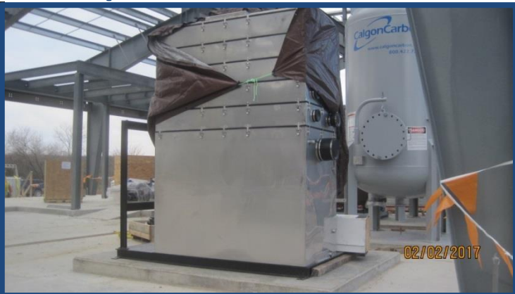
Air Stripper and Liquid Phase Carbon Unit
