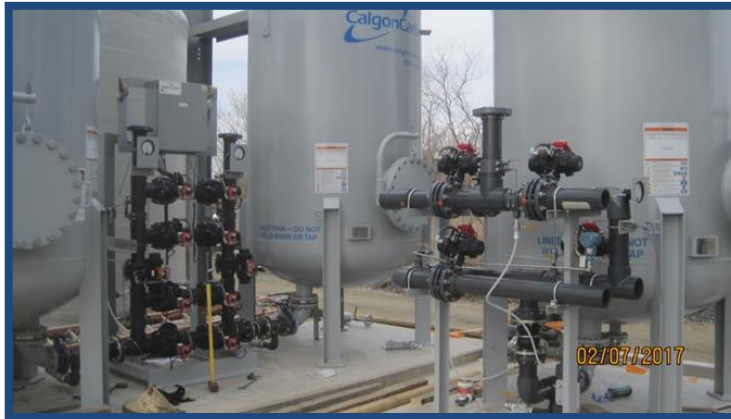
Air Stripper and Liquid Phase Carbon Unit
